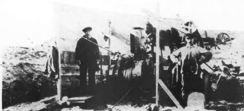
Power Hoist in Operation. It Is the Big Factor in Cutting Loading Costs at This Gravel Pit and Requires Little Attention.
