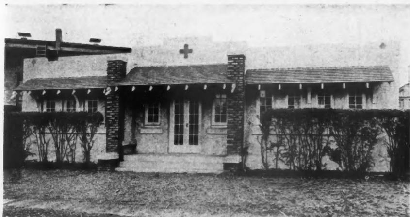
**Railroad Foreman's Office and Quarters Built by Standard System of Precast Concrete Units. A Stucco Finish Has Been Applied in the Same Way as in Any Class of Construction.**
