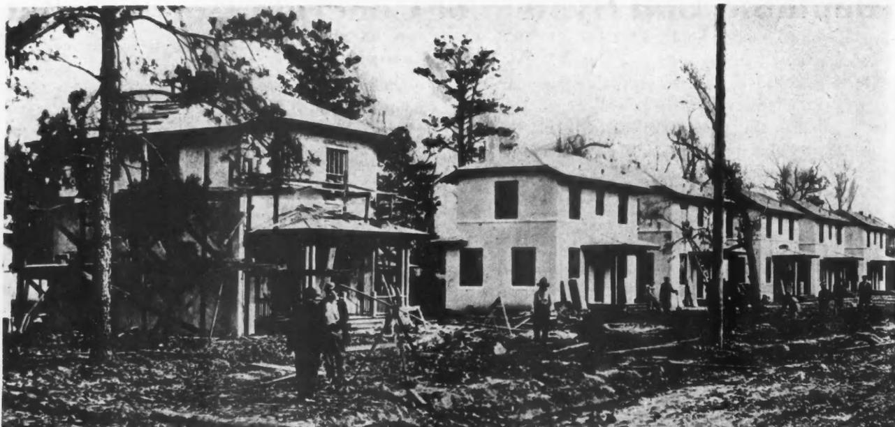
Industrial Housing Group at Baytown, Texas, Built of Precast System. The Units Were Cast on the Site of the Building. By Standardizing the Construction, the Baytown Refinery Co. Effected a Considerable Saving in Costs.
