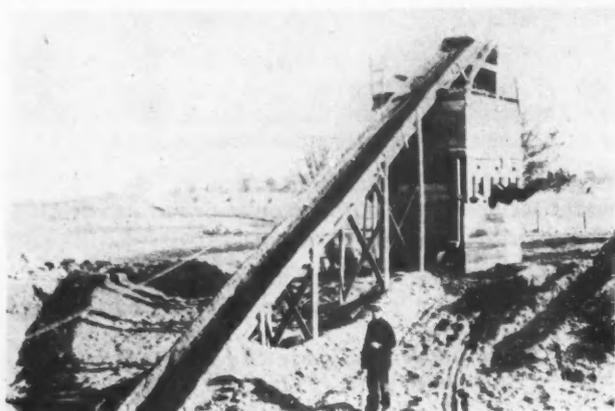
Chute Leading to Gravel Hopper. The Scoop Is Pulled Up by a Cable Operated by a Power Hoist. Trucks Can Drive Up to the Hopper and Be Filled in a Few Minutes.
