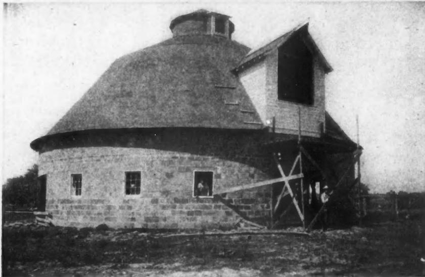
Completed Round Barn Built of Tile for W. S. French & Son in Southern Iowa by H. Mulvihill. The Barn Is 64 Feet in Diameter, the Silo 12 Feet.
