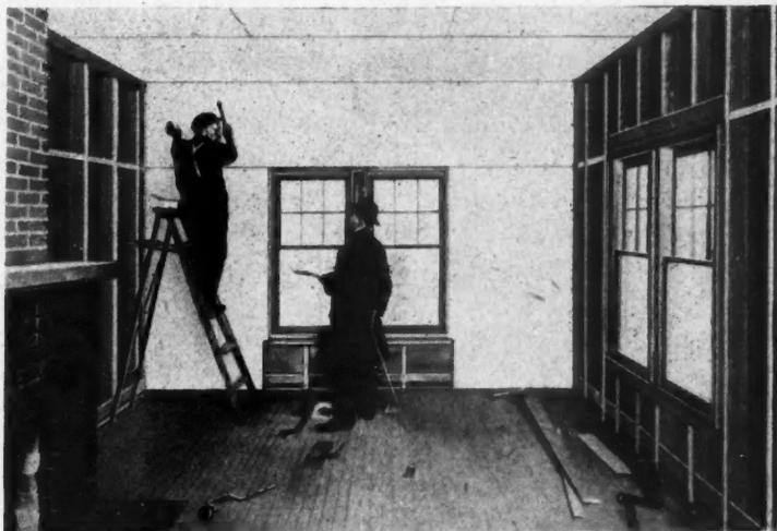
Fig. 2. Working Plan with Material List of Wallboard. Moulding Detail B with Material List. In the Small Picture the Carpenter Has Placed the Headers and is Now Applying the Wallboard. Compare Moulding Detail with Detail on Opposite Page.
