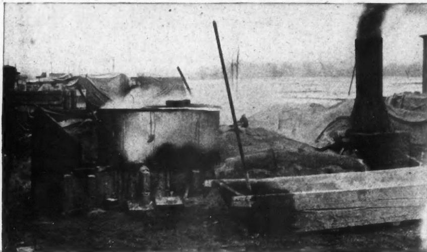
For Jobs of Moderate Size, Where a Steam Plant Is Not Available, Improvised Water and Aggregate Heaters Made of Old Tanks and Pipe Sections as Shown Above, May Well be Utilized for Cold Weather Concreting.
