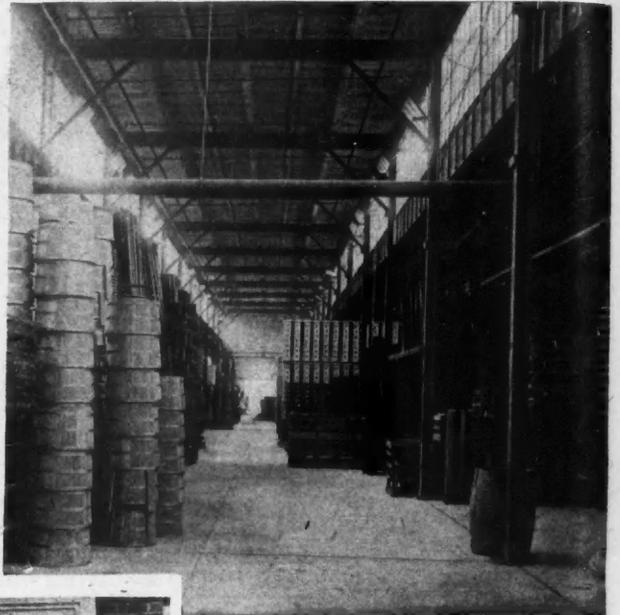
Warehouse of New Meadows Plant at Bloomington, Ill. It is 80 by 400 Feet. The Buildings Are of the Monitor Type with Brick Walls and Steel Sash.
