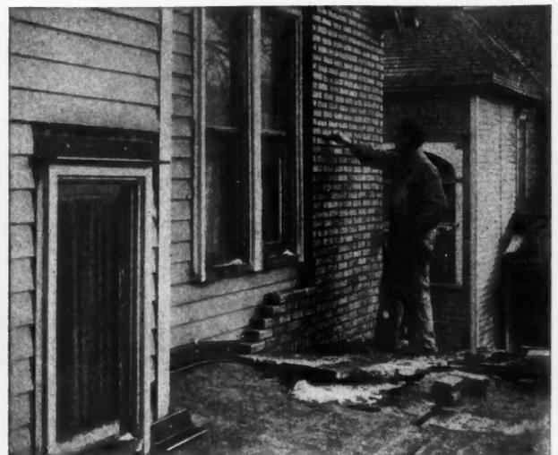
Veneering Above Kitchen Roof. Steel Angles Are Placed Against the Sheathing and Attached To the Studs So That No Weight of the Brickwork Comes on the Roof.
