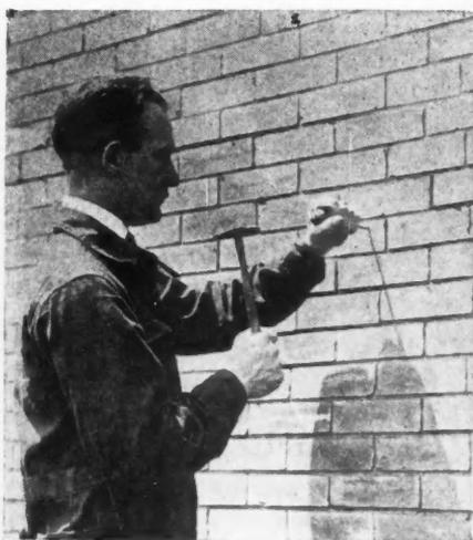
First Step—Drilling a Small Hole in the Brick Wall with Special Tool.
