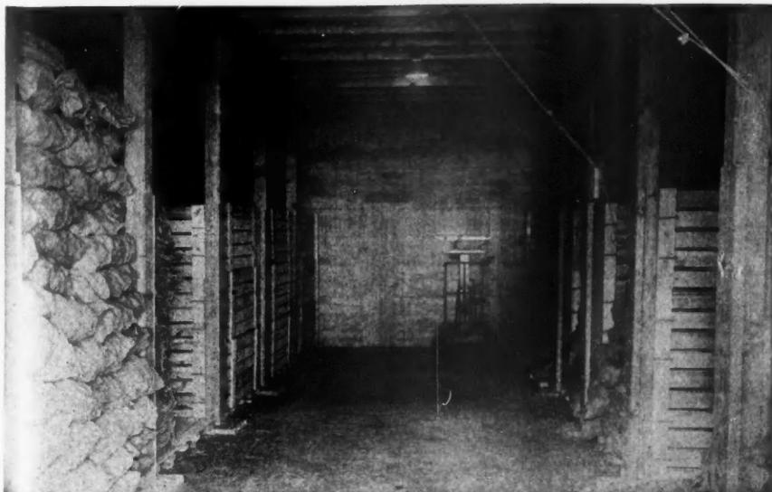
View of Cellar Inside. Note the Bins for Storing Potatoes and Other Vegetables. The Walls Are Double with the Space in Between Filled with Dry Earth. The Temperature During the Winter Was Constant at 39 Degrees.
