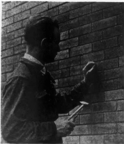
Second Step—Inserting Fibre Wall Plug in Hole. This Plug Is Made of Longitudinal Fibres Cemented Together.
