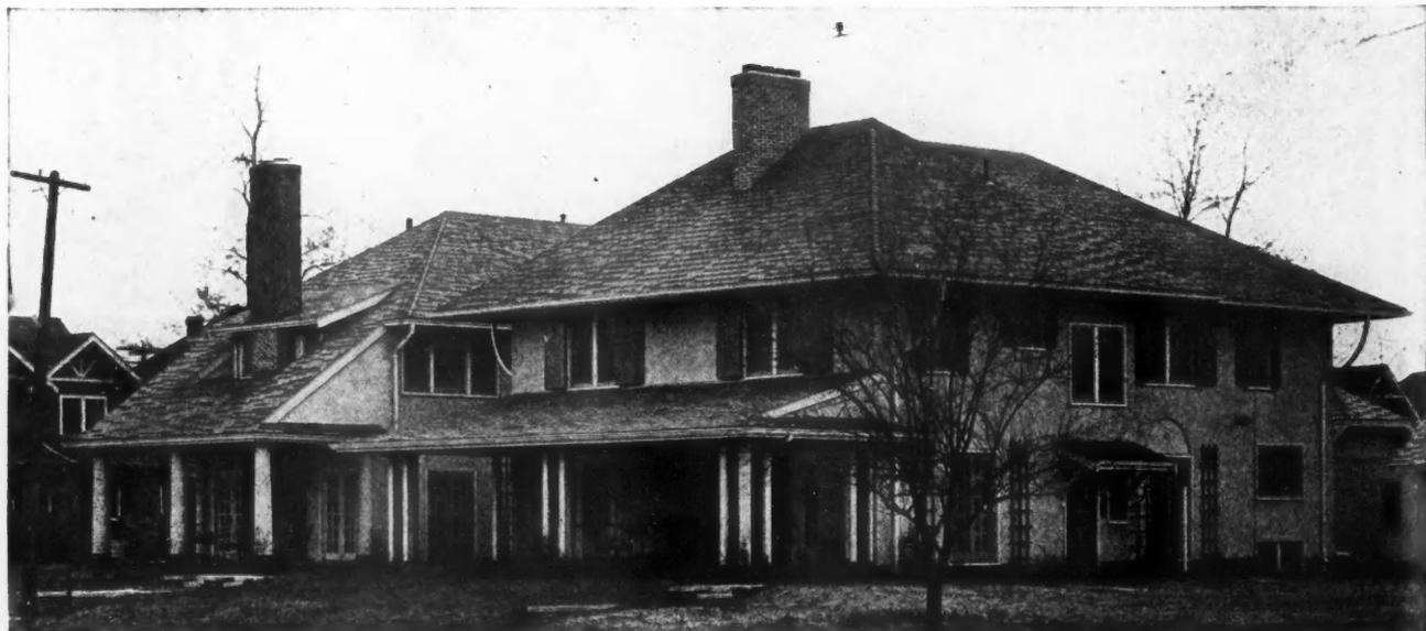
Fig. 1. Two Houses Covered with Asphalt Shingles. Notice How the Red and Green Shingles Have Been Placed on the House on the Right. This Mottled Effect Is Very Pleasing and Popular with Home Owners. This Roof Does Not Call for a Special Brand of Shingles.
