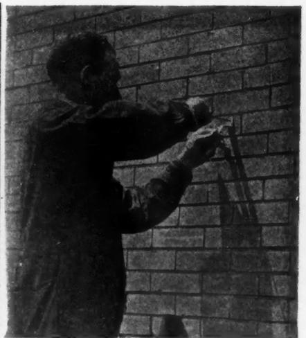
Final—Inserting Wood Screw Into Plug to Hold Fixture. The Plug Expands as the Screw Is Inserted, Gripping the Wall.
