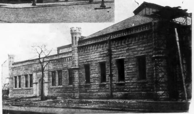
The Church Above Was Converted Into the Power House Below in About 30 Days. All of the Stone Was Hauled by Motor Truck a Distance of Six Miles.
