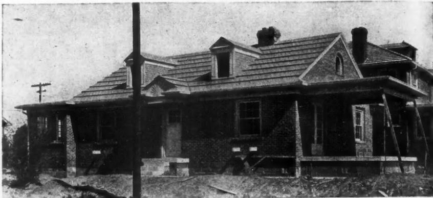
Fig. 2. Thatched Roof Effect with Composition Shingles. The Shingles Are Laid in Courses with Slight Elevations at Regular Intervals Made by Laying Two Layers of Bevel Siding.
