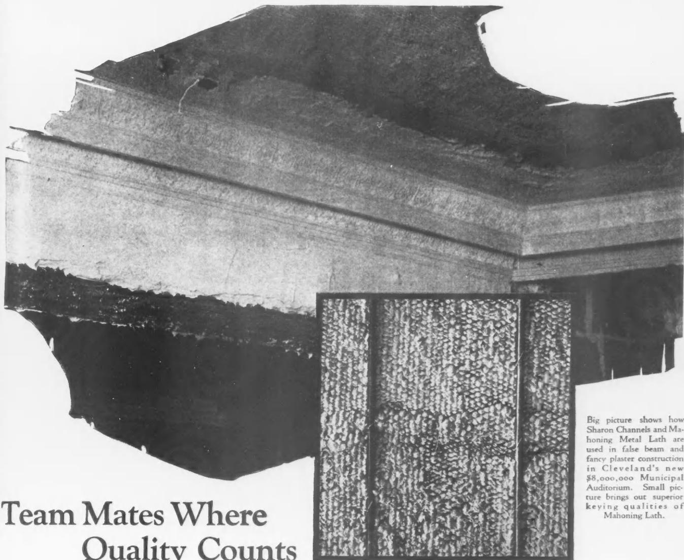
Big picture shows how Sharon Channels and Mahoning Metal Lath are used in false beam and fancy plaster construction in Cleveland's new \$8,000,000 Municipal Auditorium. Small picture brings out superior keying qualities of Mahoning Lath.
