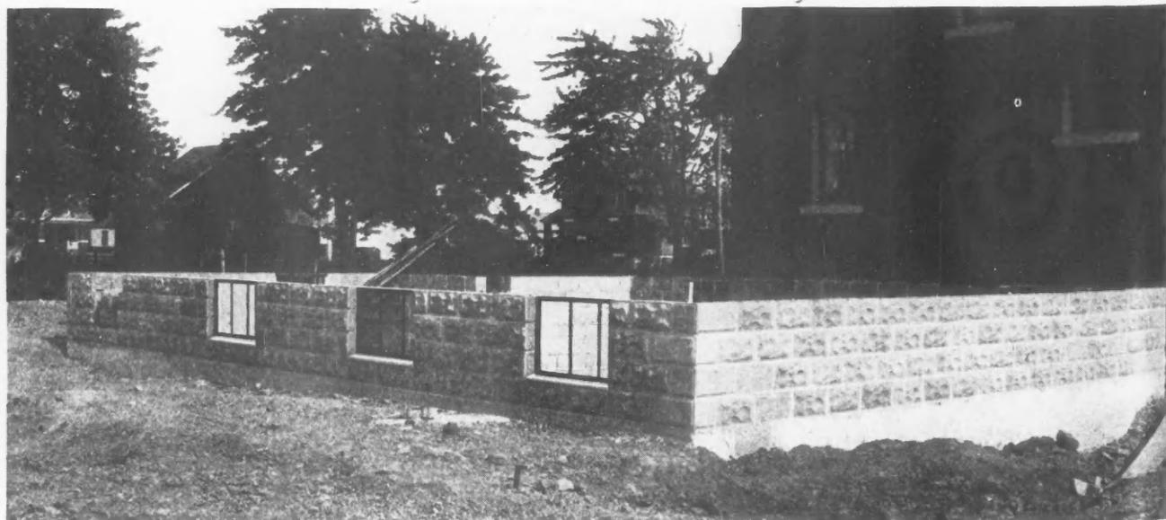
Completed Basement with Steel Sash in Place. Note the Increased Glass Area in This Type of Window. This Means More Light for Laundry and Other Rooms in Basement.
