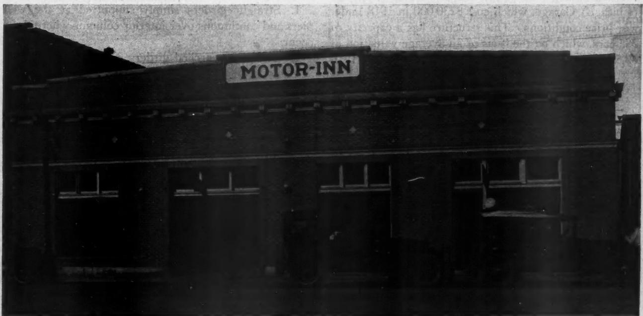
Motor Inn Garage, Detroit, Minn., Built of Concrete Brick. This Type of Fireproof Structure Is Designed to Cut Fire Risk and Insurance Rates, and Remove Menace of Public Parking.
