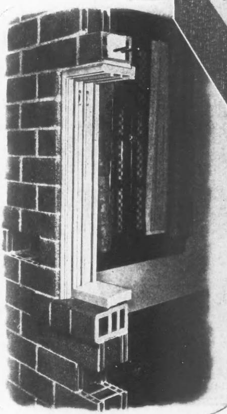
Section shows sill tile, lintel tile and joist tile in full and half lengths. Enough other special shapes are furnished to take care of ordinary residence details.
