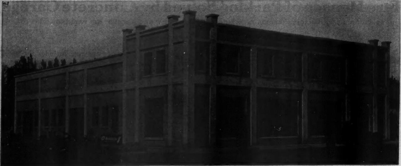
Public Garage at Ellendale, N. D., W. E. Hart, Owner, Built of Reinforced Concrete J. W. Finkle & Son, Contractors. It Has a Stucco Coating and Is Designed to Be Fireproof. It Has a Show Room With Offices Above.
