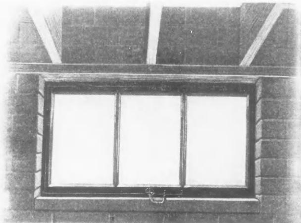
Another Type Basement Steel Sash, Showing Permanent Lock Attached.
