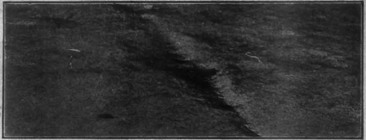
The Rut in This Floor Is at a Joint or "Seam" in the Concrete. Very Often When These Joints Are Not Well Bonded, a Line of Weakness or Soft Spot May Develop. Such a Line of Weakness, if Traversed Daily by Heavily-Laden, Metal-Wheeled Trucks, Will Wear Into Holes. When Trucks Begin to Bump Into Such Holes, Not Only Do the Rutted Sections Wear Faster, but the Entire Surrounding Surface as Well.
