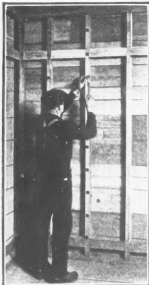
**Fasteners Are Nailed to Intermediate Studs (or Furring Over Old Plaster) Every 9 Inches.**
