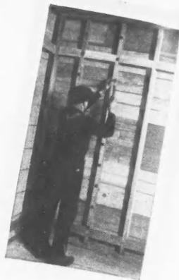
Fasteners are nailed to intermediate studs (or furring over old plaster) every 9 inches.
