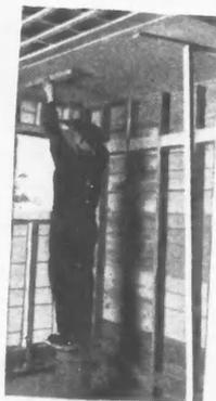
Always apply ceiling first. Apply fasteners as for side walls, nail one end of panel, and drive onto fasteners, as shown.
