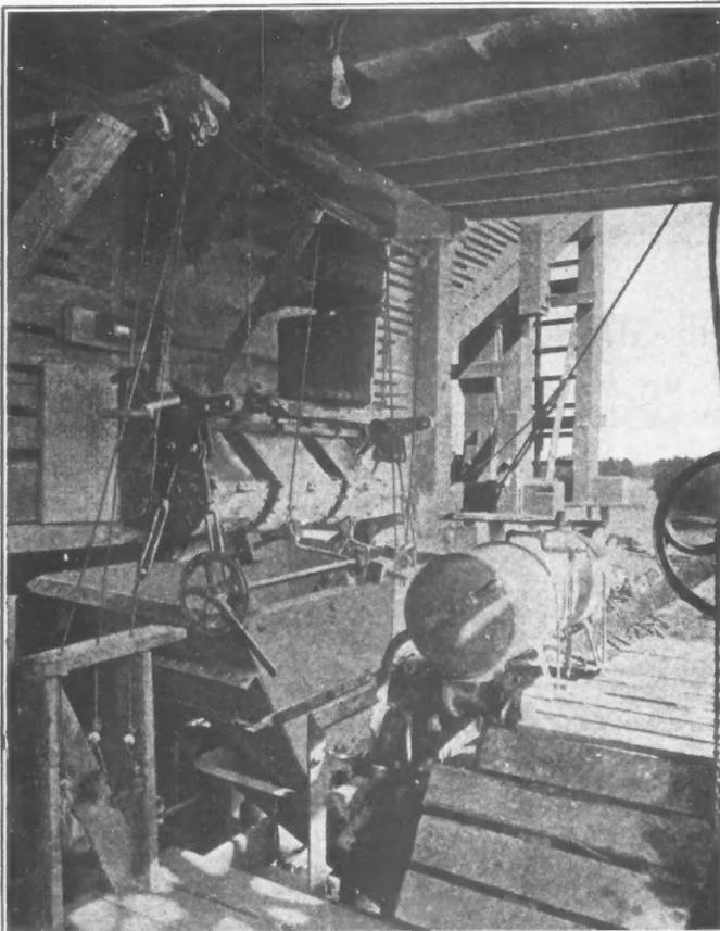
New Proportioner in Action. This Ingenious Device Measures Aggregates by Weight Eliminating Any Guesswork in Mixing the Concrete.
