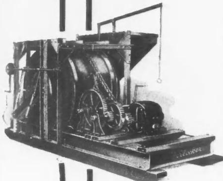
Sizes 4, 5, 7, 14 and 21 cu. ft. mixed material—on skids with batch hopper and electric motor.
