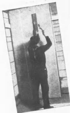
Panel is nailed at top. A piece of 2 x 4 is laid over studs, and struck with heavy hammer blows. Fasteners clinch into back of board.
