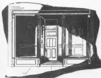
It is a simple job to tear out an old-fashioned front. Shoring up the upper structure and installing an I-beam requires little equipment. Fitting the building for the new Desco store front takes but a short time ordinarily.
