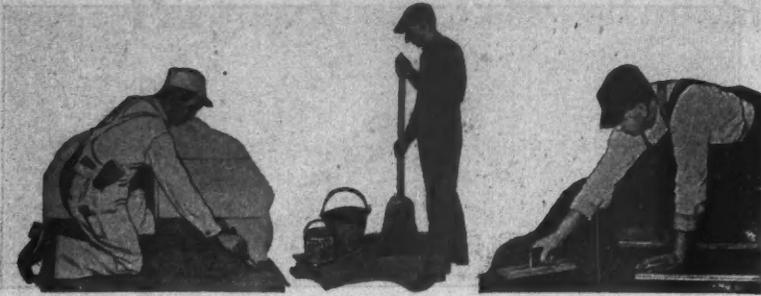
At the Left Illustrating Surface Film Treatment, at the Right Mechanically Hardening and in the Center Chemically Hardening.
