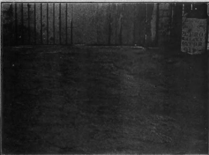
Photograph of a Cement Floor in a Shipping Room Where Proper Hardening Precautions Had Not Been Taken. Observe That Topping Has Been Completely Worn Off, Prominently Exposing Stone and Coarser Aggregate.
