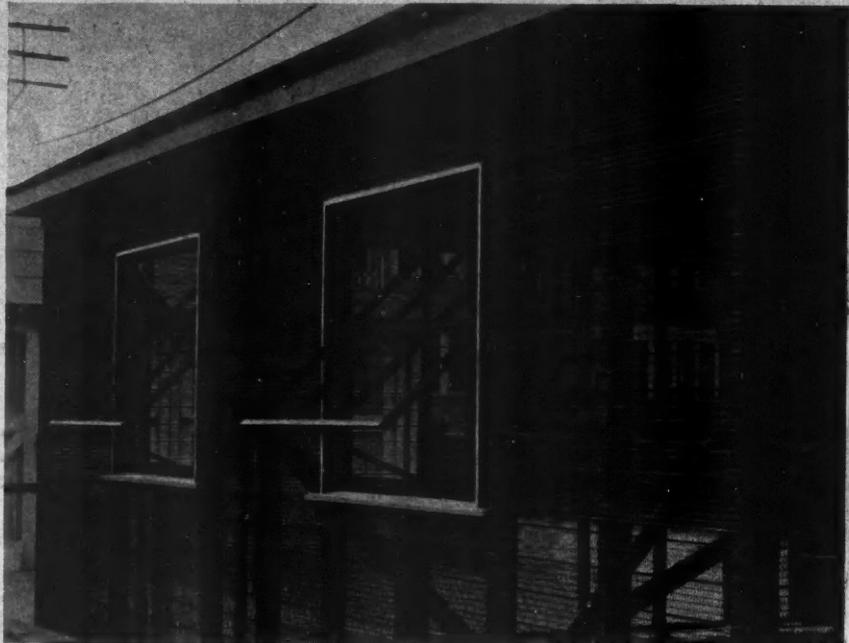
Small garage under construction fitted with steel sash. Stucco will be applied to this skeleton work of metal lath, making a fireproof structure. The sash are pivoted.
