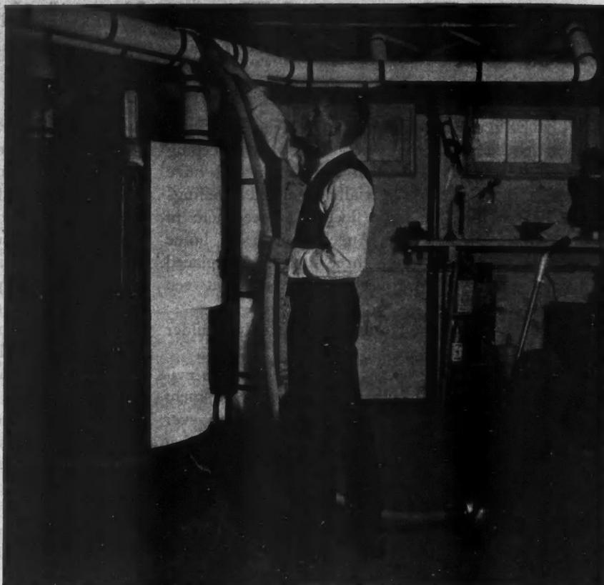
Vacuum cleaner attachment for cleaning heating pipes and other "hard-to-get-at" places in the collar. The placing of outlets makes electrical convenience possible.
