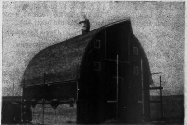
Fig. 2. Barn Built by Same Man. This Barn Is 30 by 40 Feet, a Popular Size and Style in the Dakotas Because of its Strength and Large Hay Mow.
