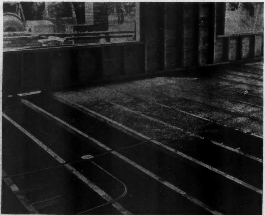
Steel Lumber Joists Covered with Metal Lath. Nailing Screeds Have Been Nailed Over the Lath Parallel with the Joists and About Two Inches of Concrete Filled in Between the Screeds.
