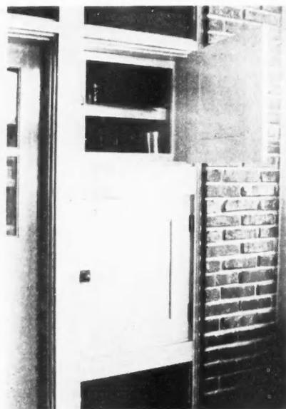
**Combination Summer and Winter Ice Box Built in Wall. The lower Door (Closed) is the Door for the Refrigerator Thru Which the Iceman Places the Ice from the Outside. The Door Above is the Opening for a Winter Ice Box. Food is Kept Well in this Receptacle Without Ice.**
