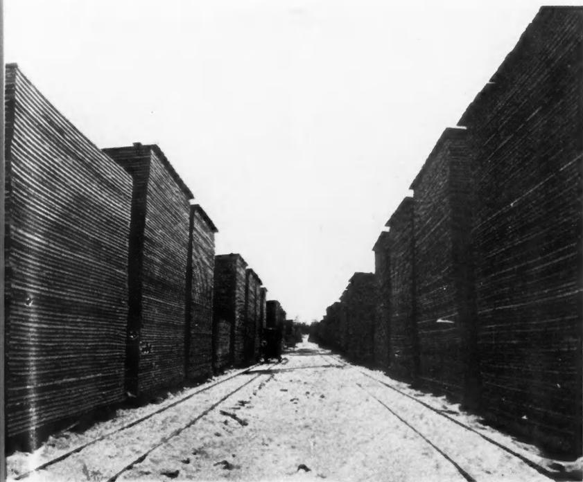
Millions of Feet of Lumber Piled Properly. The Foundations Are Concrete and Each Layer Is Carefully Separated to Allow Proper Seasoning Without Warping or Checking.
