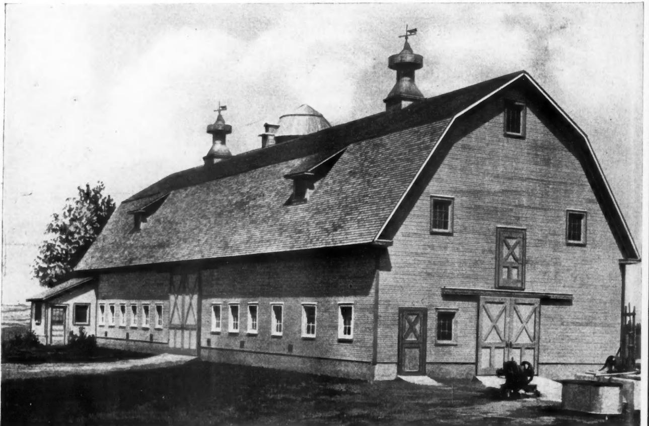
Excellent Type of Dairy Barn with Forty Cow Stalls, and Special Bull and Calf Pens. This Is Built of Heavy Timbers, Frame Siding, Solid Concrete Foundation and Has Easy Sliding Doors and Ventilation System. Dimensions, 36 by 106 Feet. The Gambrel Roof Permits of a Large Haymow.
