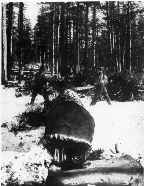
Bucking the Log—Mighty Western Pine Laid Low. It Is Being Sawed Up Into Sections Preparatory to Shipment to the Mill.
