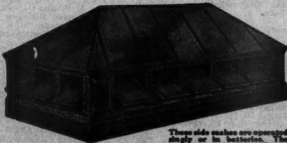
These side casings are operated simply or in batteries. The casings are pivoted and very easily operated.
