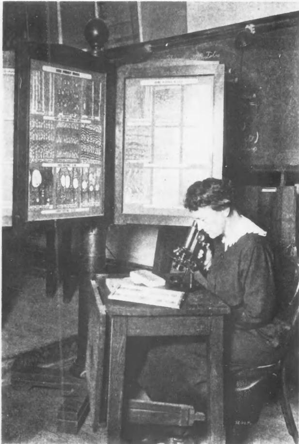
Timber Experts Can Identify Wood from Any of Our Native Trees by Examining it Under the Microscope. The revolving chart above shows the diversity in wood structure brought out under the powerful lens.
