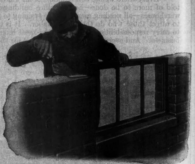
Mason Insets Anchor Clip in Channel Groove.
