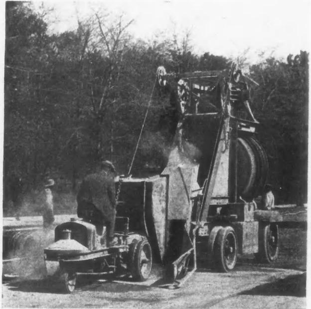
**Milwaukee Firm Uses Rubber Tired Pavers Because They Transmit Few Shocks and Are Easier on the Pavement.**
