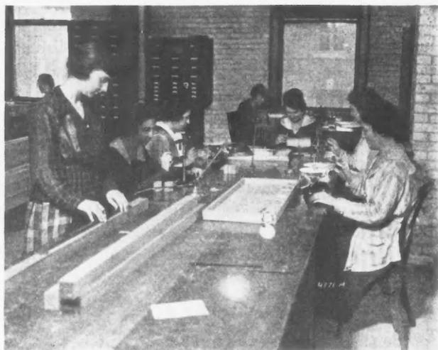
**Ascertaining the Moisture Content of Wood Samples by Simple Tests.** A knowledge of the moisture content of the stock makes it possible to avoid costly manufacturing difficulties.
