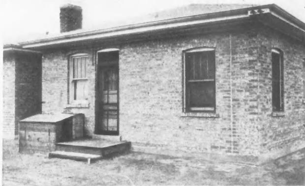
Rear Wall of a Garlow Showing 18 Ft. Built-in Steel Beam Construction. The brick beneath the beam is built into a panel which can be removed without disturbing the rest of the wall. This leaves a space for swinging the garage doors.
