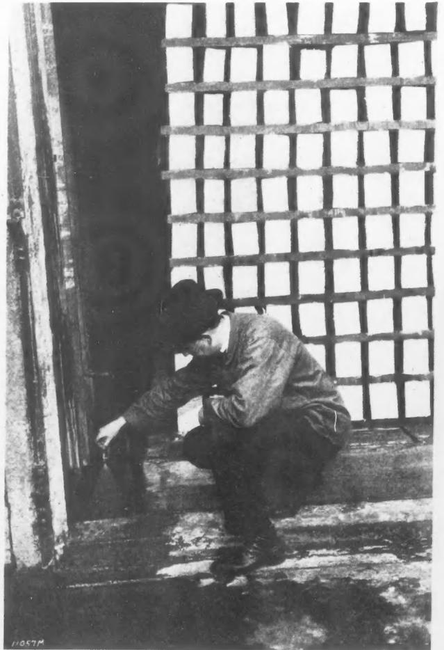
The National Timber Experts Have Invented a Valuable Water-Spray Kiln in which Humidity Can Be Controlled Artificially. The drying rate of the lumber is regulated by conditioning the air with sprays of water whose temperature is carefully regulated.
