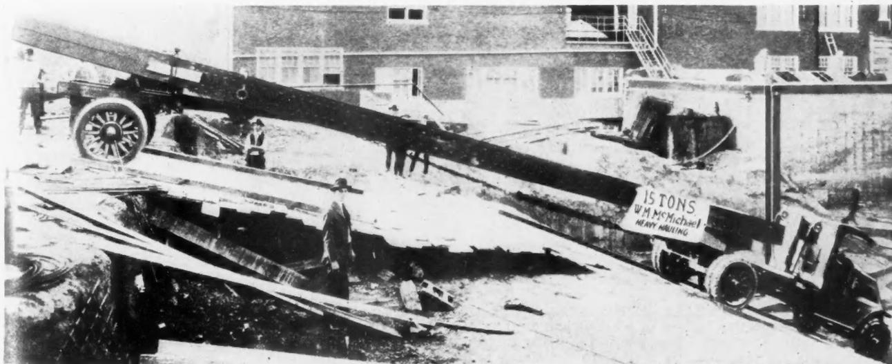
W. M. McMichael of Tulsa, a Hauling Contractor, Transported a Number of Massive Steel Beams from the Railway Cars to a New High School Site by Using a Regular 5½-Ton Dump Truck in Connection with a Trailer. In spite of twists and turns and steep inclines, the job was accomplished successfully and without mishap.
