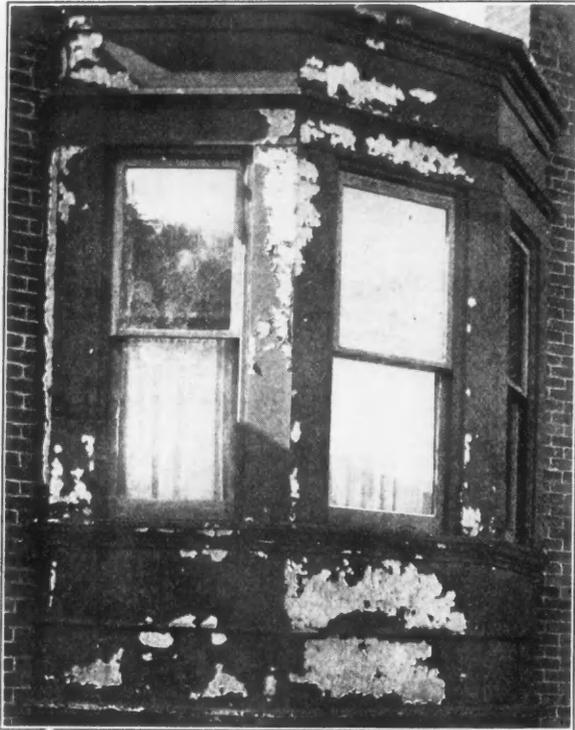
**No More Need to Feel Discouraged Over the Non-Adhesiveness of Paint Applied to Galvanized Iron. A newly invented paint combines with the galvanized surface and gives a non-peeling finish resembling stone.**
