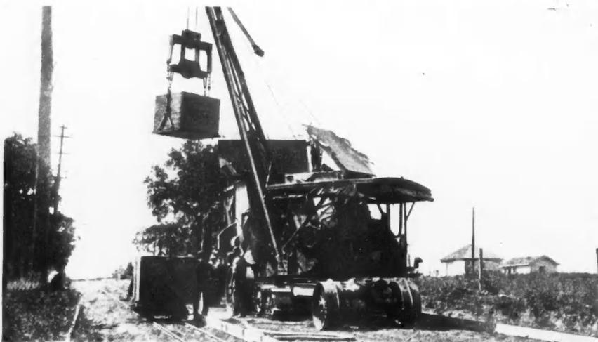
Dump-bottom Batch Boxes Were Hauled in 15-car Trains to the Mixer, Where the Crane Bridle Picked Them Up and a Tug of the Releasing Line Dumped the Contents Into the Charging Hopper.
