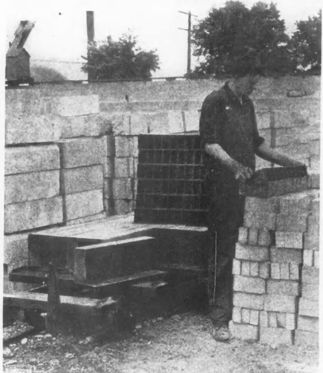
This Shows How Cement Brick May Easily Be Handled, Ten at a Time. After the molds have been entirely removed and the brick placed in piles, the workman quickly sets the molds back into place and the truck is rolled back to the mixer for filling.
