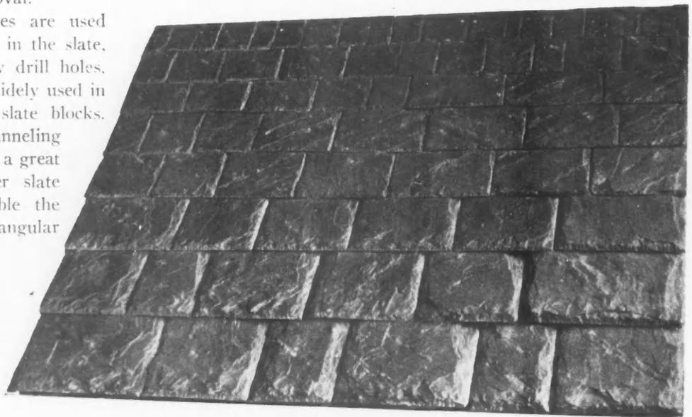
A Rustic Roof of Attractive Design, Made of Architectural Grade Slate. Not the least attractive part of a slate roof is this rugged, irregular, artistic effect. Properly manufactured roofing slate, laid according to established practice on uniform and strong supports of moderately steep pitch, provide a roof that will not leak.
