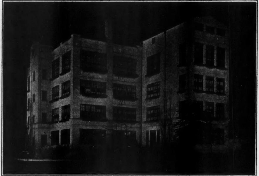
Floodlighting Installation, Night View, Wheatena Company, Rahway, N. J. This Is Lighted from Four Stations, the Projectors Floodlighting the Plant from All Four Sides.
