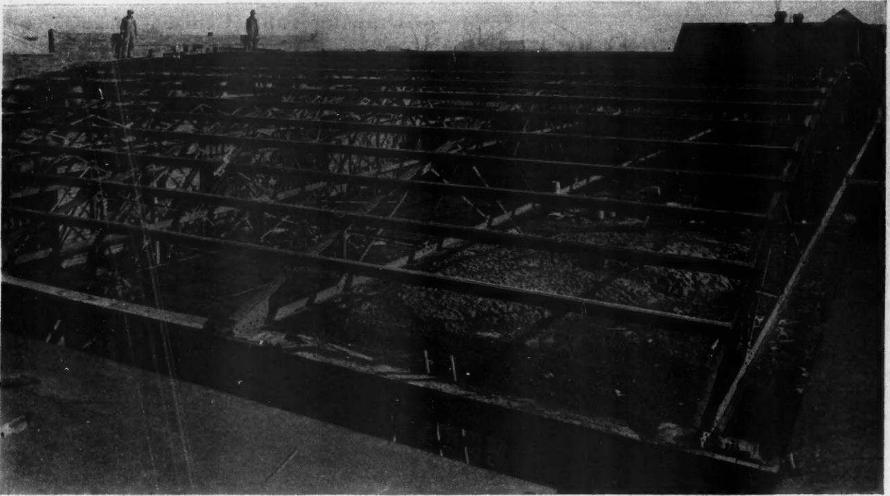
Do You Know That You Can Build Garages Like This, with the Whole Organization of a Structural Steel Company Behind You as Though It Were Your Own? The bowstring truss as shown has come to be the accepted style for public garage roofs.
