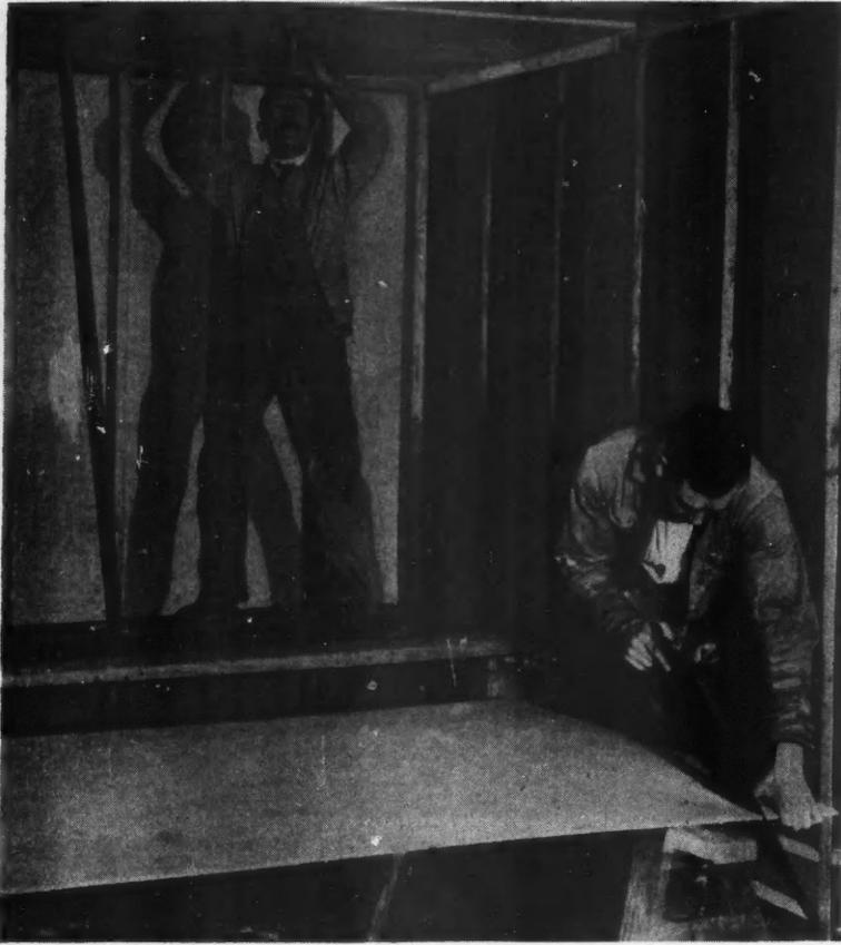
This Gypsum Wallboard Is Handled as Easily as Lumber. The Board, Ceiling-High Sheets Are Sawed and Nailed Direct to Joists and Studs.
