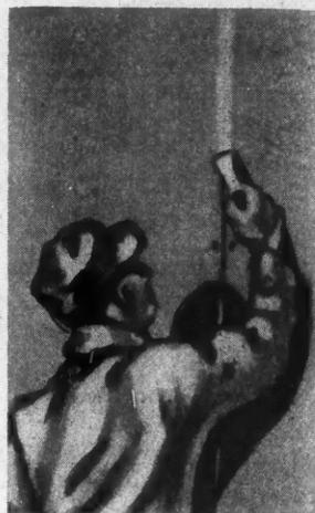
To "Spot" Nails and Eliminate Joints a Special Joint Filler Is Used.
