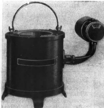
**This Bench Solder Pot Melts Solder Quickly and Keeps It at a Uniform Temperature.**
