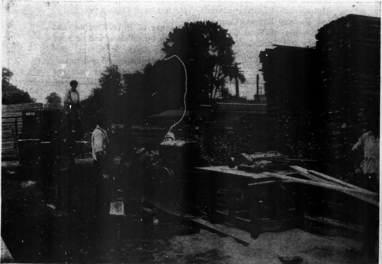
**Using a Tractor as a Power Unit to Operate a Saw in Lumber Yard. Besides Cutting 3 to 5,000 Feet a Day, Think of the Saving in Lumber Handling This Means. The view is in the yard of the Sterling Lumber and Supply Company, West Pullman, Ill.**
