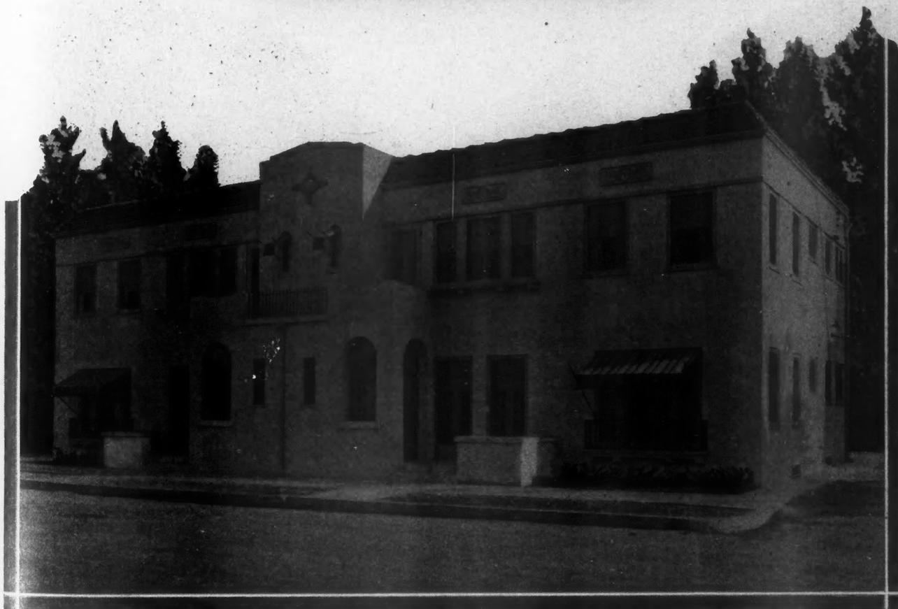
**A FOUR-FAMILY FLAT IN THE SPANISH STYLE.** Here we see Spanish architecture in a good adaptation. It will be an ornament to any street, and is sure to command high-grade tenants. The exterior is of stucco, over tile, concrete block or lath, with ornamental insets below the cornice line. In our southern and western states the usual white stucco exterior could be colored with the more vivid blues, ecrus and reds favorable to the stronger sunlight. Every flat of the four herein has absolute
