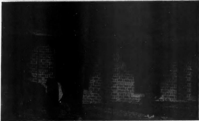
**This Fire-Resistive Test Building Constructed at the Bureau of Standards Has a Reinforced Concrete Slab Roof. The walls are brick, laid on edge, rolock method. Half the brick was subjected to a preliminary 6-hour furnace test.**
