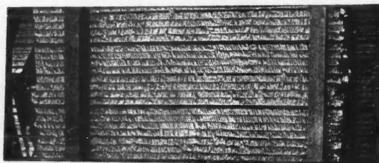
**Pictured Here Is the Combination of Metal Lath with Furring After the Plaster Has Been Applied. The rib, which serves as furring, shows plainly, running at right angles to the studding. This feature makes for strength of the product.**
