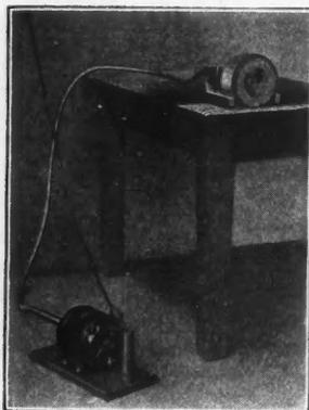
**A Power-Driven Sanding Machine Speeds Up Wood Finishing.**
