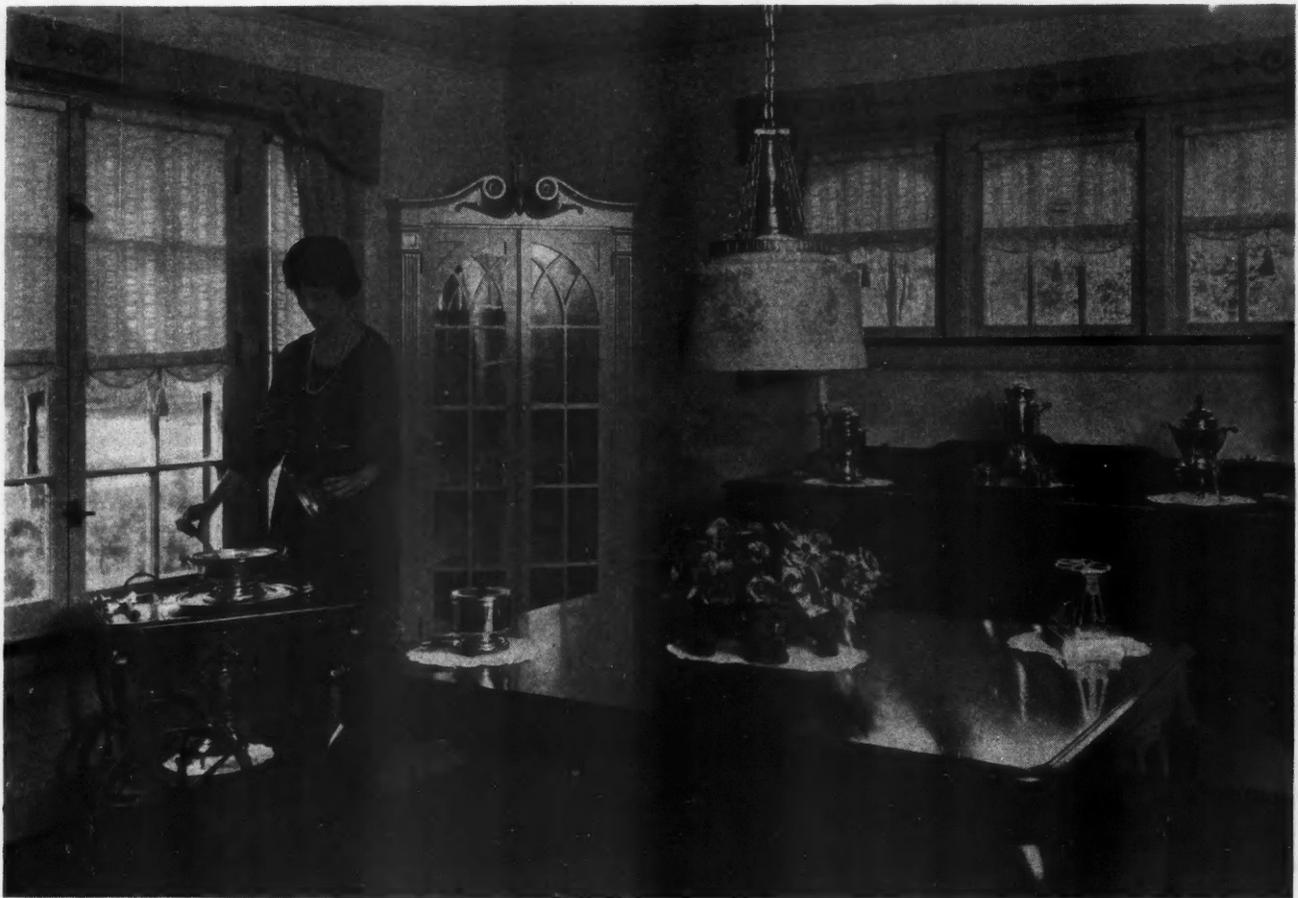
In the Dining Room of the Electrical Home Efficient, Illustrated with an Exterior View and Floor Plan in the Following Pages, the Engineers Have Fixed the Height of the Central Fixture at Just 24 Inches Above the Table Top. Notice the utility of the floor outlet.
