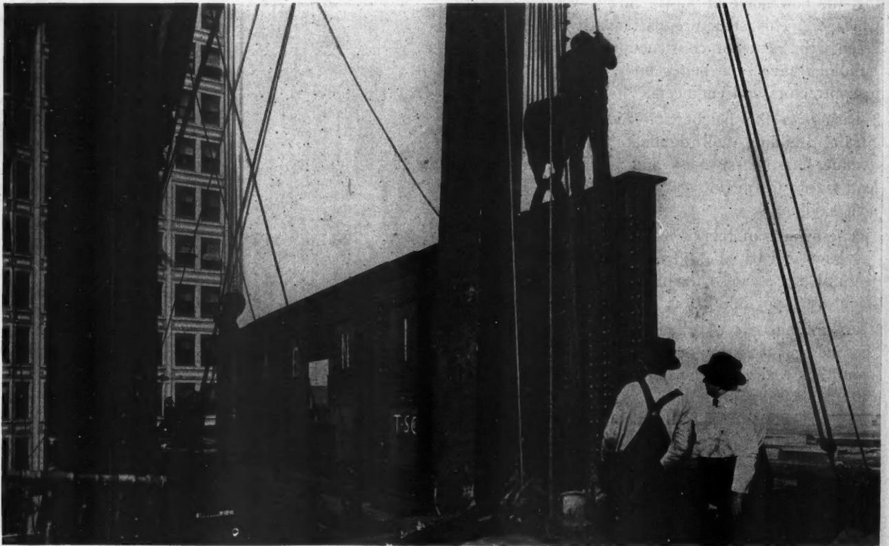
One of the 68-Ton Girders, 55 Feet Long and  $11\frac{1}{2}$  Feet High, That Carry the Weight of All of the Stories Above the Sixth Floor, Including the Weight of the Ten-Story Tower in the Straus Building. This girder, with its companion of like dimensions, makes possible the elimination of two columns.
