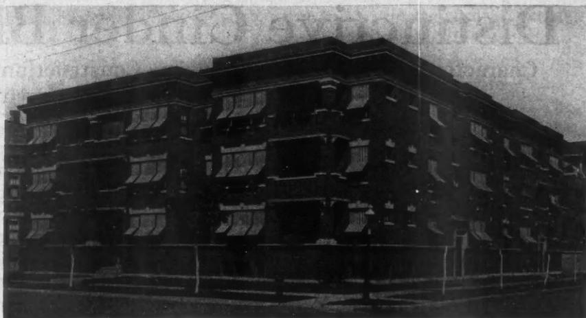
Roller Awnings Operate Like a Window Shade. The illustration shows a modification of the roller type, a cross-bar keeping the upper portion flat against the window.
