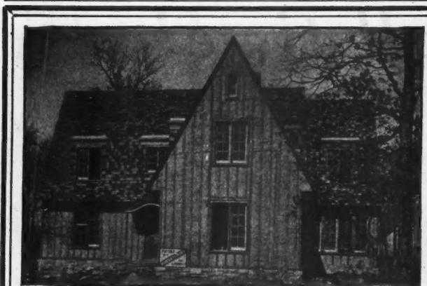
House near Chicago, showing its "underclothing" of Cabot's Quilt, with furring strips over the Quilt, on which the outside finish is laid. Roo also insulated. Leon E. Stanhope, Architect, Chicago
