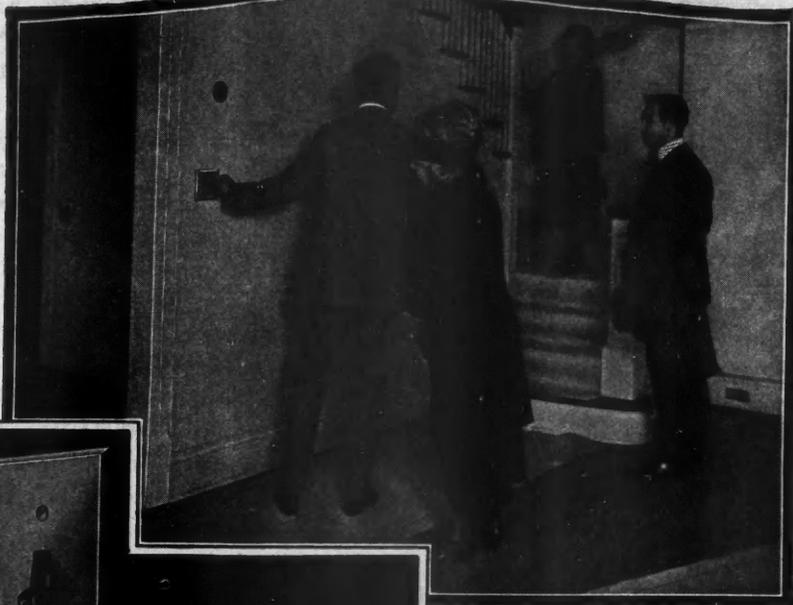
"How is the stairway lighted?"—you show them how you have provided switches—both downstairs and up—for flooding the steps with light and for turning the lights off as soon as you are up or down.
