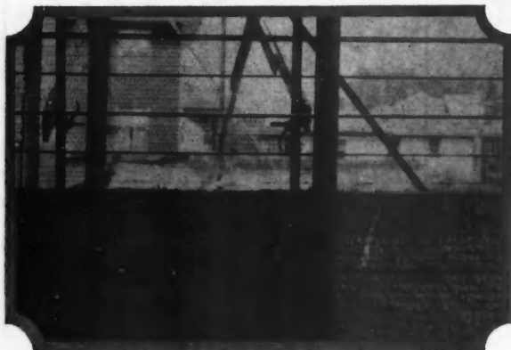
Metal Lumber studs in exterior wall of residence. \frac{3}{8} " Berloy Ribplex is attached to the exterior, and stucco is being applied. After stucco has been back-plastered, interior lath and plaster will be applied.
