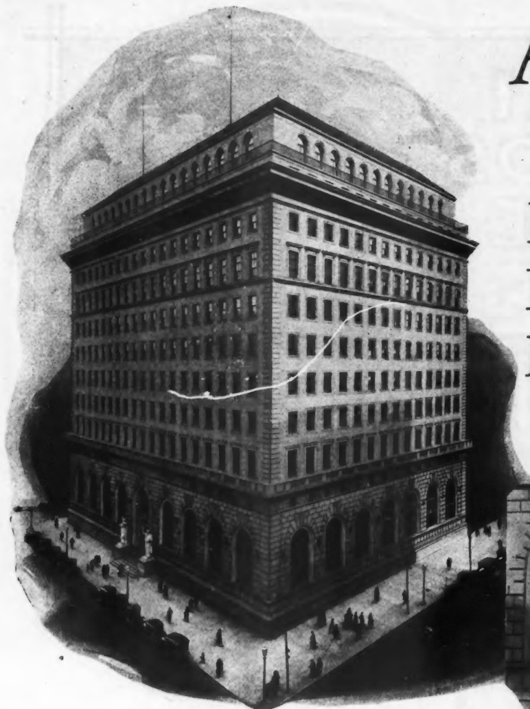
FEDERAL RESERVE BANK OF CLEVELAND Atlas White Portland Cement mortar used for setting, backing and pointing the stone.
