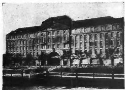
Sales Department of a Furniture Factory: In which Terranova has been used throughout; first as a beautiful wall surface that is as perfect as natural stone and again in the decorations which were cast in the same material to harmonize with the architecture of the building.
