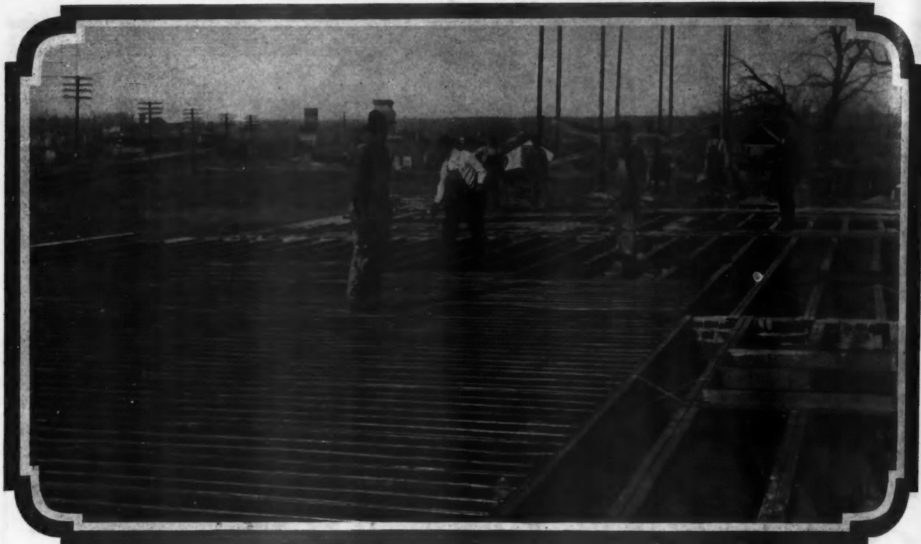
Applying the \frac{3}{8} " Ribplex to Metal Lumber joists. As the floor will be of concrete, wood nailing strips are not needed.
