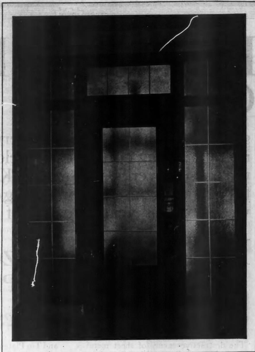
Missouri Pacific Hospital, St. Louis, Mo. C.H. Wray, Architect. E. M. Tucker, Supervising Architect. Plain Tapestry Glass with 1/2-inch mitre.
