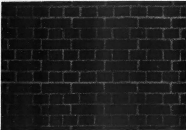
The Section of English Bond Brick Wall Shown Here Shows the Predominance of the Mortar Surface in Determining the Effect of the Wall.
