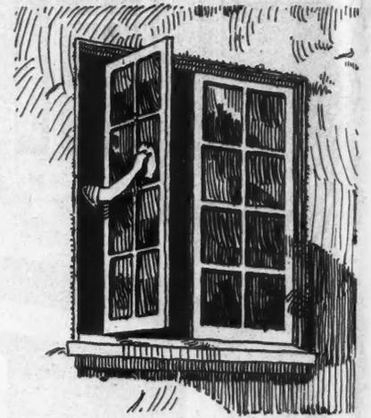
Outswinging Casement Windows Which Can Be Washed From Inside the House Are a Convenience Which Will Be Appreciated by the Housekeeper.
