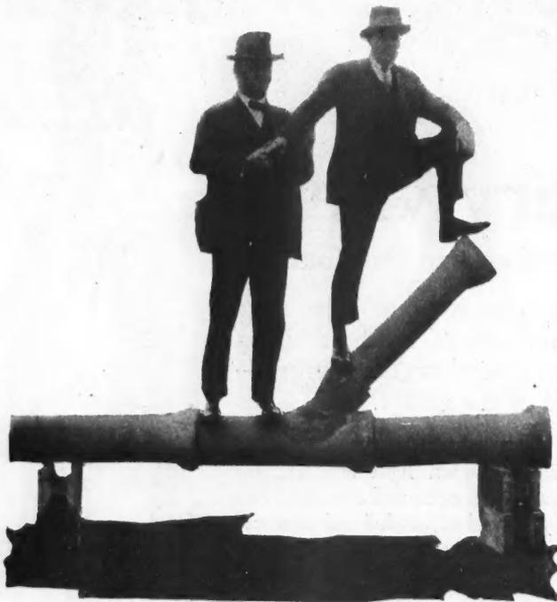
A Joint for Sewer Pipe Has Been Developed. Its strength is shown by the illustration. Manufacturers claim for it the additional advantages of flexibility and ease of application.
