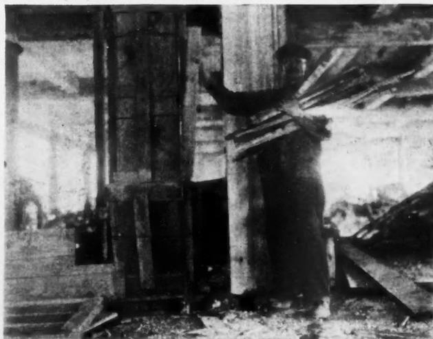
All Debris and Pieces of Wood Are Removed from the Floor by This Chute Passing Through a Light Well.
