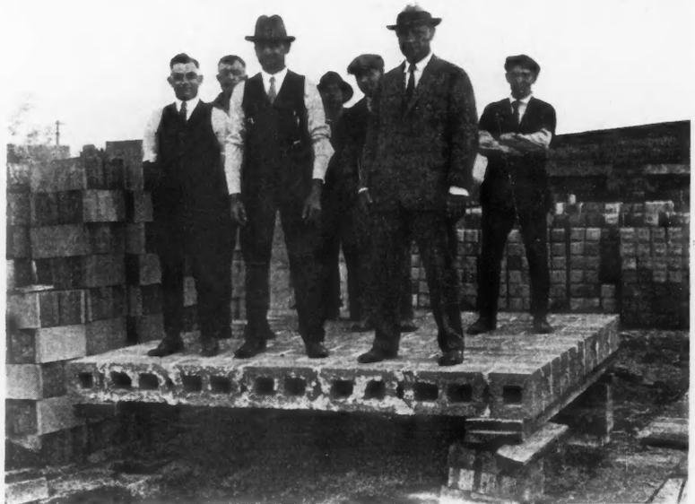
Eight by 8-Foot Straub Block Wall Laid Down; Supported Seven Men and Several Cinder Blocks Before Rupture. Note mortar joints—battered on edges only.
