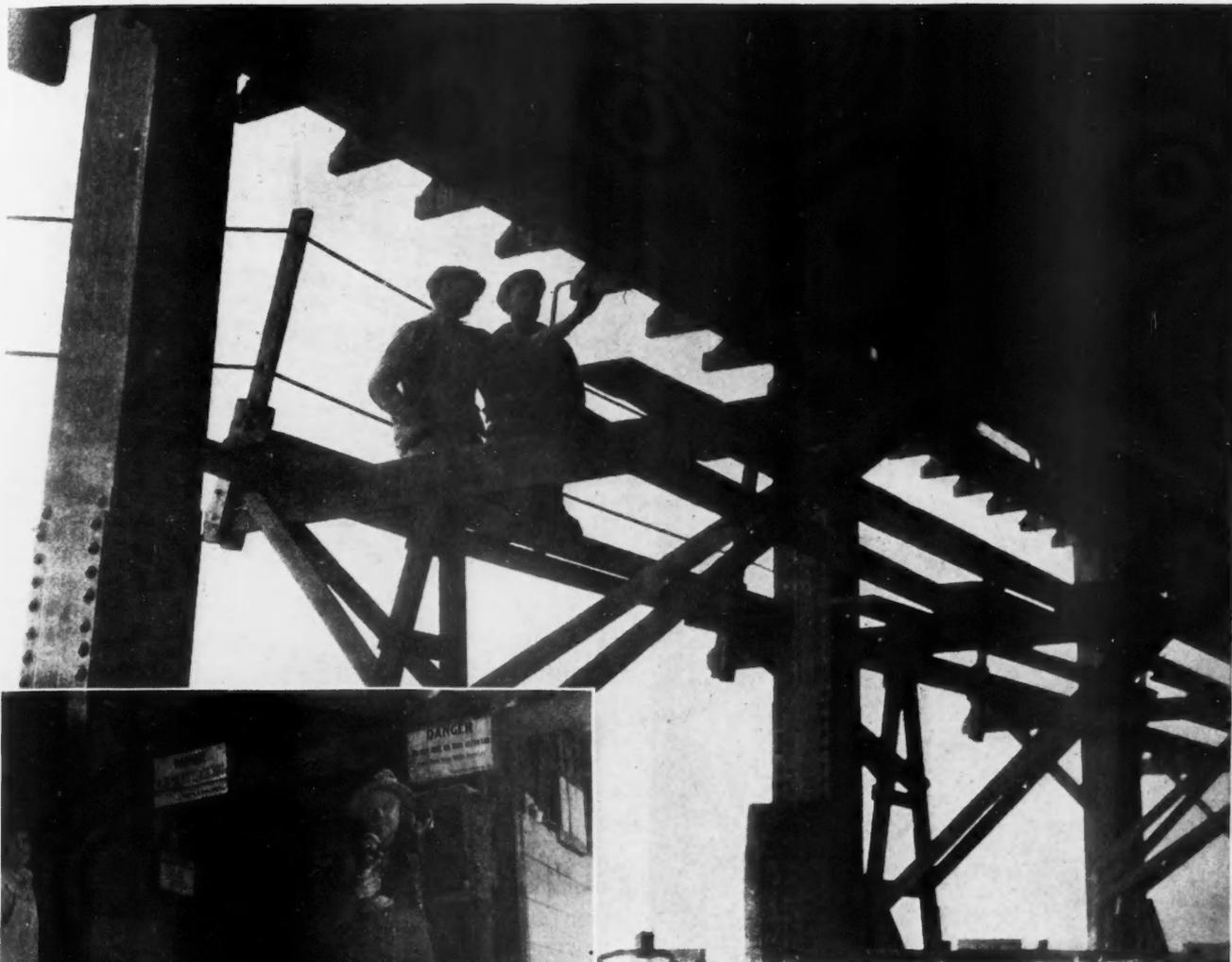
Men Working on the Outer Edge of the Outriggers' Scaffold, Stripping Cement Forms on the Outside Wall, Are Protected by the Rope Railing.
