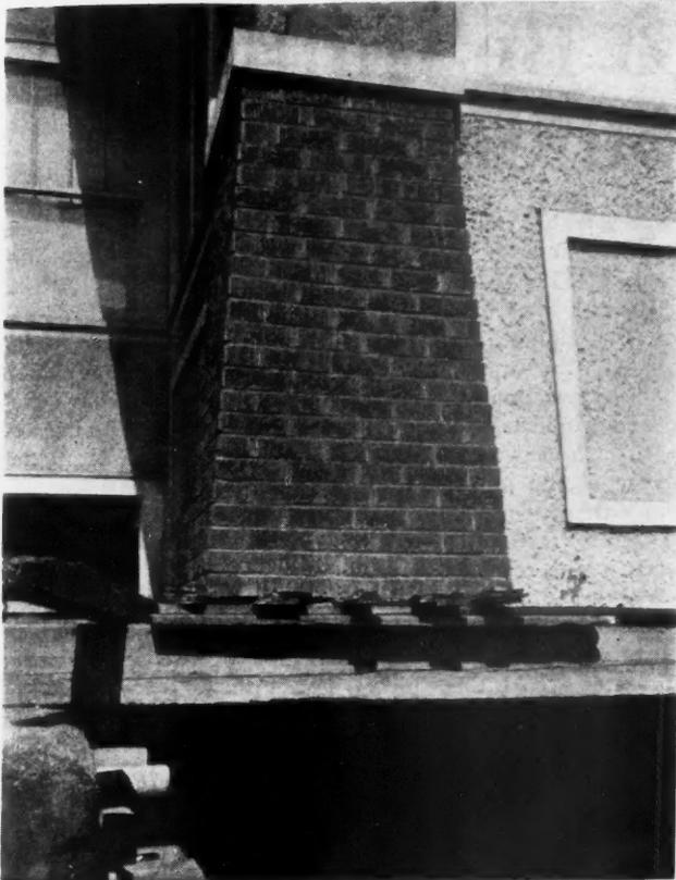
Fig. 4. The Brick Porch Piers Were Carried on 10 by 10's Placed Across the Longitudinal Timbers.
