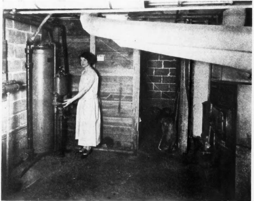
**A Water Softener Occupies Only a Small Space in the Basement, but It Makes Available an Ample Supply of Clean, Soft Water at All Times and Costs Less Than a Cistern in the Long Run.**
