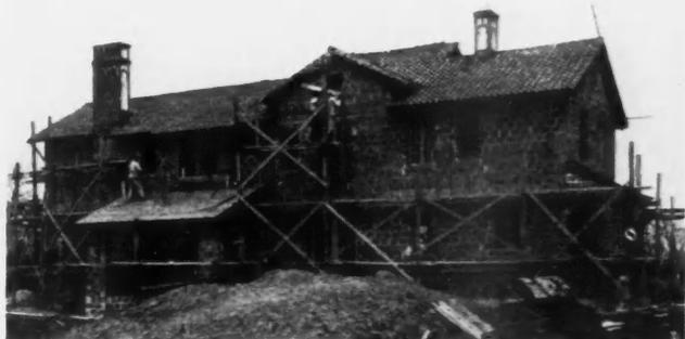
The Completed Rheinfrank Residence Is Shown Above While Just Below It Is Seen in the Course of Construction Showing the Tile Walls Construction.
