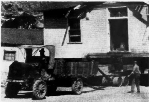
Fig. 5. Popular Steel Wheel Truck for House Moving in Use at Genierco, New Mexico.
