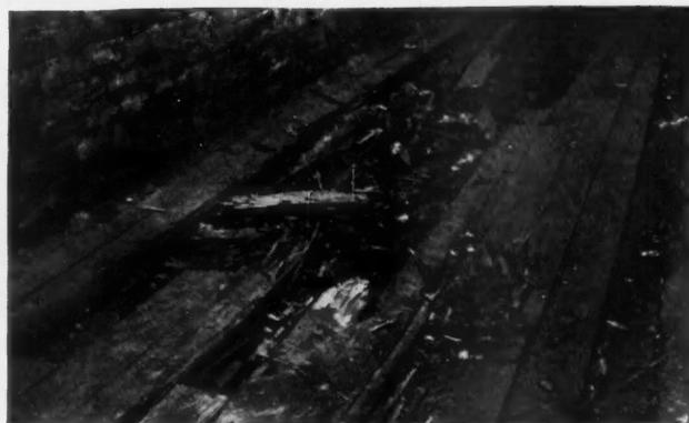
Rot Is Caused by Fungi Which Exist in All Moist Earth. These boards laid directly on the ground, with no paint protection, decayed in a short time.
