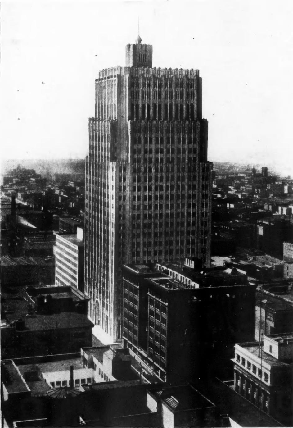
Photography and Modeling Cleverly Combined. This halftone reproduction is from a composite photograph showing cardboard model of coast division building of Pacific Telephone and Telegraph Company stripped into position on photograph of actual site.
