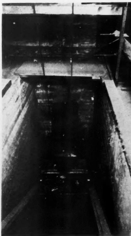
Concrete Pit for Loading the Coal Chute Bucket of the Conveyor.
