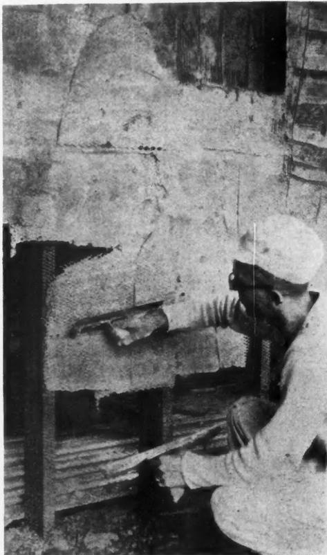
**In Order to Make a First Class Job of Plastering the Studding Must Be Absolutely Upright.**
