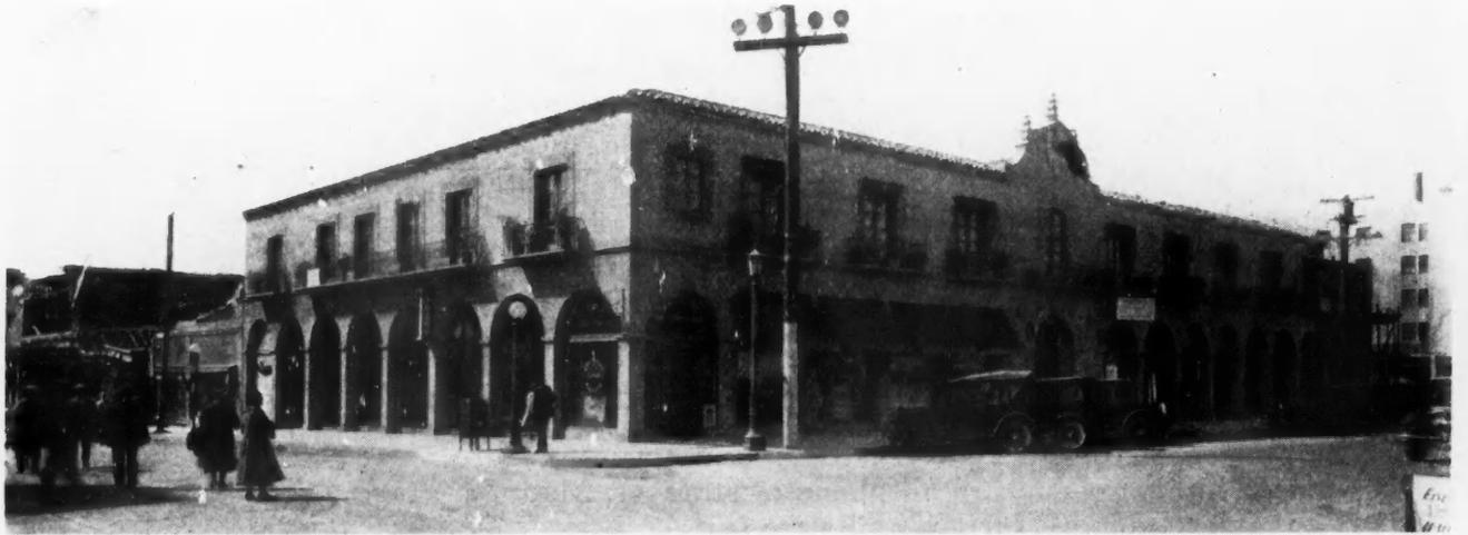
Though the Surrounding Buildings Were, for the Most Part, Either Completely Demolished, as Seen at the Left of This Photograph, or so Badly Damaged as to Be Condemned, the Carrillo Building, of Special Concrete Construction, Survived the Recent Santa Barbara Earthquake Without Damage and Was Approved as Safe Without Repair by the Inspecting Engineers.
