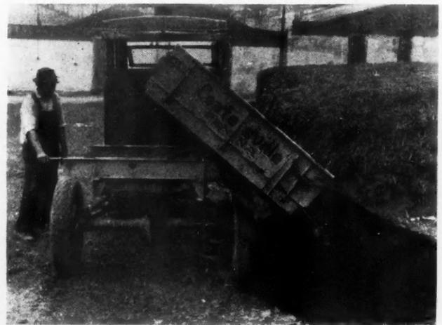
**A Side Dumping Body Which Is Easily Operated by Hand and Offers a Perfectly Smooth Bed with  $1\frac{1}{4}$ -Yard Capacity Can Be Installed on a Ford Chassis in Half an Hour.**
