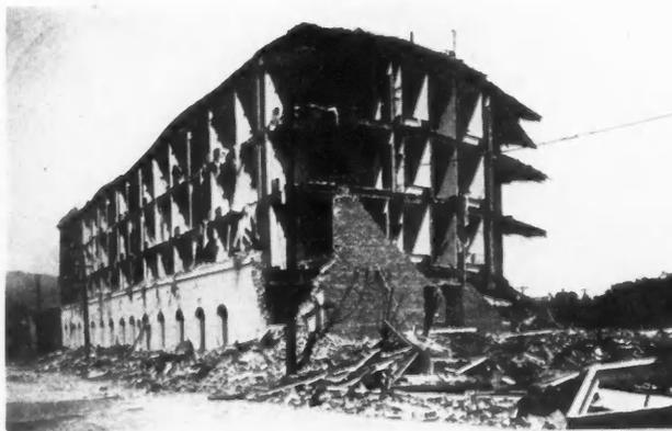
A Typical Example of the Effect of the Earthquake on Most of the Business Section of Santa Barbara Is Seen in the Wreckage of This Hotel Building with Its Walls Completely Destroyed.
