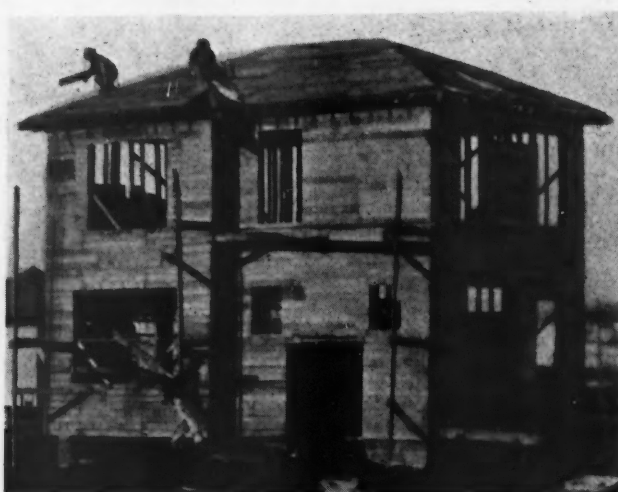
Photo 6—Here Is a House Which Is Sheathed and Roofed with 1-Inch by 6-Inch by 5-Foot \frac{1}{4} -Inch Car Roofers.
