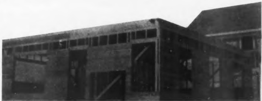
Photo 3—Here Is an Example of 7-Foot 11½-Inch Studs and Short Length Sheathing.
