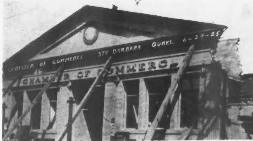
Temporary Bracing to Prevent a Heavy Cornice from Falling Into the Street. Cornices of this sort are dangerous in quake regions.
