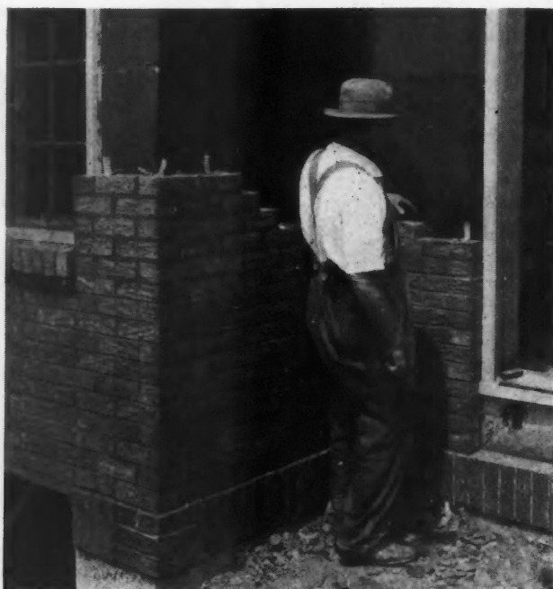
Applying the Brick Veneer for the Exterior Finish Over Walls of Structural Gypsum Concrete. The metal ties are nailed right onto the walls and are embedded in the mortar between the brick courses. Note how tight the concrete sets up against the window and door frames.
