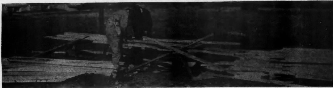
Photo 5—Cutting 8-Foot Lengths from 16-Foot Pieces. The shorter lengths would serve the purpose just as well and effect a considerable saving of lumber and labor.
