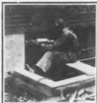
Bushing rough concrete
