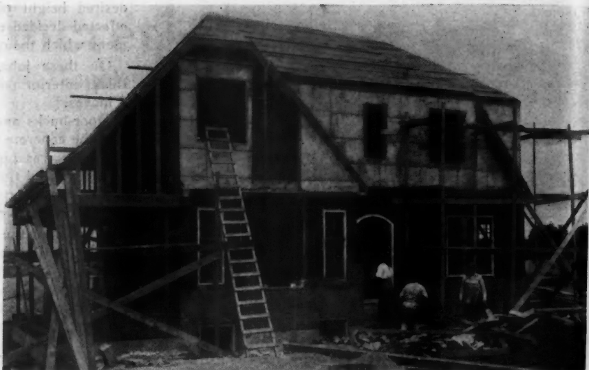
House of Structural-Gypsum Concrete as It Appears When the Walls Are Entirely Poured, the Roof Erected and the Application of the Exterior Facing and Trim Is getting Under Way. In this case, a wooden roof was used, its surface covered with asphalt roofing. The big space in the center has been left open for the chimney. The black color of the lower half of the building is due to the waterproofing compound which, at this time, had not been applied over the entire structure.
