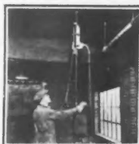
Drilling in concrete ceiling for conduit
