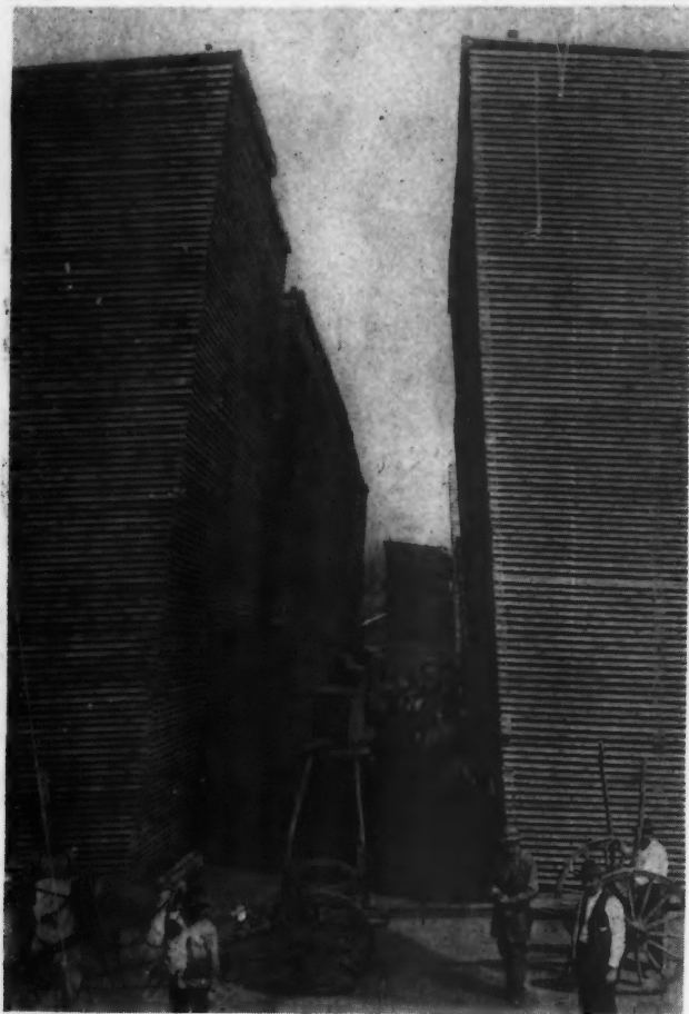
If the Ends of Lumber in Storage Are Coated with a Special Wood Preservative, Cracking and Checks Can Be Prevented Without Staining the Lumber.
