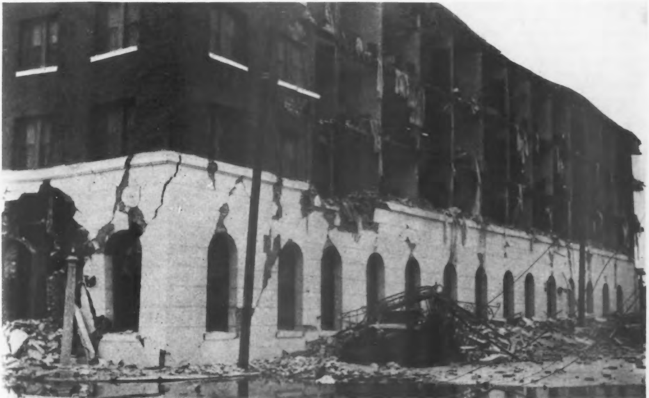
Effect of the Earthquake on a Three-Story Hotel Building Where no Brick or Tile Cross-Partitions Protected the Structure Against Side Thrust.
