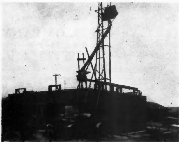
This Rig Is a Tower, of Angle Iron, Mounted on a Truck, and a Distributing Trough, for Concrete Work. Power is furnished by the truck engine.
