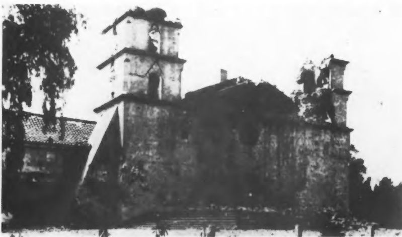
The Heavy Adobe Walls of the Old Santa Barbara Mission Made This Building More or Less Rigid and Only the Towers Were Wrecked by the Quake.
