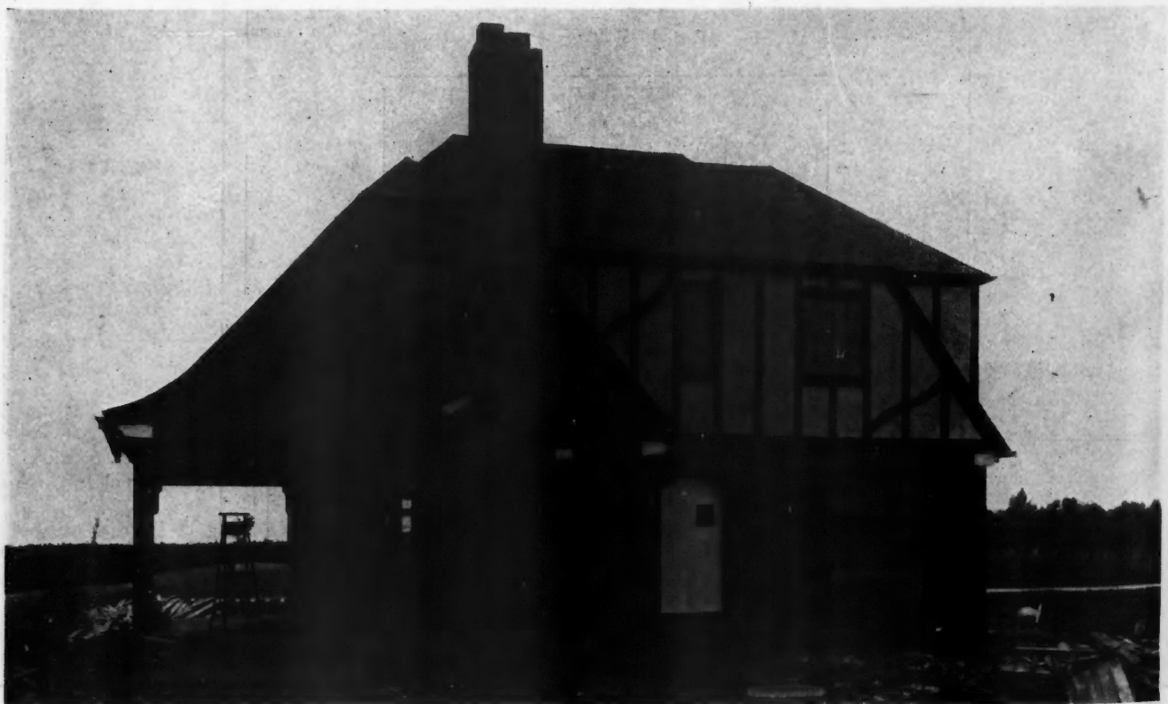
A House of Structural-Gypsum Concrete Built at Elgin, Ill., and Finished in a Combination of Brick Veneer and Stucco. The brick is tied to the walls by means of metal strips nailed to the wall and embedded in the mortar between the brick courses. The stucco is applied over a 2-inch, 14-gauge, welded steel, self-furring reinforcing fabric stapled directly to the gypsum concrete.
