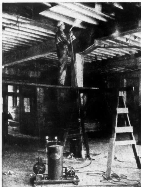
This Paint Spray Brush Can Be Obtained in Two Sizes and Either Compressed Air or Gravity Feed Types.
