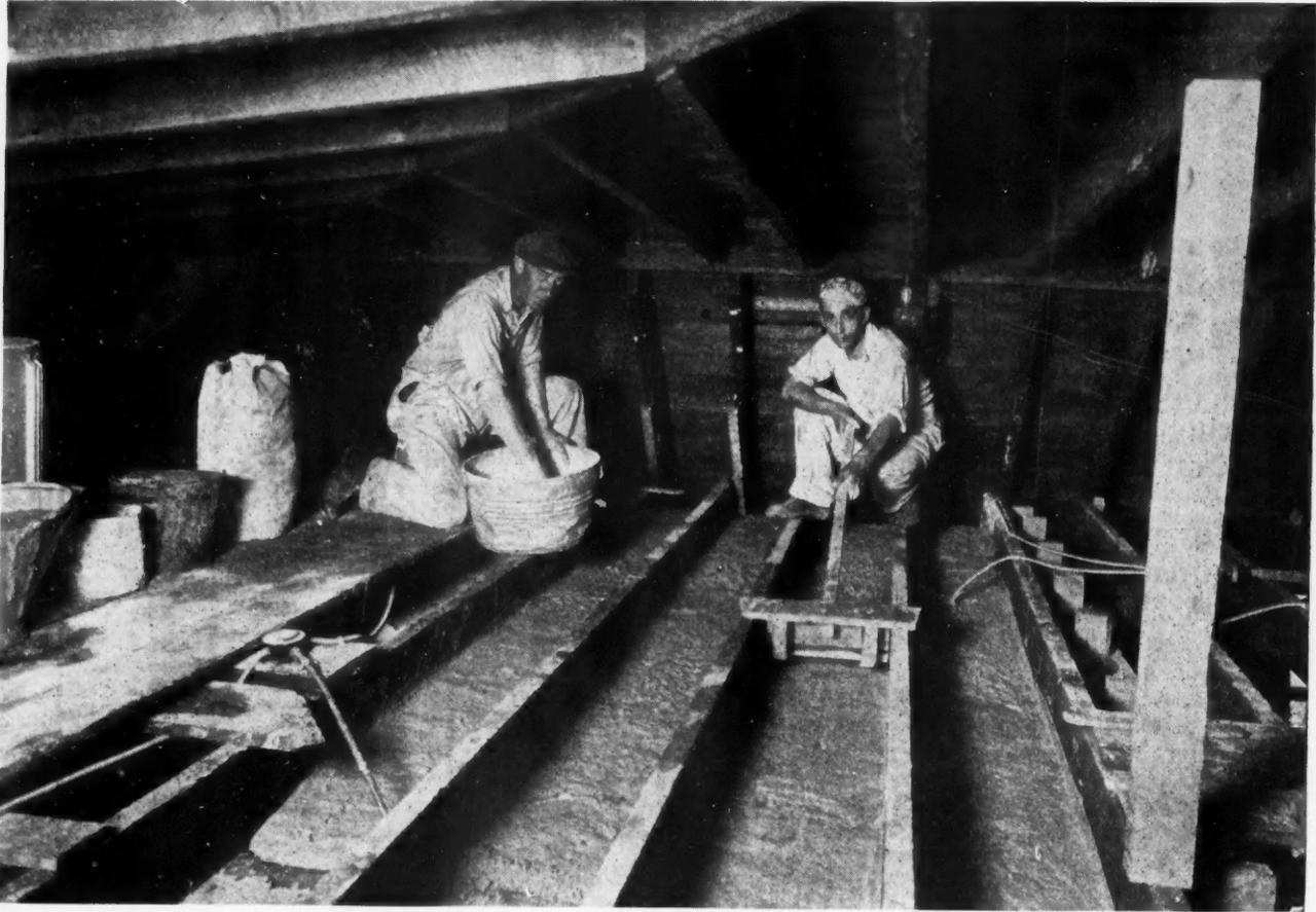
Insulating the Attic of the Buffalo Arts Club Building. The cellular gypsum has been poured over the lath and plaster forming the top-story ceiling and is being leveled to the proper thickness.
