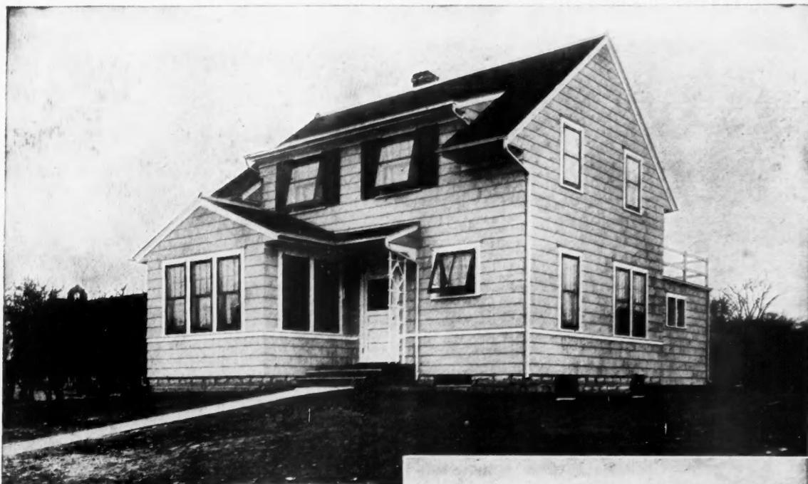
A Remarkable Change Was Made in This Old Home by the Addition of a Sun Room, Raising of the Front for Second Story Windows and a Complete New Covering of Stained Shingles.
