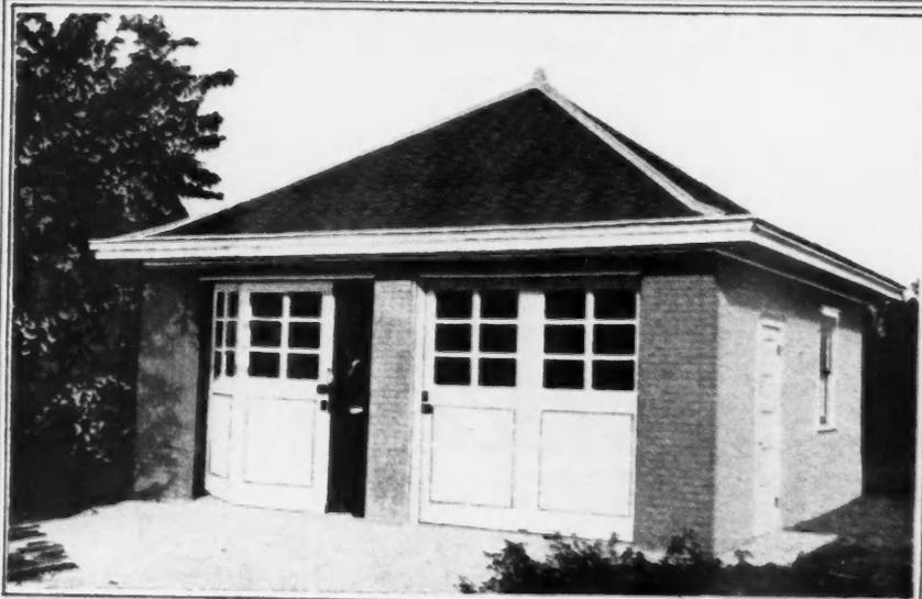
THE OSAGE GARAGE, a double garage of brick construction. Doors arranged to slide inside back around the corners.
