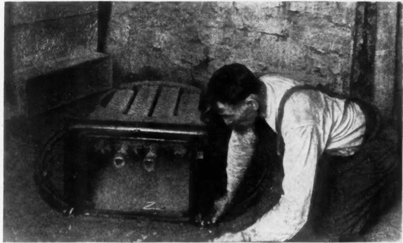
Fig. 2. Workman Fastening Bolt to Concrete Floor on Furnace Installation. The cold air duct, at the left, is ready to receive the boot connection to join at the bottom of heater casing.
