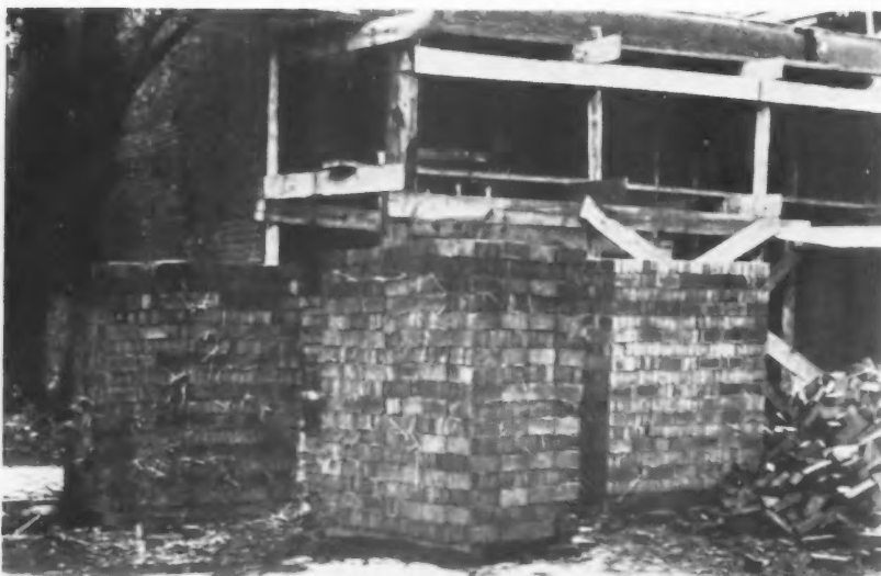
Bricks Handled in This Way Are Up Out of the Mud, Take Up Little Space, Are Easily Checked for Quantity and There Is No Wasteful Breakage.
