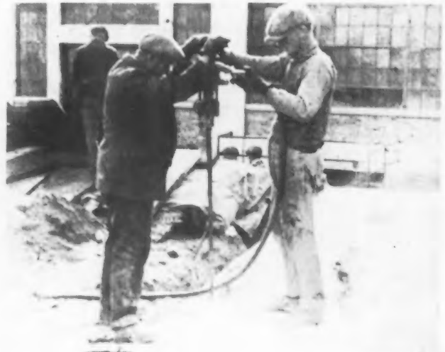
If an Engine Bed or Similar Foundation Is to Be Removed the Holes May Be Drilled Vertically and the Charges Fired One at a Time with Cap and Fuse.
