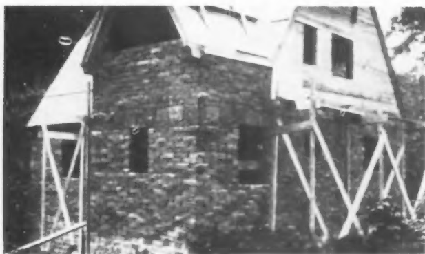
This House Under Construction Shows the Rough Wall Built of the New Fibrous Block.
