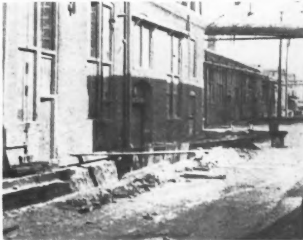
By the Use of Minimum Charges, Spaced Close Together, a Foundation May Be Blasted Without Danger to Adjacent Buildings.
