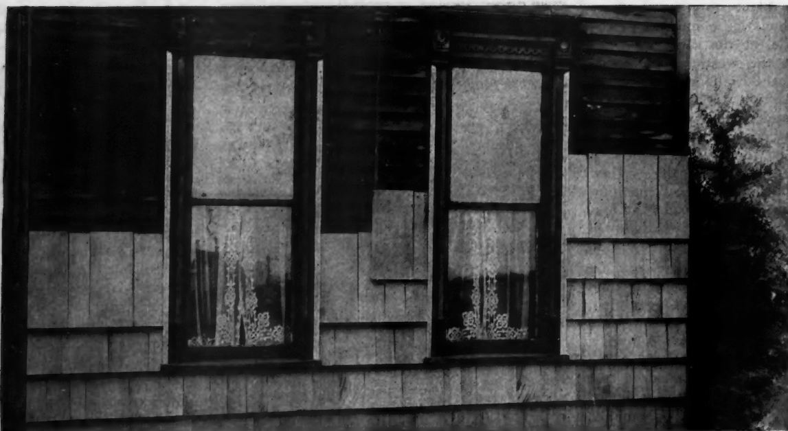
A Recovering Job Partially Complete. Note that the shingles are placed over the corner boards as well as the siding. A moulding is nailed on sides of window casings to receive the added thickness of the walls. On casings which do not have an extended drip cap the moulding should also be placed across the top of casing.
