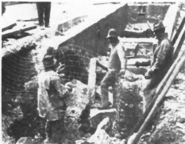
Woven Wire Fencing Will Serve as a Blasting Mat to Protect Nearby Objects Which Might Be Injured by Flying Pieces of Concrete.
