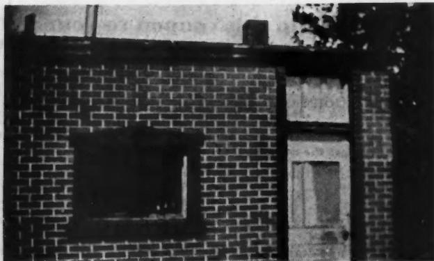
A Stucco Wall Finished with the Aid of a New Device Gives a Very Satisfactory Imitation of Brick.
