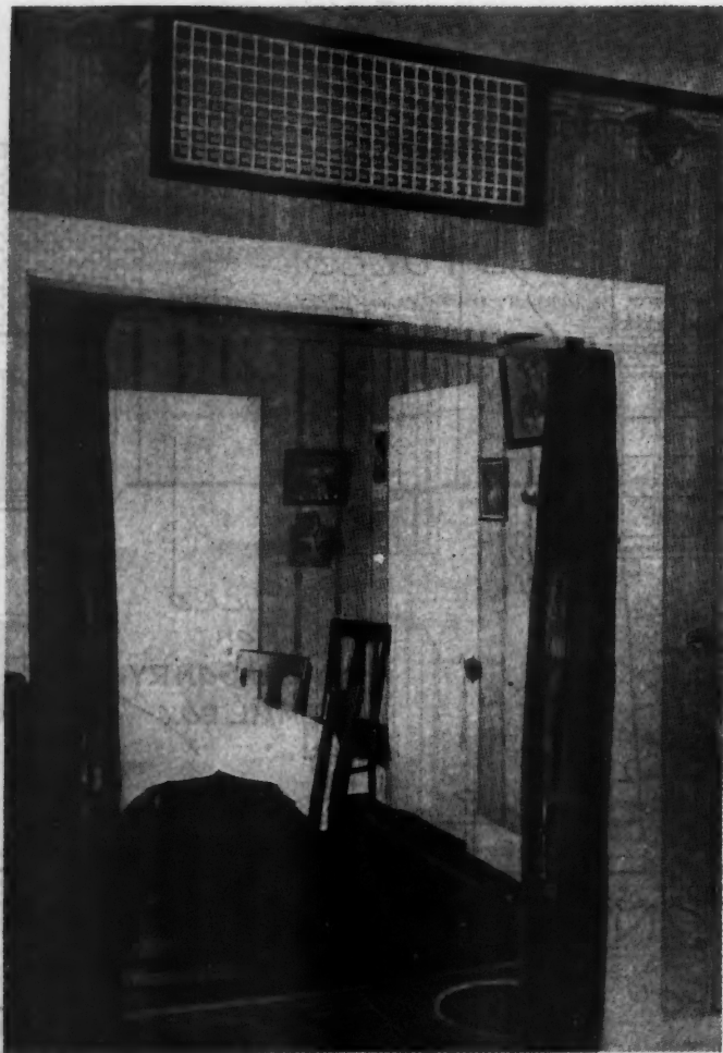
Fig. 1. A Wooden Grille Set in the Walls Over the Doorway Permits the Passage of Heat Between Rooms.
