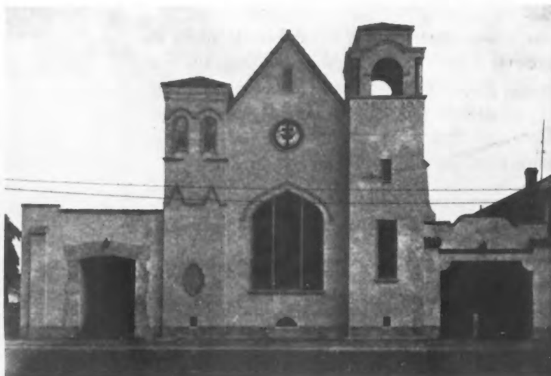
This Is How the Old Church at the Left Appeared After It Had Been Remodeled and Two Wings Added. The main structure was not changed except for the outside finish.
