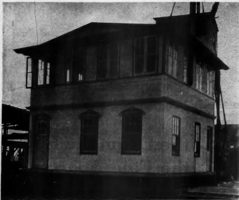
Walls, Floor, Roof and Partitions of This House Consist of Slabs of Pre-Cast, Reinforced Concrete and All Parts Were Assembled at the Building Site.
