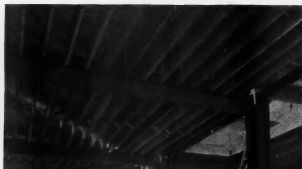
Fig. 2. Method of Framing Wood Joists to a Steel Beam. Note that the joists are tied to each other.
