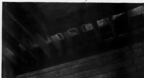
Fig. 4. This Is Not a Good Way to Frame Wood Joists to a Steel Beam for Reasons Which Are Fully Explained in the Text.
