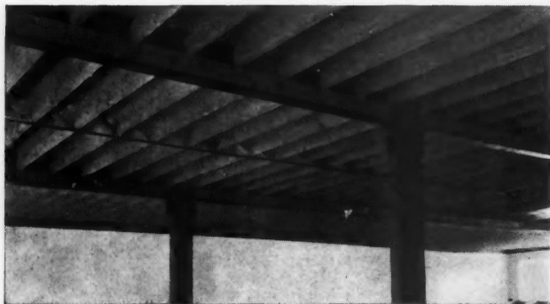
Fig. 1. Method of Framing Wood Joists to a Steel Beam by Means of a Wood Shelf.
