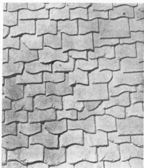
Section of a Thatched-Slate Roof
