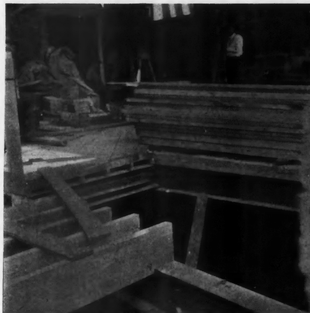
Fig. 8. Joists Coming to an End at Steel Girder Should Be Handled in This Fashion to Provide Greatest Stability.
