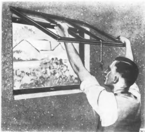
Instant Removal of Steel Basement Sash Is Possible with Sash Having This Painless Type of Hinge. The upper view shows the simple construction of the hinge.
