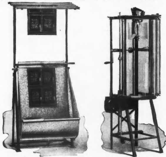
This Blueprint Machine and Sheet Washer Was Designed for the Drafting Room Which Does a Limited Amount of Blueprint Work.
