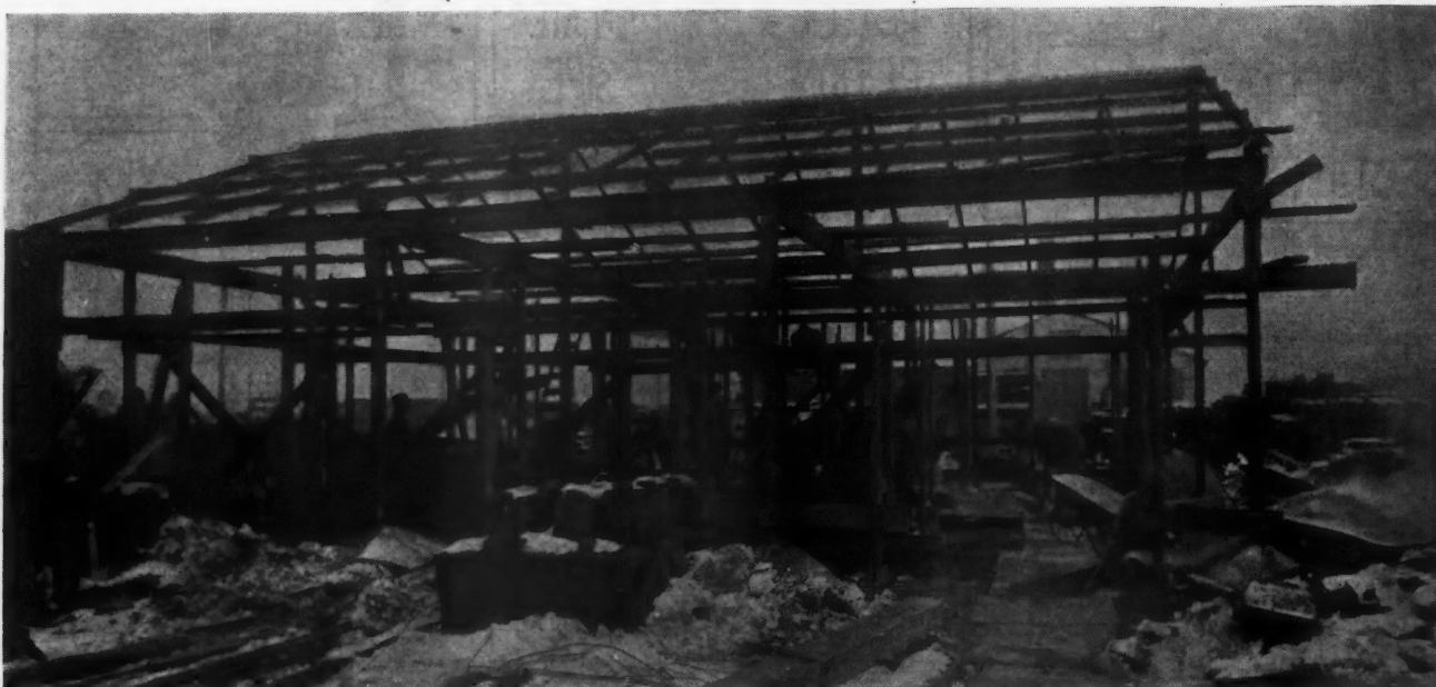
Fig. 1. An Electrical Arc Welded Building Under Construction by the Chicago, Burlington and Quincy Railroad. At the same time another building of the same size was constructed by riveting and a comparison of the costs of the two is contained in this article.
