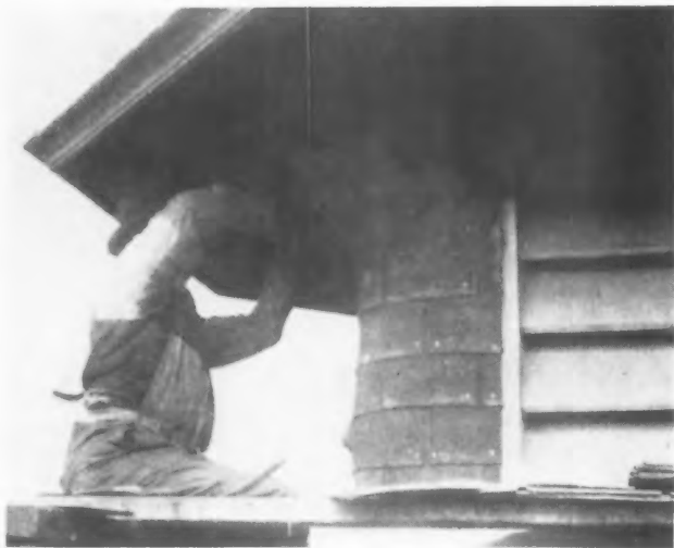
Applying Copper Coated Composition Shingles Which Bring a Copper Roofing Within the Means of the Average Home Builder.
