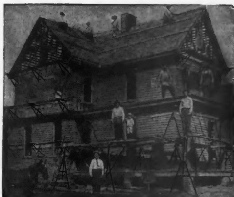
Trouble Saver Wood and Asphalt Shinglers. May be used on the steepest roofs.
