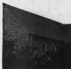
Roof of edge-grain shingles built in 1897. The owner writes: "In all these years I have spent not to exceed $15.00 in repairs and the roof seems as good as ever".
