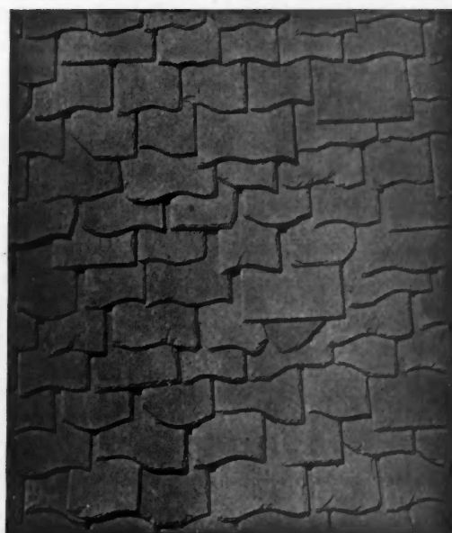
Section of a Quarry-Cleft-Slate Roof
