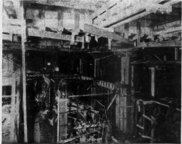
The First Floor of the New Building Which Was Built Entirely Independent of the Rest of the Building and Carried on Separate Columns and Footings.
