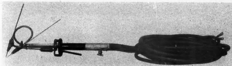
A Close-Up View of the Torch Used in the New Atomic Hydrogen Welding Process.
