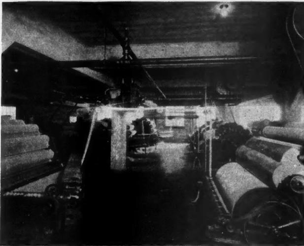
An Interior View of the New Building With the Machinery in Place and in Operation, Showing the Details of Line Shafting and Sprinkler Layouts.
