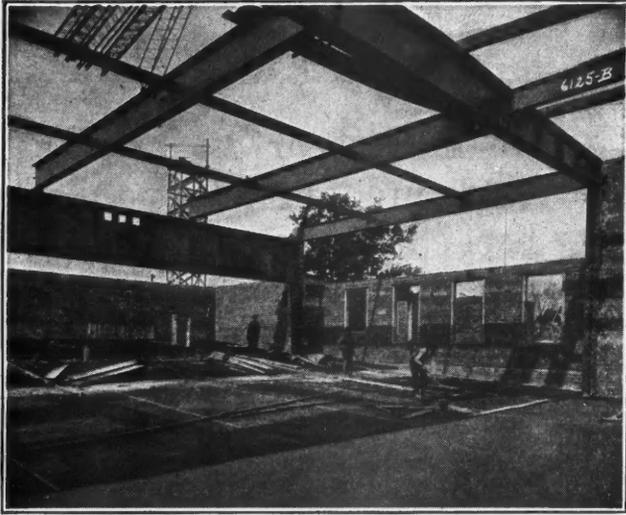
School Building, New Lexington, Ohio, Built with Massillon Bar Joist Fireproof Floors. View Shows Pouring Concrete Slab.
