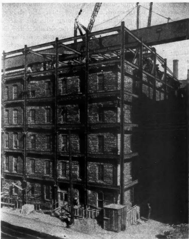
The Old Building Completely Encased by the Steel Frame of the New Building Which Was One Story Higher and Slightly Larger in Width and Length.
