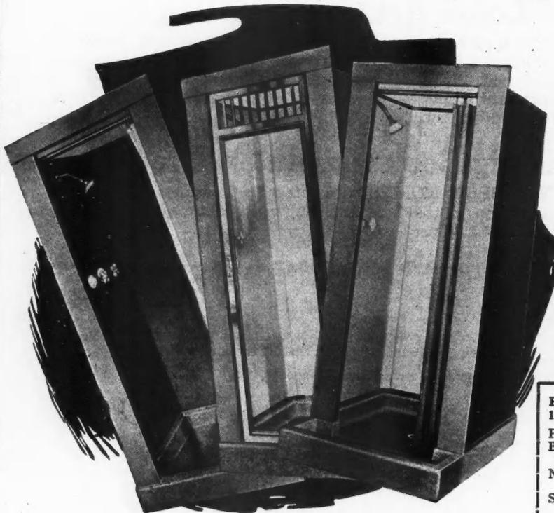
No matter how expensive or inexpensive the Bathroom may be, Fiat Showers make the ideal installations. Their knocked-down construction permits of ease in handling and quickness and simplicity in assembling.
