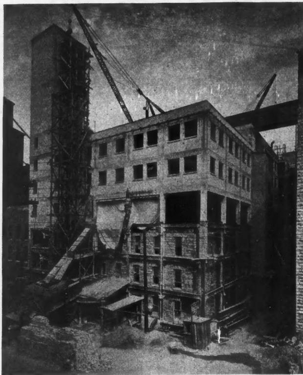
Here Is Shown the Progress of the Construction Work. Two stories of the new building have been completed, the machinery transferred to them and two stories of the old building demolished.
