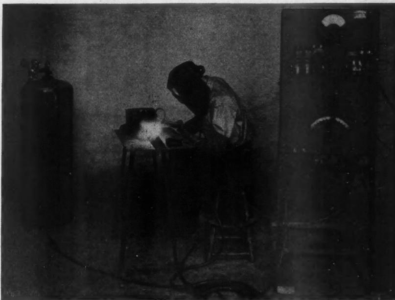
An Operator at Work with the New Atomic Hydrogen Welding Equipment Which Opens Up Entirely New Fields for Electric Welding.
