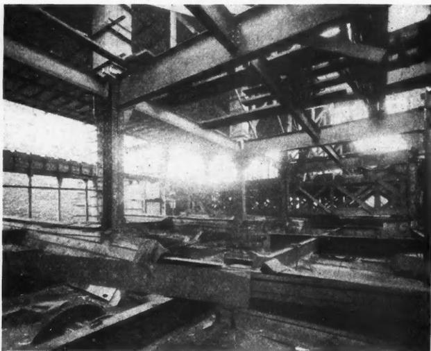
Temporary Wooden Trusses Were Placed on the Outer Walls of the Old Building to Support the Construction Equipment Until the New Steel Frame Was in Place.
