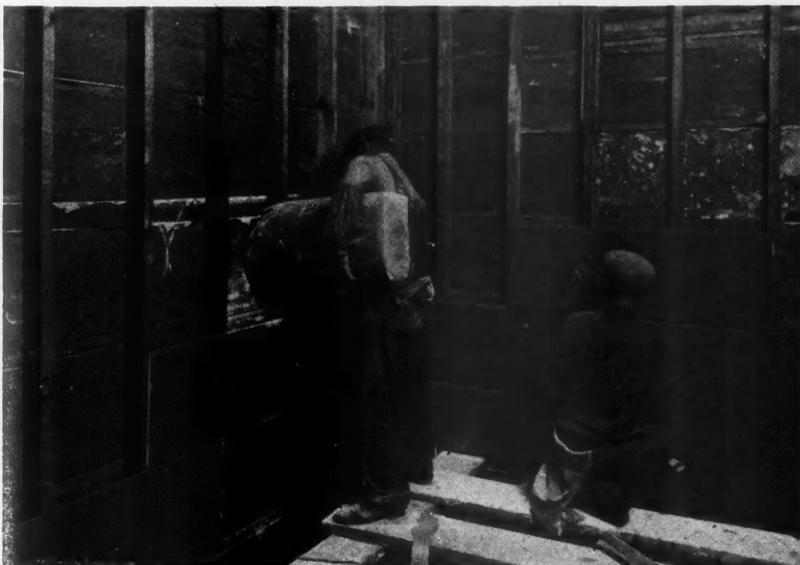
**The Walls of All the Buildings in This Development Are Thoroughly Insulated as Shown Here by Pouring a Gypsum Insulating Material Between the Studs.**
