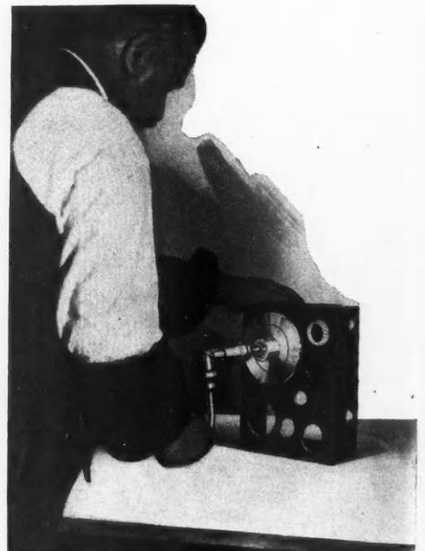
Round Holes May Be Cut in Wood, Steel, Sheet Metal and Other Materials in Minimum Time with This Hack Saw.
