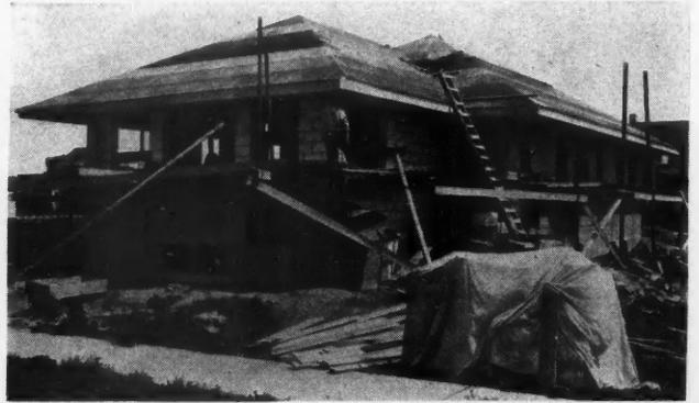
**The House Under Construction Here Is Being Built of a New, Hollow, Load Bearing, Gypsum Tile.**
