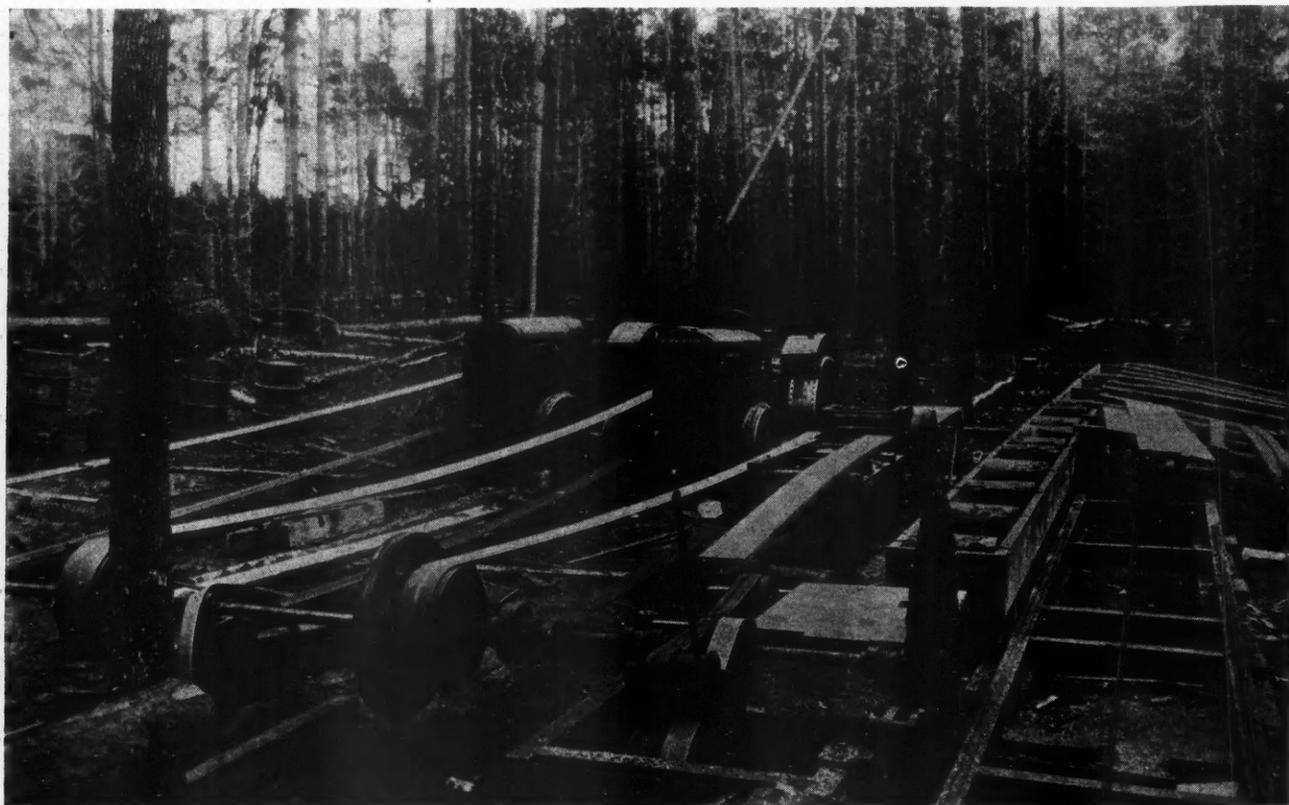
A Portable Sawmill Operated by Two Tractors in East Texas. When one tractor is used the output is from 10,000 to 15,000 feet per day. The extra tractor enables the operator to double his output and may be used, whenever necessary, for miscellaneous hauling, skidding logs and for road work.
