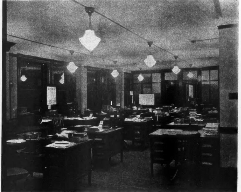
An Office Well Lighted by the Installation of 200-Watt Lamps Giving 2.35 Watts Per Square Foot and an Illumination of 11.6 Foot Candles:
