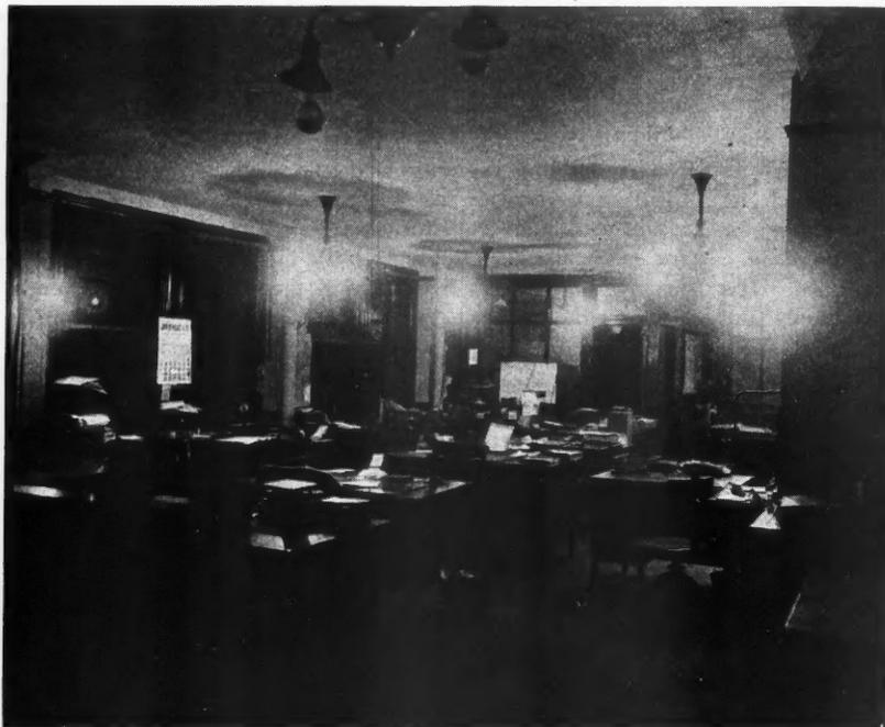
The Same Office as Shown Above Before the Installation Described; 100-Watt Lamps in Shallow Opal Glass Reflectors Giving 1.1 Watts Per Square Foot and an Illumination of 2.8 Foot Candles.
