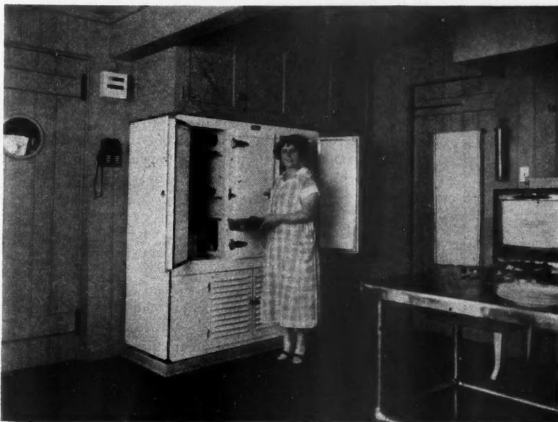
Here Is a Somewhat Larger Model Electric Refrigerator with Three Separate Storage Compartments. Enough of this kitchen can be seen to show that it is quite modern and well equipped. Some cases are built around this refrigerator but there are others which do not show in the picture.
