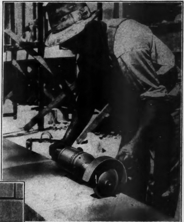
Cutting Random Ashlar strips to required length. Quick and easy because this electric carborundum saw is used instead of old mallet and chisel.
