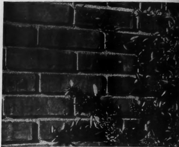
Note the Play of Shadows in This Deeply Raked Joint. Darrah Corbet, owner; A. L. Loveless, architect, Seattle.
