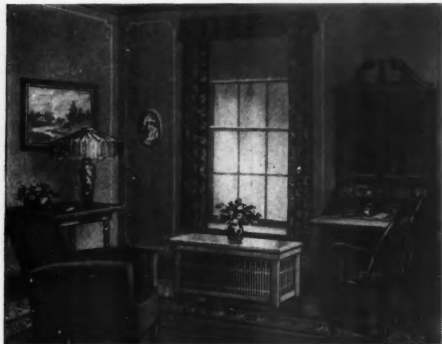
These Radiator Cabinets Greatly Improve the Appearance of the Room and Also Humidify the Air.
