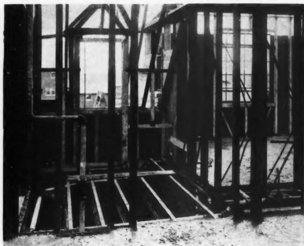
Partition Studs Are Steel. Note how the piping runs through the expanded steel floor joists without cutting.
