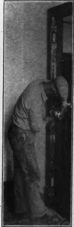
Hinge Butt Router and Templet on Jamb
