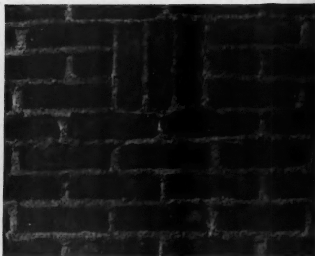
A Variety of Reds in a Pressed Joint with Natural Mortar. J. J. Cromwell, architect and owner, Woodmere, L. I.
