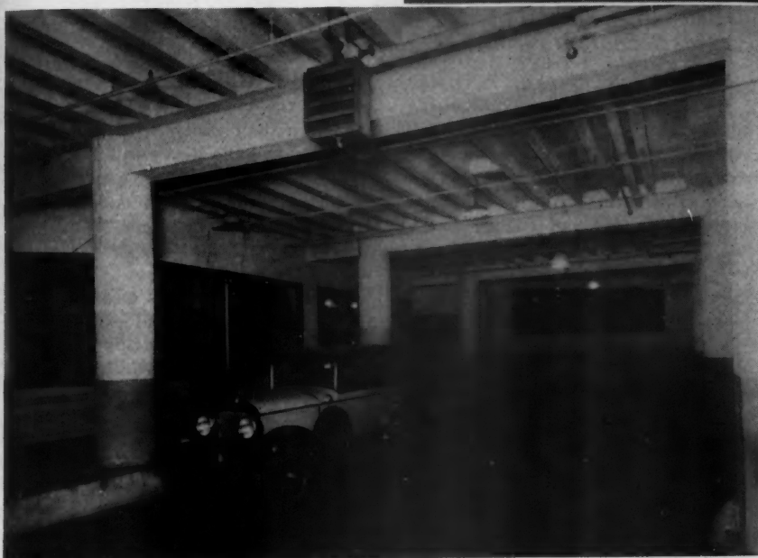
Entrance Driveway to the Baker Garage Showing Office Where Cars Are Checked In and Out, Also Doorway to "Foot Entrance." One of the unit heaters which heats the building shows in the immediate foreground.
