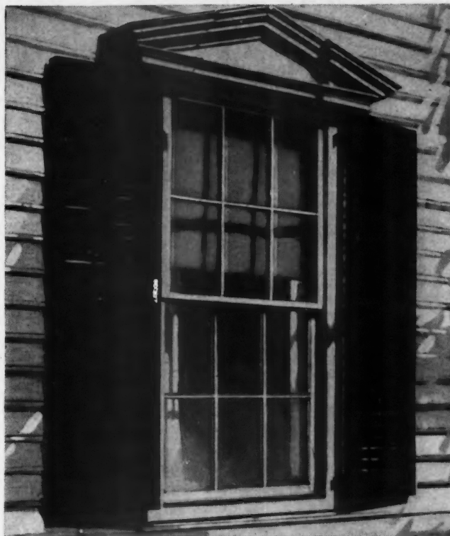
Pine moulding detail of a first story window of the Governor Wolcott House built at Litchfield, Conn. in 1753. The mitered break was a favorite device of early American woodworkers.
