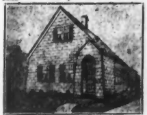
Photo by Lane Lumber Company. With the front porch removed, the exterior was covered with a new roof, dormer windows and a new porch. The upstairs was made lighter and well ventilated.
