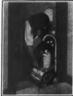
Sanding Door Openings
