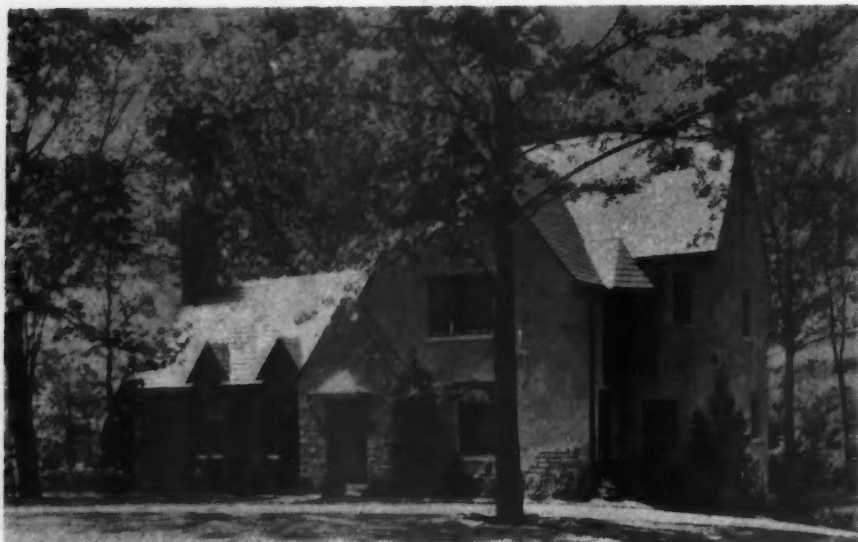
At Louisville, Ky., Local Stone, Stucco and Brick Were Combined in Pleasing English Adaptation to Produce the Louisville Courier-Journal Model Home Which Had a Built-In Garage at the Rear of Two Bathrooms.
