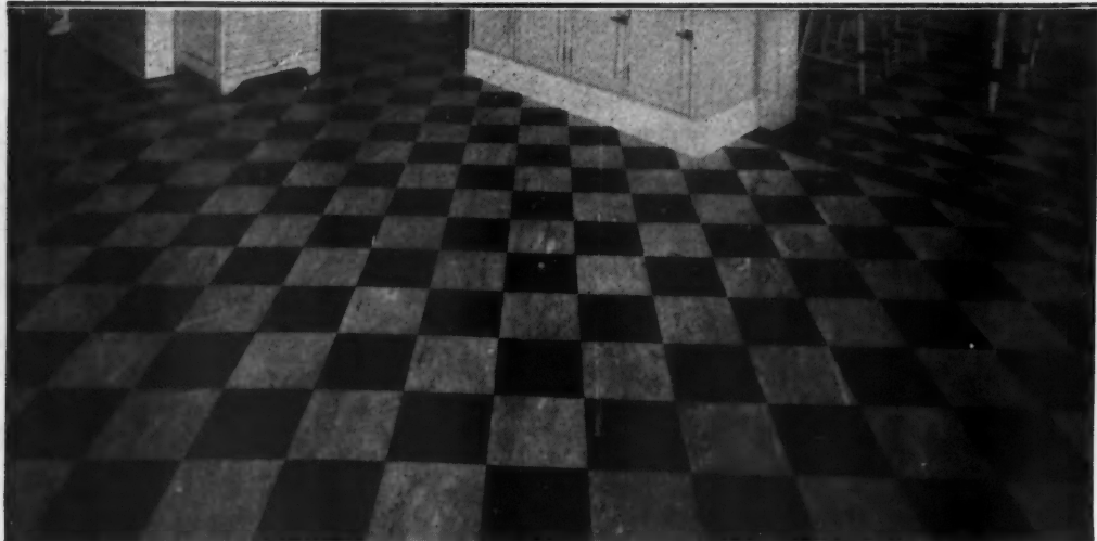
Lamson Floor Company made this fine installation of Goodyear Rubber Tiling in the kitchen, service dining room, butler's pantry and service hallways of the Studor Thompson residence, Cleveland, Ohio
