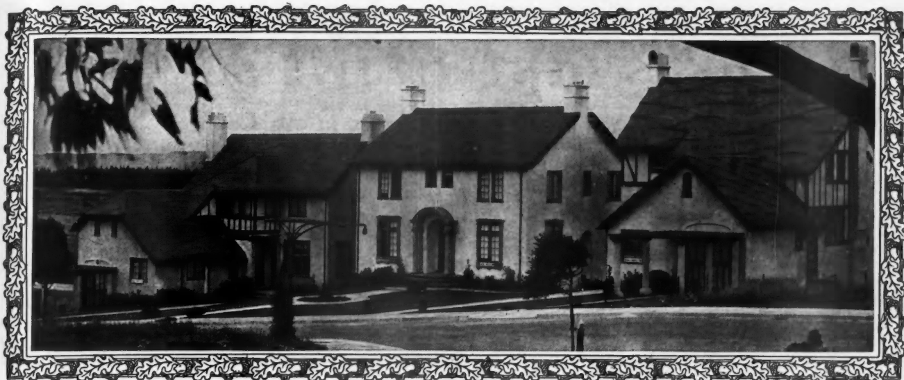
Leonard & Holt homes in Ingleside Terraces, San Francisco, floored with Oak
