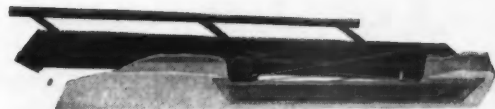
When flush with the ceiling, the panel of the stairway makes a pleasing appearance. It may be finished to match the other woodwork in the room.
