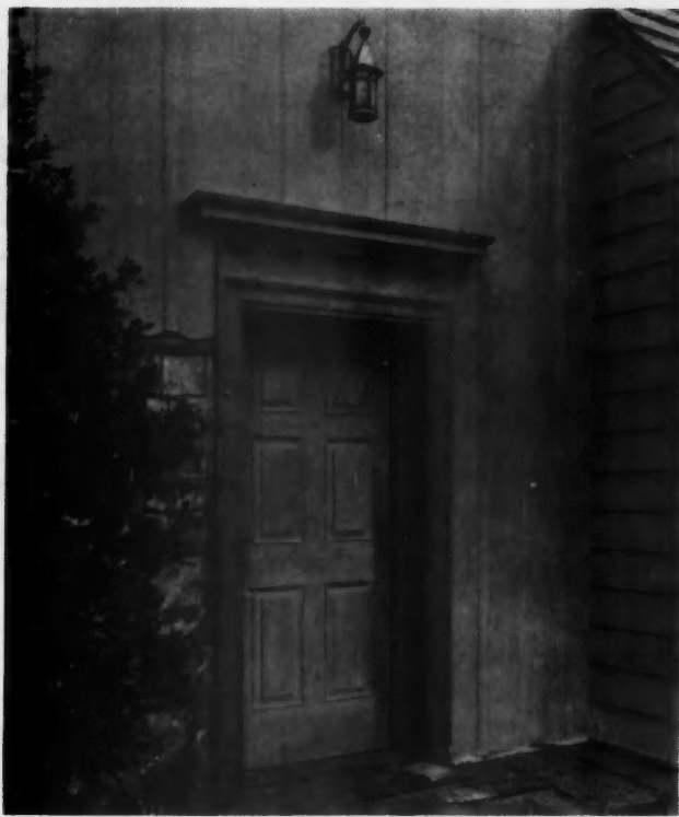
The Vertical Siding in the West Coast Woods Prize Home Is of Western Red Cedar, the Horizontal Siding of Sitka Spruce, the Door of Western Red Cedar Outside and Douglas Fir Inside.
