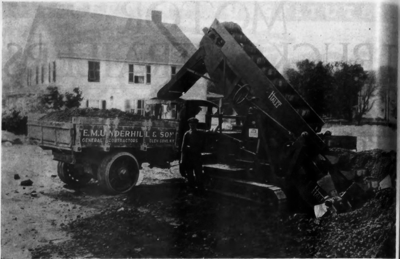
The Tires and Wheels of the Truck Must Take Up a Large Proportion of the Road Shock and Require Careful Attention, Especially Where Trucks Are Operated Under Rough Road Conditions, as Is so Often the Case with a Contractor's Equipment.
