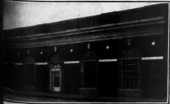
Fenestra windows give an individual character to the exclusive shop, store or office.
