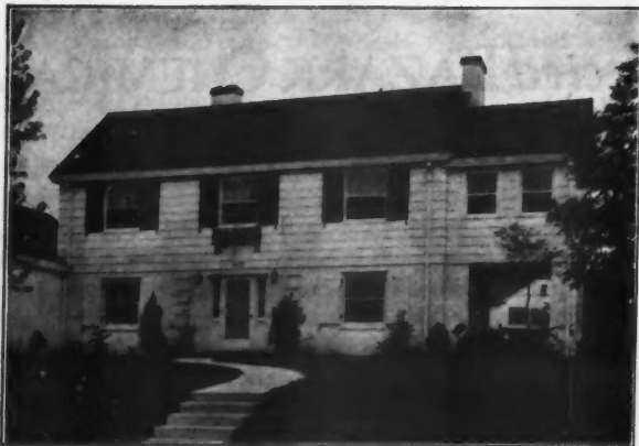
Residence of R. O. Smith, Kansas City, Mo., Edward Buehler Delk, Architect, Exterior Trim finished with Cabot's Double White and Green Collopakes, Exterior Walls finished with Cabot's Old Virginia White Collopakes, Roof of Cabot's Creosote Stained Shingles. Walls and 2nd floor insulated with Cabot's XX and XXX Quilts.
