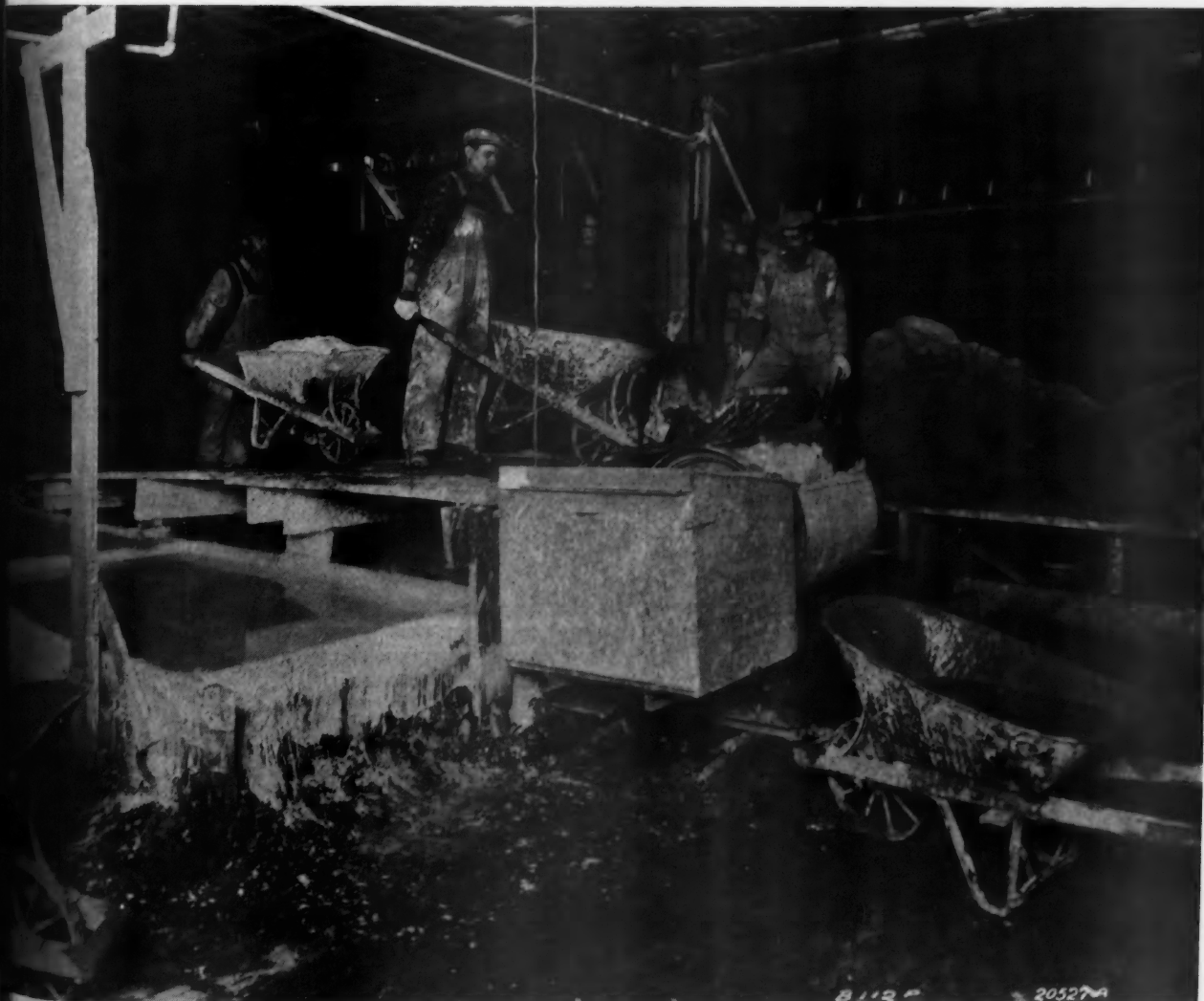
Loading Platform Built to a Level with the Top of the Mixer Greatly Facilitated Loading on the Pittsfield Building Job.
