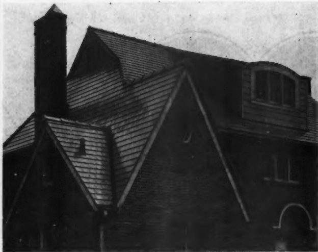
Home on Balfour Road, Detroit, Three Years Old, Showing the Adaptability of Glass Coated Armco Iron Shingles to the Various Angles of Hips, Ridges and Valleys.
