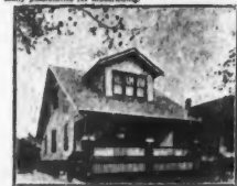
Photo by Lane Lumber Company. This is the same house after remodeling. The outside walls were a new roof, dormer windows and a new porch. The upstairs was made lighter and well ventilated.
