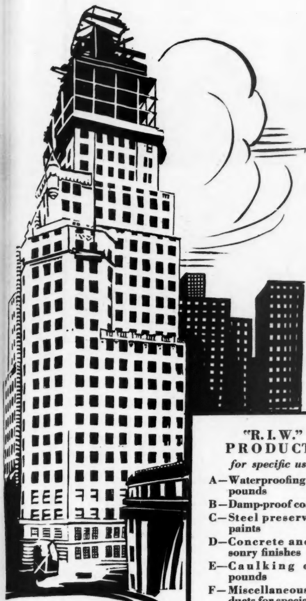
The International Telephone Building New York City Buchman & Kahn, Architects Louis S. Weeks, Consulting Architects A. E. Lefcourt, Builders Toch's R. I. W. Semi-Mastic and Mastic, Damp-proofing and Plaster Bond used on the above structure.
