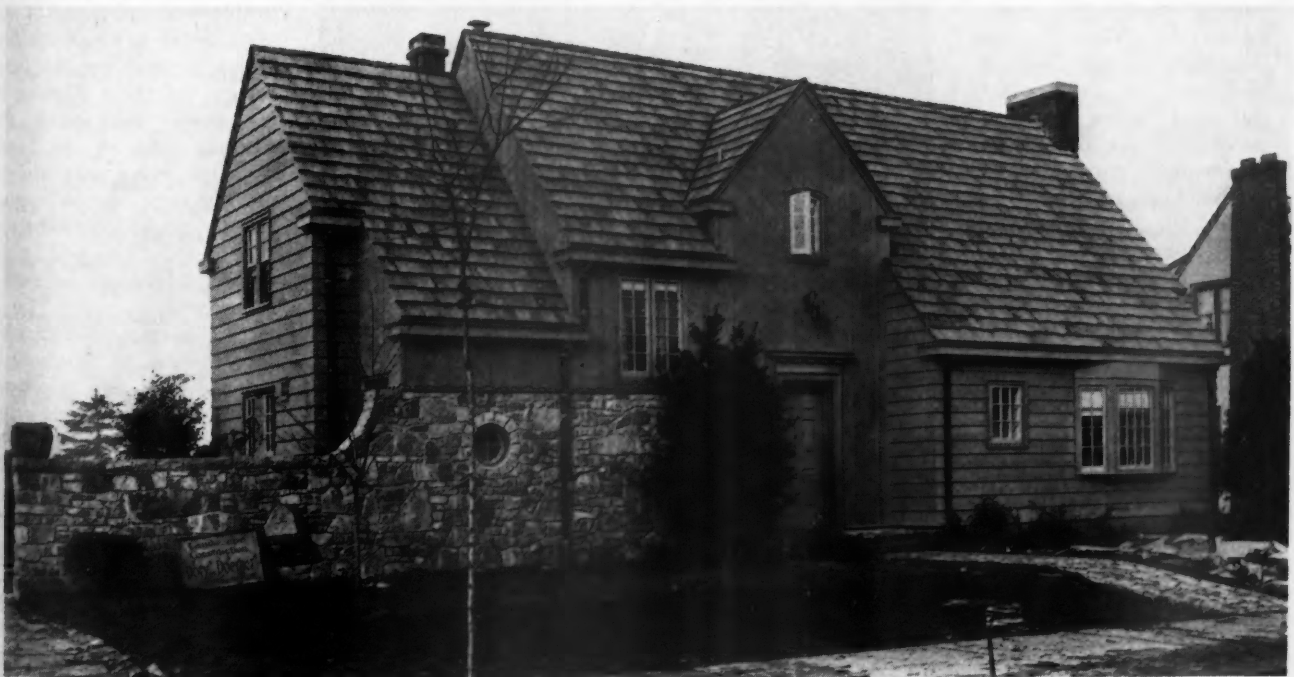
This Charming Home Was Built in Portland, Ore., from the Plans of Otho McCrackin, Hutchinson, Kansas, Which Were Awarded the First Prize of $2,000 in the West Coast Woods Architectural Competition. Four of the major commercial woods of the West Coast were used in its construction; Douglas fir, West Coast hemlock, Western red cedar and Sitka spruce.
