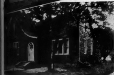
Modernized home of Mr. Madison Gilbert, Owosso, Mich. Shingles for sidewalls cost $145.35. Other remodeling cost $920. Entire labor $155.05. Increased valuation—over $2,000.
