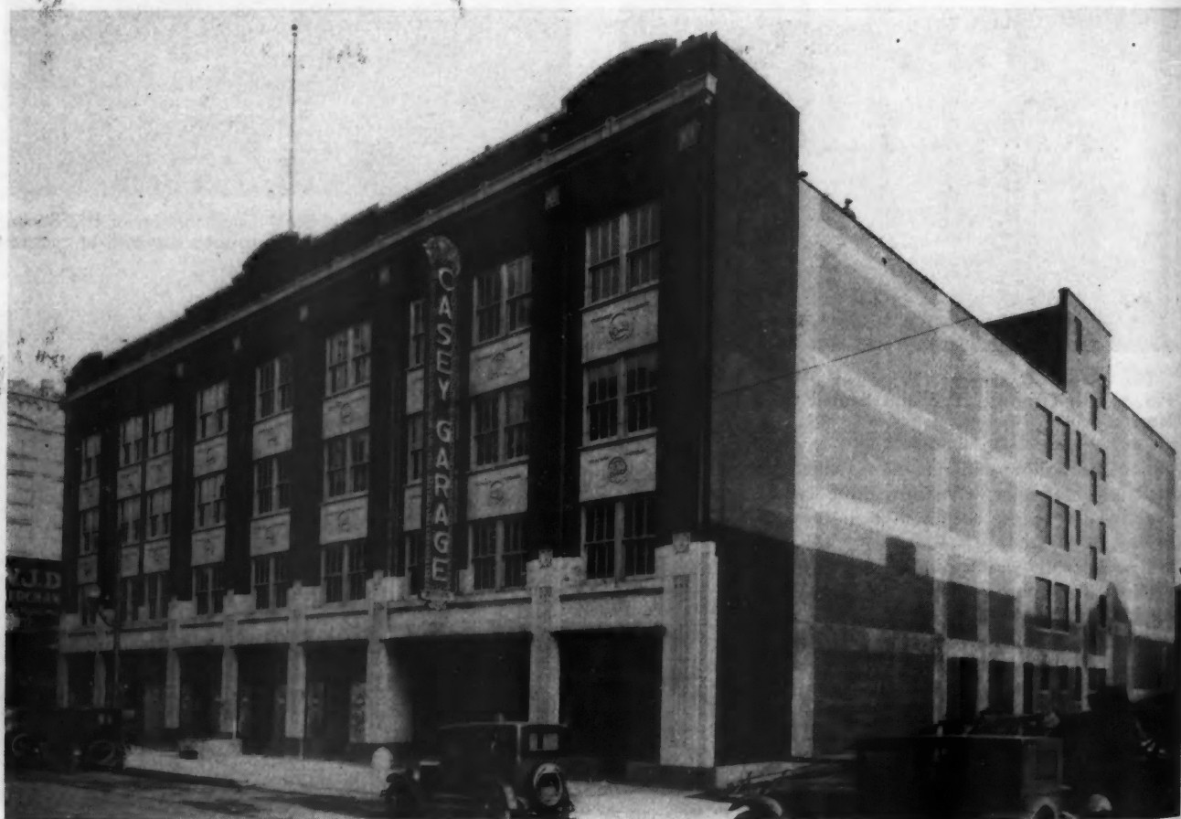
Built for Extension by Additional Floors. This Most Completely Equipped Garage at Scranton, Pennsylvania, Will Ultimately Have Capacity for 1,000 Cars. Columns go down 58 feet to bed rock and considerable coal was taken out of the excavations.
