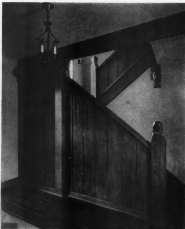
This Balustrade Is of Vertical Grain, West Coast Hemlock with Sand Etched Decorations. Port Orford cedar was used for the carved posts and the floor is of Douglas fir made from finished boards rounded on the edge.
