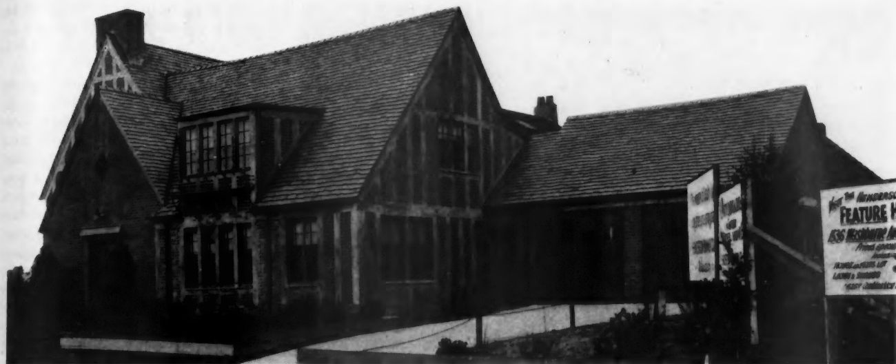
This Brick and Half-Timber Model Home Sponsored by the Portland Oregonian Contained Seven Rooms, Two Baths and an Attached Two-Car Garage.
