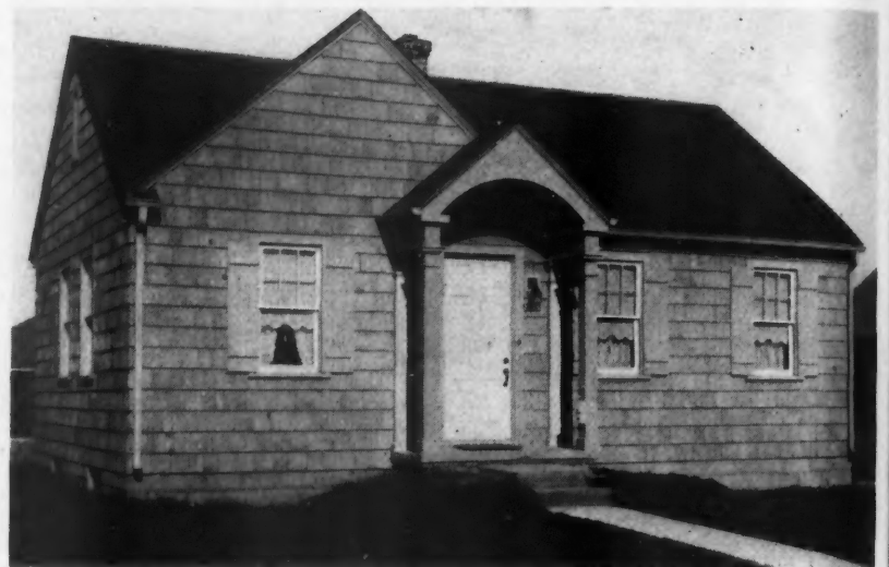
Here Is One of the Small House Series of Designs Which Roth Brothers, Inc., Is Prepared to Build on Short Notice. It is listed as design No. 2804.
