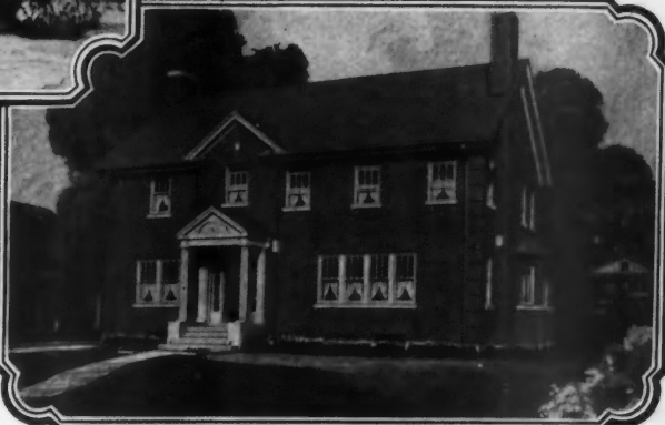
Residence of John A. Saerman, 9927 S. Robey St., Chicago. This also has Masonite Insulating Lath as a plaster base. Architect, Bert Hubbard. Contractor, Geo. A. Nordgren
