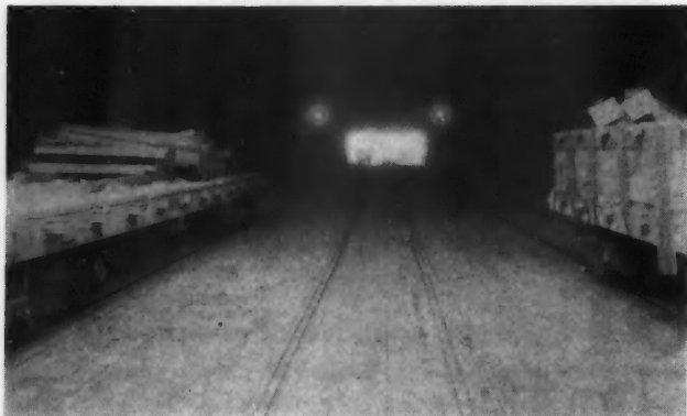
The New Plant of the Seaboard Refrigerating Co., Jersey City, N. J., in Which Treated Lumber Was Used.
