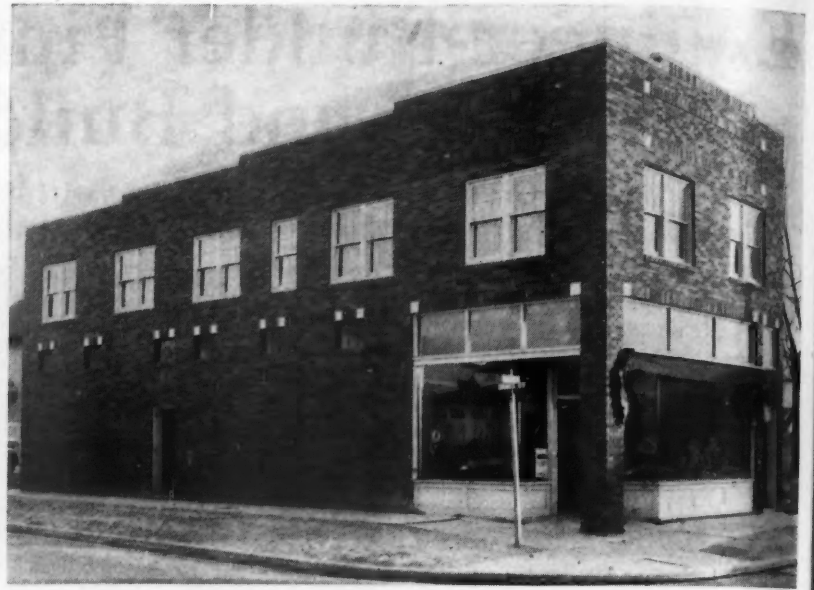
Store and Apartment Building Erected in Flint by the Wade Hampton Horn Company. This building was finished last summer and has a small basement, steam heat, refrigeration, wood floor joists and studs on second floor. It contains two suites of apartments and one store room.
