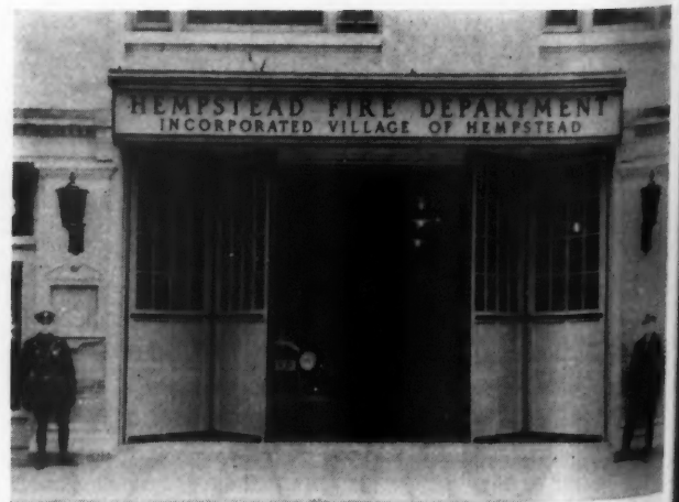
These Doors Are of a Quick Acting Type Which Has Been Found Particularly Suitable for Fire Stations.
