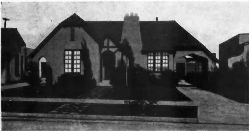
Some of the Types of Home Architecture Which Have Become Popular of Late Years, Lend Themselves Particularly Well to Treatment in Stucco.
