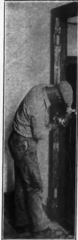
Hinge Butt Router and Templet on Jamb
