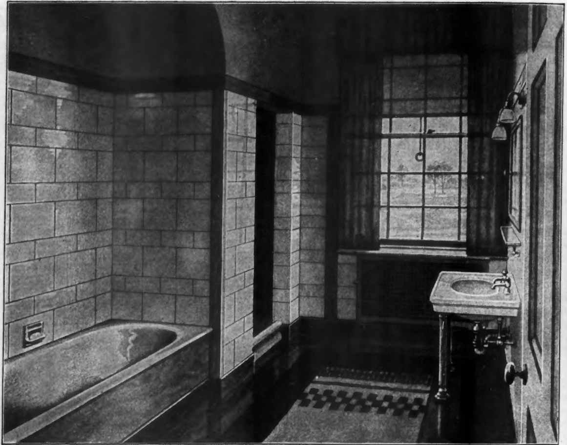
One of Several Bathrooms in the Residence of Mr. Marshall Field, Lloyd's Neck, Huntington, Long Island. John Russell Pope, Architect
