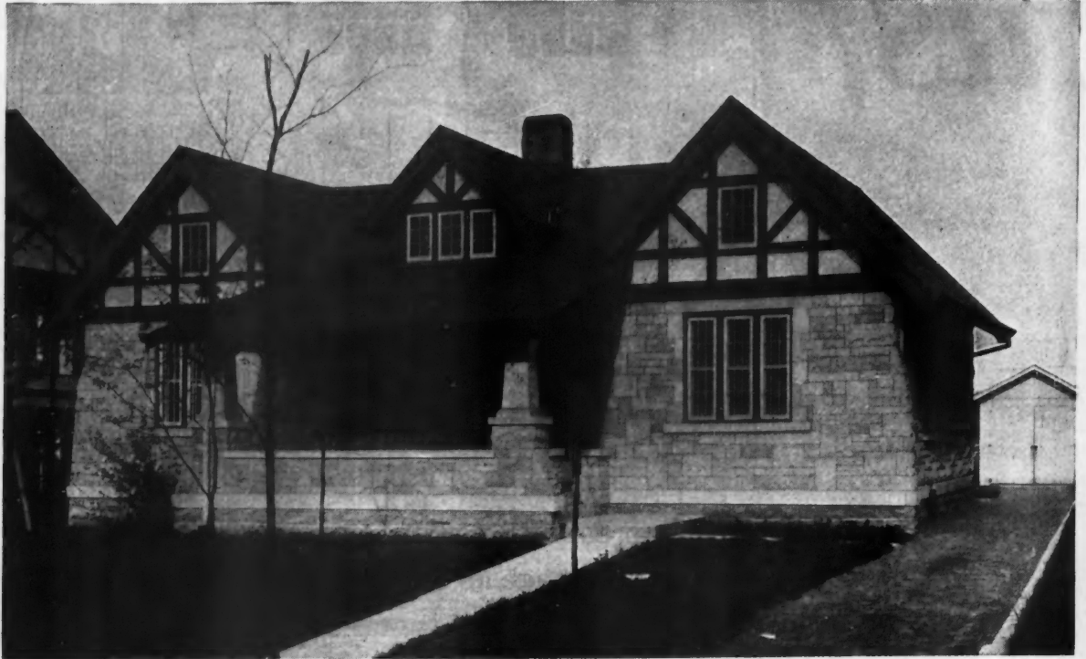
English style bungalow, five rooms and bath. Ordinary wood stud-frame construction faced with veneer of Indiana Limestone laid up as rock-face Random Ashlar.
