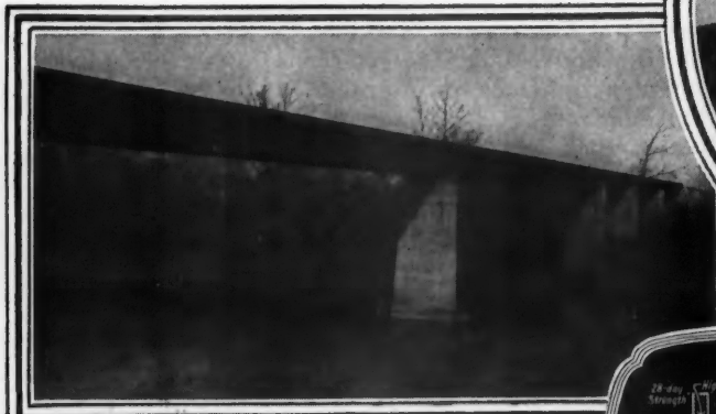
Periodic rises of the Vermilion River made it necessary to increase the height of the bridge of the Streator, Ill., Drain Tile Co. Both early use of the improvement and permanently stronger concrete resulted from use of High-Early-Strength Universal Concrete .
