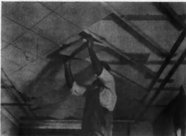
These Tile Are Attached to the Ceiling by Inserting in Metal Tee Stripes Which Lock Them Rigidly in Place.
