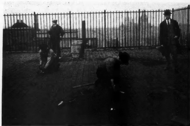
The Next Step Was To Caulk the Cracks Between the Tile With a New Asphalt Compound Which Is Quickly and Easily Applied.
