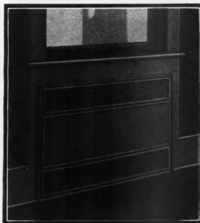
The front of the unit, including grilles, is a one-piece panel, furnished complete. Slips on and off in a moment—provides immediate access to the unit at any time.
