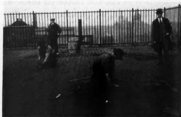
The Next Step Was To Caulk the Cracks Between the Tile With a New Asphalt Compound Which Is Quickly and Easily Applied.
