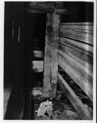
Fig. 9—A Post in a Retail Lumber Shed Thoroughly Infected with Dry-Rot and Showing Fruit Bodies of Pora Incrassata Running to the Top. Infection will be transmitted, in the course of a few days, to the sound stock piled against it.
