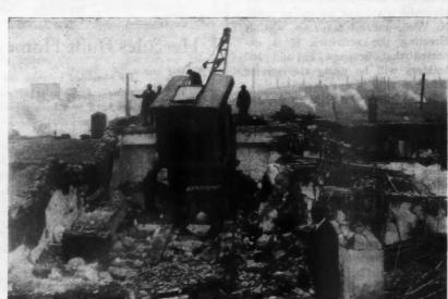
Here the Crane Is Being Lowered from One Floor to Another on Two 12 by 12-Inch, 20-Foot Timbers. One winch truck below is doing the lowering. Conrad Lurie, the contractor handling the job, is standing in the foreground.
