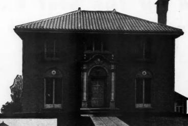
An unusual type of bung low with cement stucco walk Sheet steel roof with standin seams.
