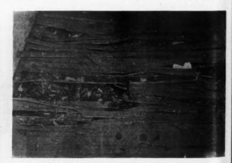
Fig. 3—Dry-Rotted Pine Floor Laid Over Brick. A new floor would not last more than a year or two unless treated with a wood preservative.
