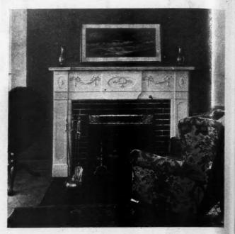
A Fireplace, Equipped with the Heater Described Here, Has a Neat Grill Above the Opening, from Which the Heated Air Comes Into the Room.
