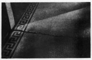
Fig. 2—Tile Surfaced Porch Floor, Showing a Large Crack in the Tile, Due to the Rotting Out of the Form Lumber Left in Position Beneath.
