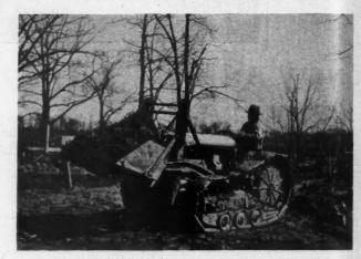
This Crawler Power Shovel Is One of Two New Machines Recently Placed on the Market, the Other Being a High Lift Loader.
