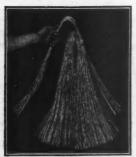
Steelcrete Lathers Tie Wire Here is a Tie Wire designed for the Lather. A product of un-usual strength, yet soft and pli-able for quick and efficient workmanship. Wrapped in sanitary packages, a safeguard tothe Lather like sterilized nails. Supplied in hanks 25 lbs. each.
