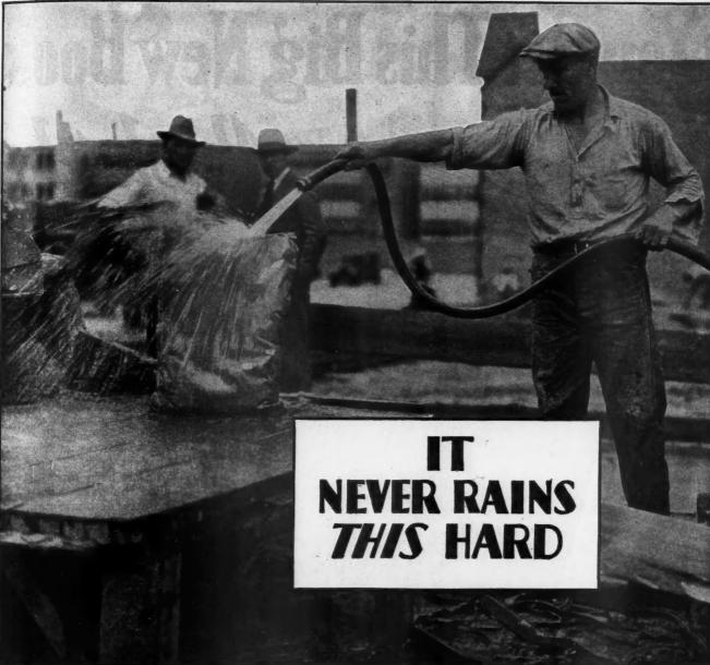
THE man with the hose gave this cement-filled Bates Multi-Wall Paper Bag a test far more severe than weather could give it. Yet, even after continued soaking under the heavy hose stream, this bag, chosen at random from
