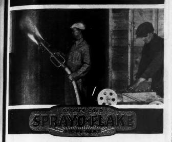
SPRAYO-FLAKE is creating a sensation. Architects, builders and homeowners, everywhere, are interested in this efficient, low-cost insulation sprayed on with guns. Now, for the first time, it makes available a tight-sealing insulation that penetrates every nook and crevice, seals every opening, covers around pipes and window jambs—blankets every space perfectly.
