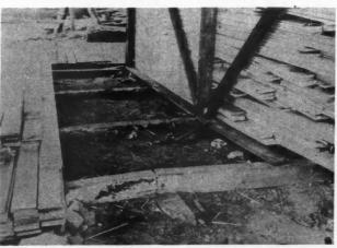
Fig. 10—The Dry-Rot Fungus, Poria Incrassata, in the Foundations and Running Up the Post of an Open Shed in Southern Alabama.
