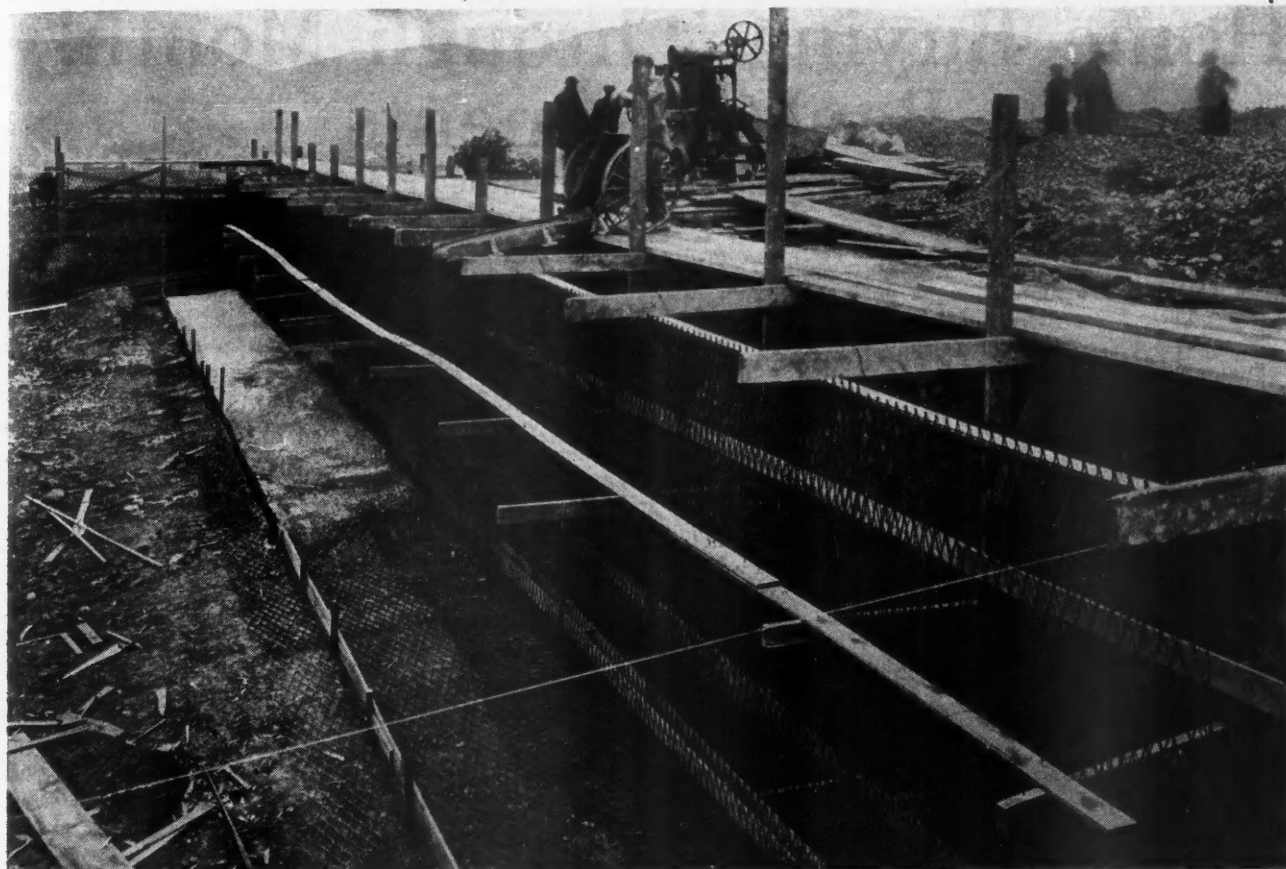
Fig. 5. When Used for Pool and Reservoir Wall Reinforcement, Expanded Metal Is Found Convenient to Place and Remains in the Proper Position After It Has Been Correctly Placed.
