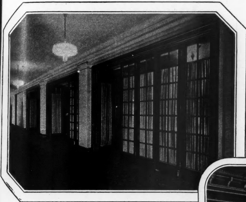
FoldeR-Way illustrated here is particularly suitable for doors of medium weight. Doors are carried by ball-bearing hanger running in overhead track.
