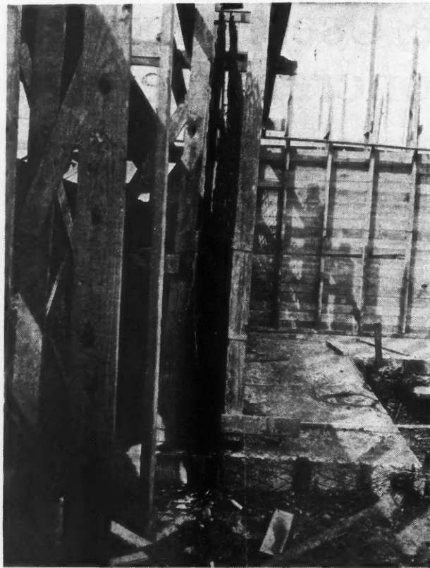
Fig. 3. Expanded Metal Has Proved Adaptable to the Reinforcing of Concrete Walls of Swimming Pools and Reservoirs.
