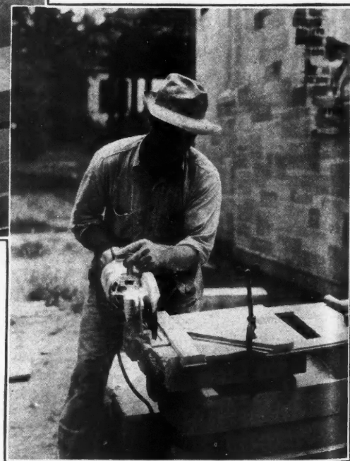
(Right) This man is using portable electric carborundum saw for cutting the groove across the stone. Little more than a scratch is necessary and an ordinary hand saw or buck saw can be used if preferred.
