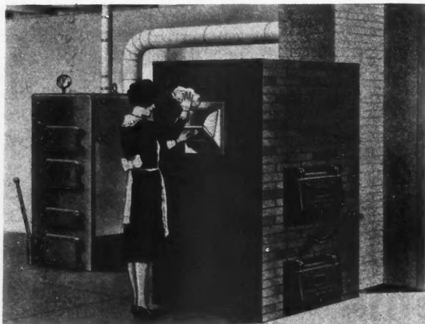
An Incinerator of Well Known Make Which Has Now Been Adapted to Basement Feed for Houses Already Built.
