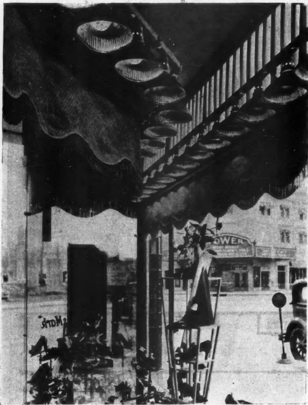
Show Window Lighting Equipment Used for the First Floor Shops in the McClatchey Building.
