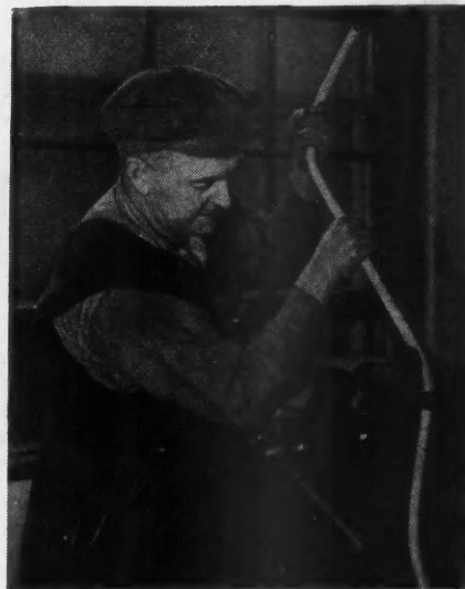
Workability and Elimination of Thread Cutting Make This Metallic, Electric Tubing Economical.
