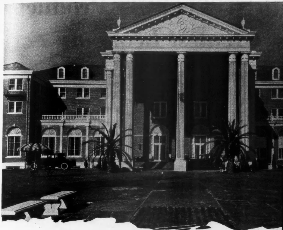
Hotel Biloxi, Biloxi, Mississippi. Architects, Federal Engineering Co. Associate Architect, H. S. Muesse. Eleven Union Metal Columns No. 213, 38' 6" in height with two pilasters to match used on the entrance. In addition half and quarter round columns 16' 11" in height of the same design were supplied.
