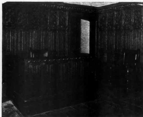
Asbestos and Cement Have Been Moulded Into Panels Which Give, at Low Cost, a Remarkable Reproduction of Hand Carved Wood Paneling.
