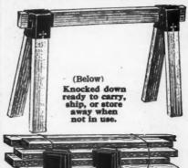
Quickly assembled or taken apart. Easily carried from job to job. Hold 8600 lbs. without a creak. No nails or braces.
