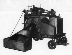
Powered with a 4-cylinder, 12 H. P. gasoline engine. 8 seconds to elevate skip from ground and 15 seconds to empty. Automatic clutch knockout bar holds skip in charging position. Operating levers arranged on drum end, making effective one-man control.
