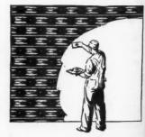
One Sheet of Arch Lath (28 x 96) grips the plaster at 8064 points; making the wall an integral unit of rigidity and strength, while minimizing possibility of cracking
