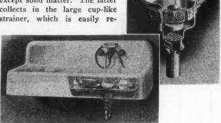
A Sink Equipped with This New Strainer and an Enlarged View of the Strainer Itself.
