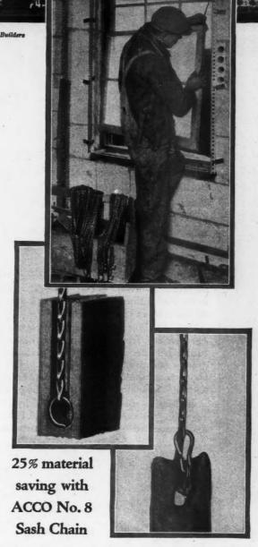
Tying knots wastes from 4 to 5 feet of cord per window. 100 feet of Acco No. 8 Sash Chain will hang 2 more windows.
