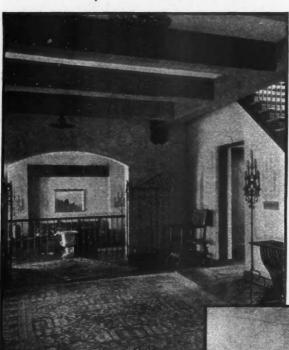
The concrete floor protects the furnishings of this living room from damage by basement fires.
