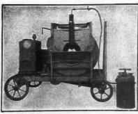
Concrete Heater Attacher a Mixer in Operation, Ass Smooth, Even, Strong Work. Attached Assuring
