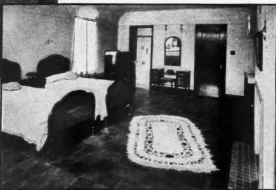
In this bedroom, the concrete floor is overlaid with cork floor tile. There will never be any creaking floor here!
