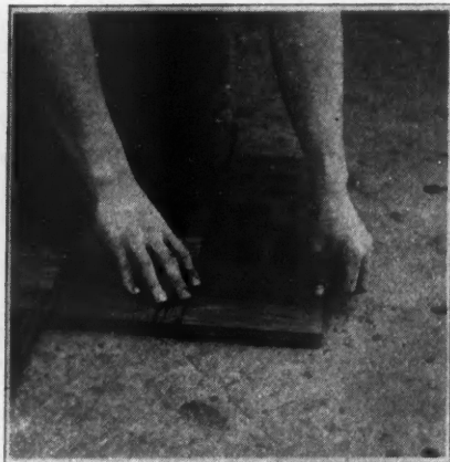
The Final Steps in the Process of Laying Wood Block Flooring. This is so simple and rapid that labor cost is materially reduced, bringing parquet flooring within the range of any flooring estimate.
