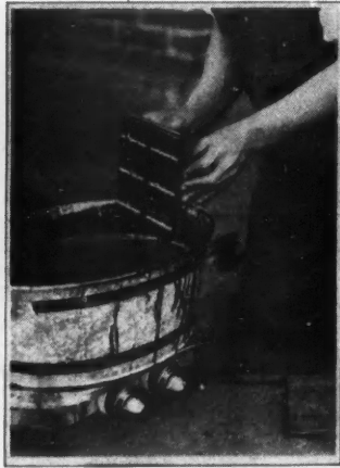
Here Are Four Views Showing the Successive Steps in Laying Treated Blocks in Mastic, Over Concrete or Wood Sub Floors. See three views at bottom of page 72 for continuation of this process.
