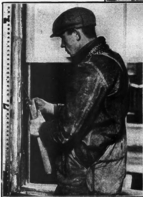
The chain is hooked to the weight. Both ends are thus anchored securely with no possibility of the connections loosening or breaking.
