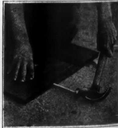
The Final Steps in the Process of Laying Wood Block Flooring. This is so simple and rapid that labor cost is materially reduced, bringing parquet flooring within the range of any flooring estimate.
