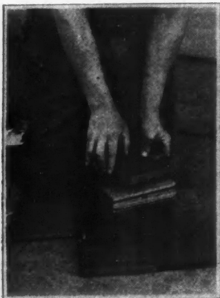
Here Are Four Views Showing the Successive Steps in Laying Treated Blocks in Mastic, Over Concrete or Wood Sub Floors. See three views at bottom of page 72 for continuation of this process.
