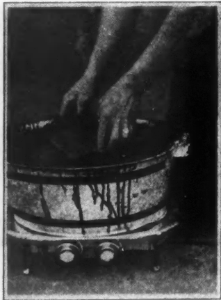
Here Are Four Views Showing the Successive Steps in Laying Treated Blocks in Mastic, Over Concrete or Wood Sub Floors. See three views at bottom of page 72 for continuation of this process.
