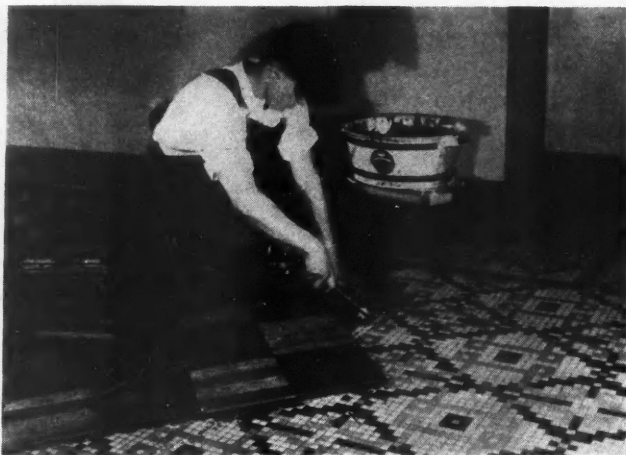
Laying Nine-Inch Treated Blocks in Mastic, Over an Expensive Mosaic Tile Floor in the Peabody Hotel, Memphis.
