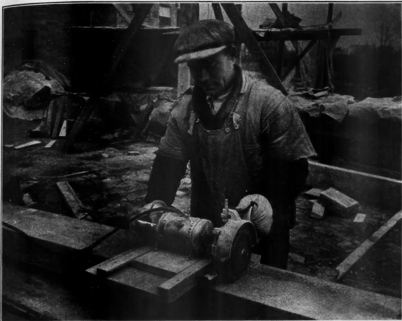
In breaking Indiana Limestone Random Ashlar, a shallow groove is made on one side of the stone strip by means of an electric portable saw or ordinary hand saw. The stone is then turned over and a tap with a mallet breaks it clean on a line with the groove.
