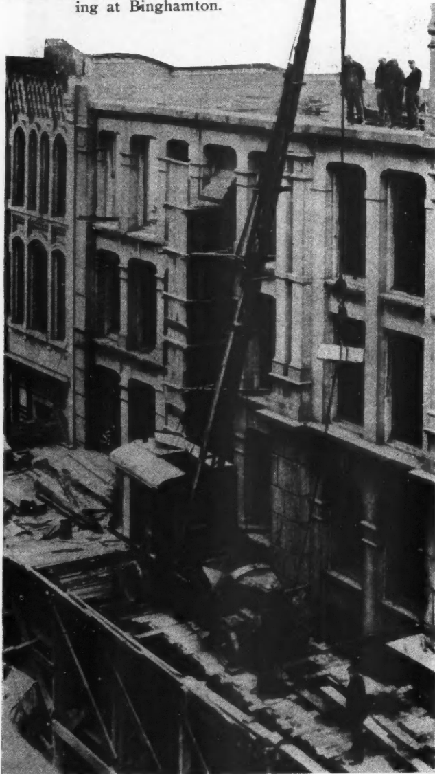
TRUCK CRANE on the Job, Taking Down the Old Six-Story Phelps Building at Binghamton.
