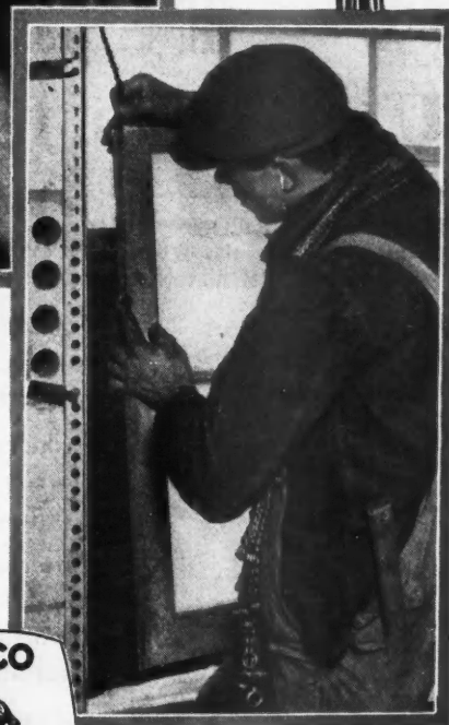
The above illustration shows how ACCO No. 8 Sash Chain is attached to the weight.
