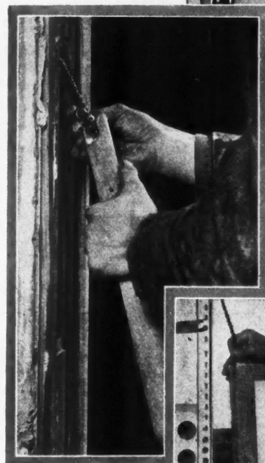
The above illustration shows how ACCO No. 8 Sash Chain is attached to the weight.
