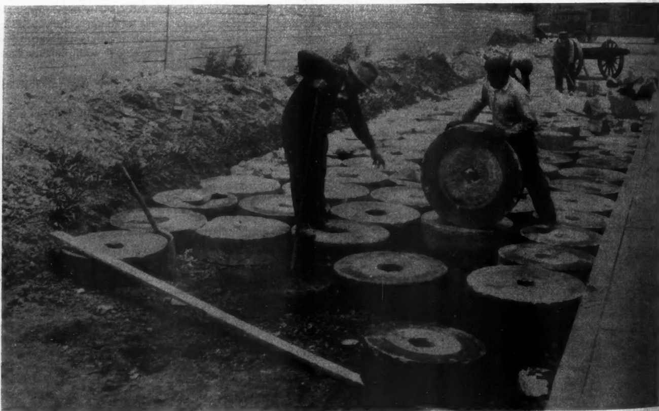
A GRINDSTONE ROAD Built of Stones Worn Down Making Hand Saws. The spaces between stones are filled with concrete. The road is standing up well under heavy truck traffic.
