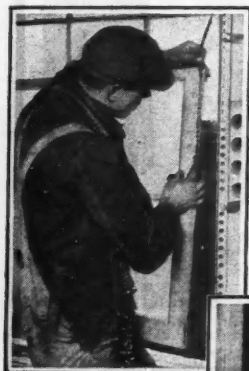
Sash is anchored with simple coil
