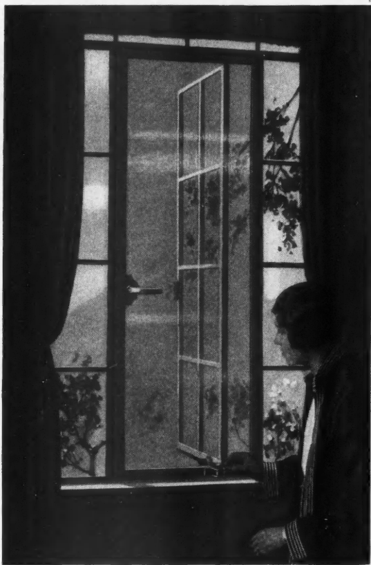
The swing leaf is opened or closed without touching the screen.
