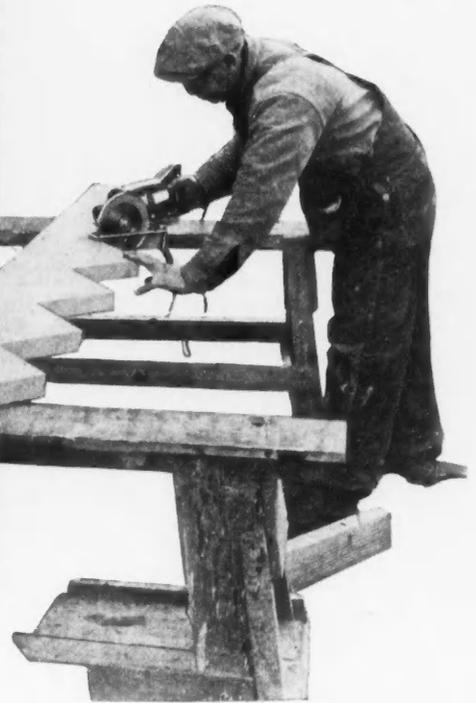
Below: With a Carborundum Disc, the Electric Hand Saw Is Efficient in Cutting Random Limestone Which Comes to the Job in Long Slabs.
