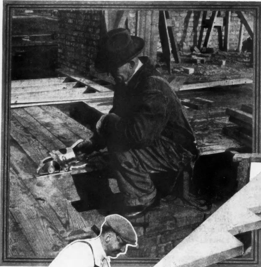
Left: The Electric Hand Saw Trims a  $\frac{1}{8}$ -Inch Rough Floor on a Large Apartment Job. Below: Stair Stringers are cut out in a fraction of the time required with an ordinary hand saw.
