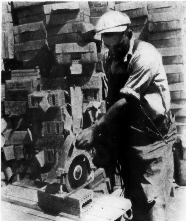
Cutting tile, brick, or stone with an electric saw is the only practical way. In addition to being many times as fast, the electric saw saves material and insures an accurate fit.
