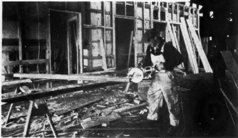
Electric hand saws are from 7 to 10 times as fast as "muscle" hand saws. They will rip a 2-inch pine plank 6 feet long in 30 seconds.
