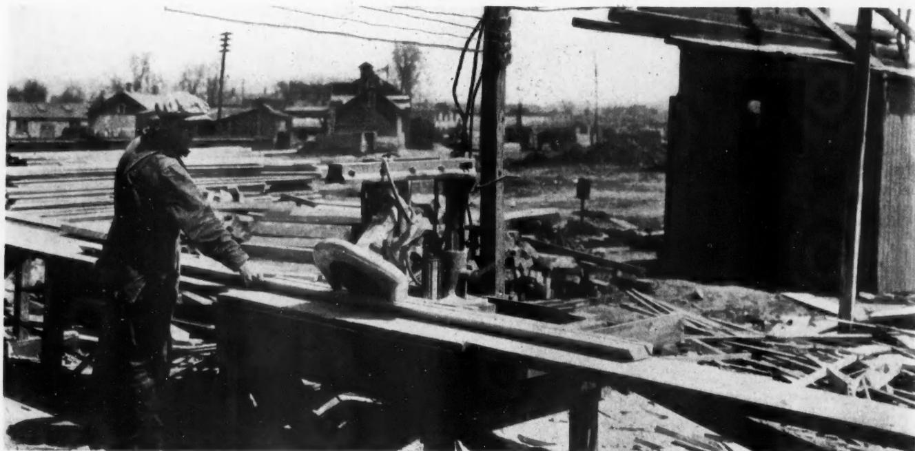
On concrete form work the power saw has reduced carpentry cost 50%. It is used to rip, cross-cut or bevel all columns, end beams, battens, stair-risers, wedges, shoring, spreaders, etc., and speeds up the entire job.
