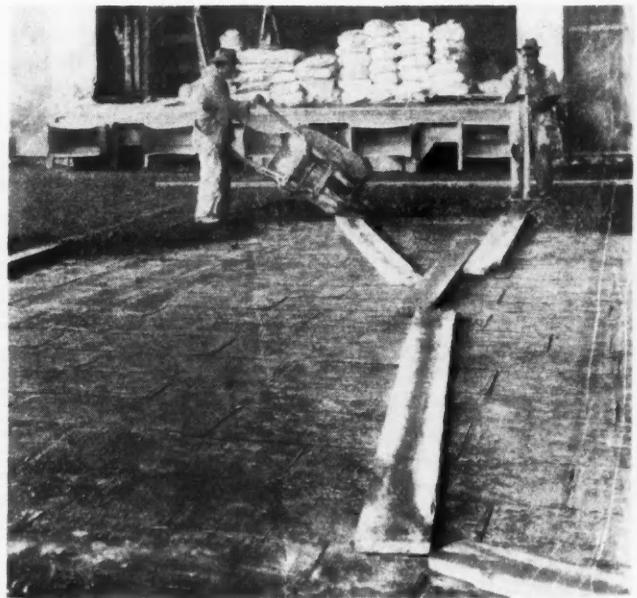
A Floor Over the Ground, or Over an Unheated Space, Requires Insulation Under the Concrete.
