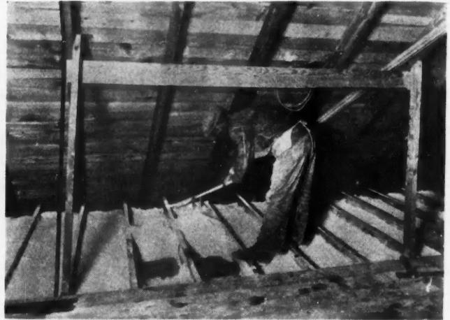
Gypsum Dry Fill Materials Are Poured Into the Wall Spaces or Between Floor Joists Filling the Entire Space.
