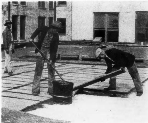
Two Layers of Fiber Board Insulation Covered with Prepared Roofing and Gravel Assure Conservation of Heat Below.
