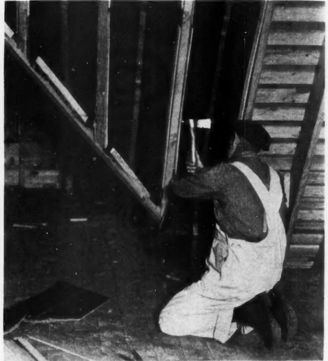
Flexible Blanket Materials Are Turned Up at the Edges and Nailed to Studs or Rafters.
