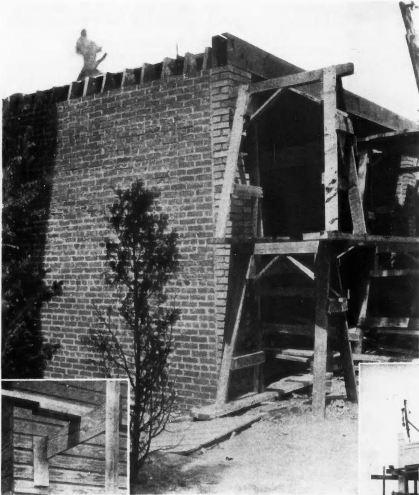
ERECTING HORSES on job at Pelham, N. Y., by Anthony Smith; note pin anchors. In insert—notched piece used for scaffold support by S. T. Briggs, Essex, Md.
