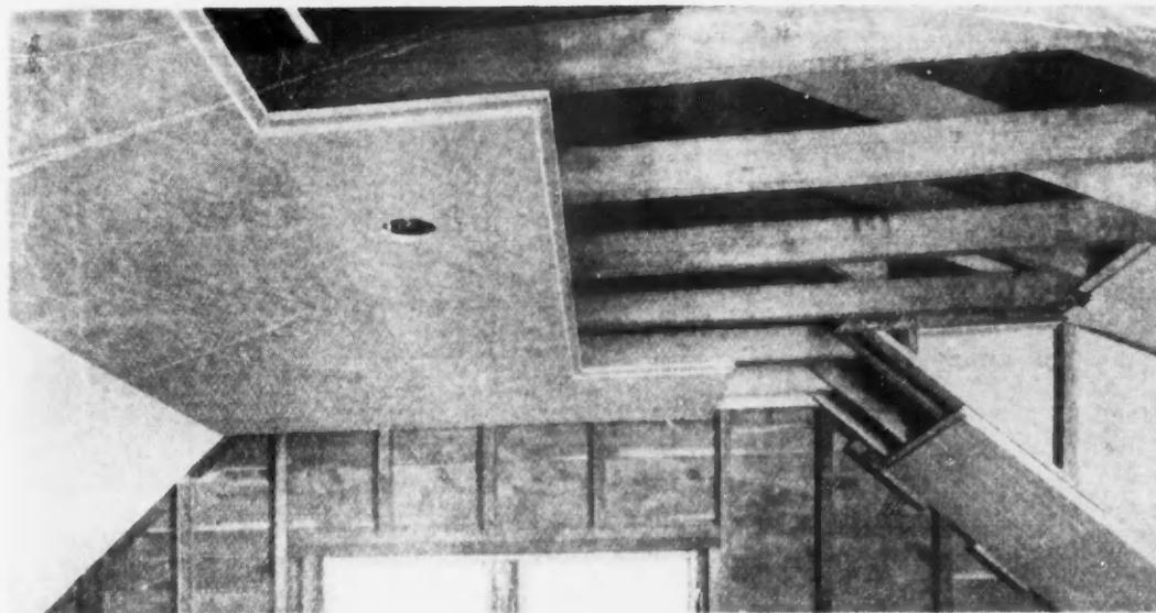
Many Manufacturers Are Now Offering Insulation in a Form Called Lath, as a Plaster Base. The Lath Comes in Small, Easily Handled Sizes, with Shiplapped Edges to Produce a Smooth Wall Surface.
