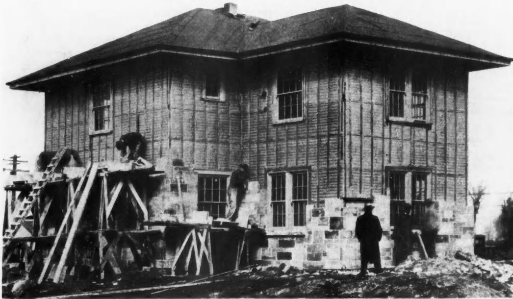
Placing Limestone Veneer over Walls of a House Completely Insulated with a Flexible Blanket Material to Produce a Home That Will Be Comfortable at All Times and Inexpensive to Heat.
