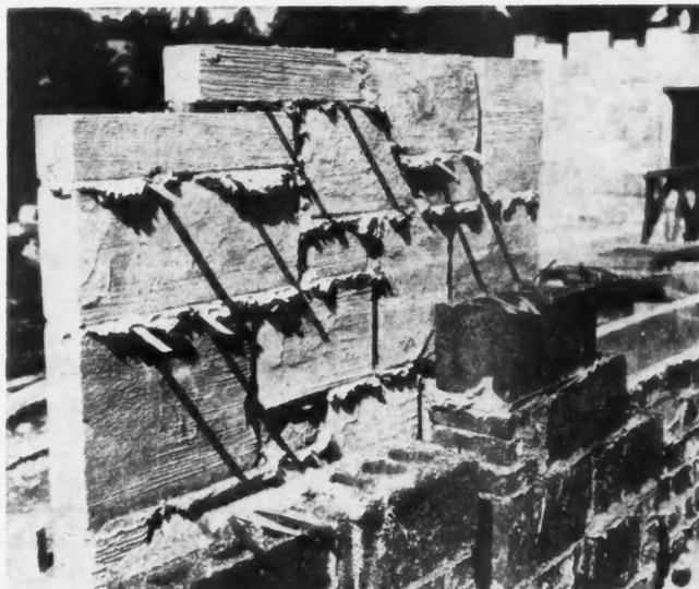
Four-Inch Limestone Veneer Tied to Cinder Block Backing with Metal Ties.
