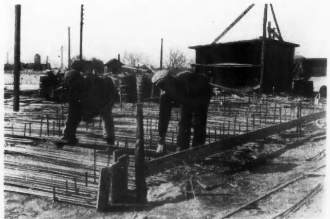
If Reinforcing Steel Is Segregated and Marked as Shown Here It Is Quickly Located When Wanted.
