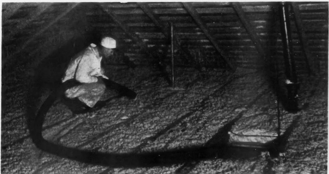
The Cost of Applying Insulation Is Reduced by Methods Like This where Mineral Wool Is Blown from the Ground Equipment, Through a Hose Into the Spaces Between the Attic Floor Joists.
