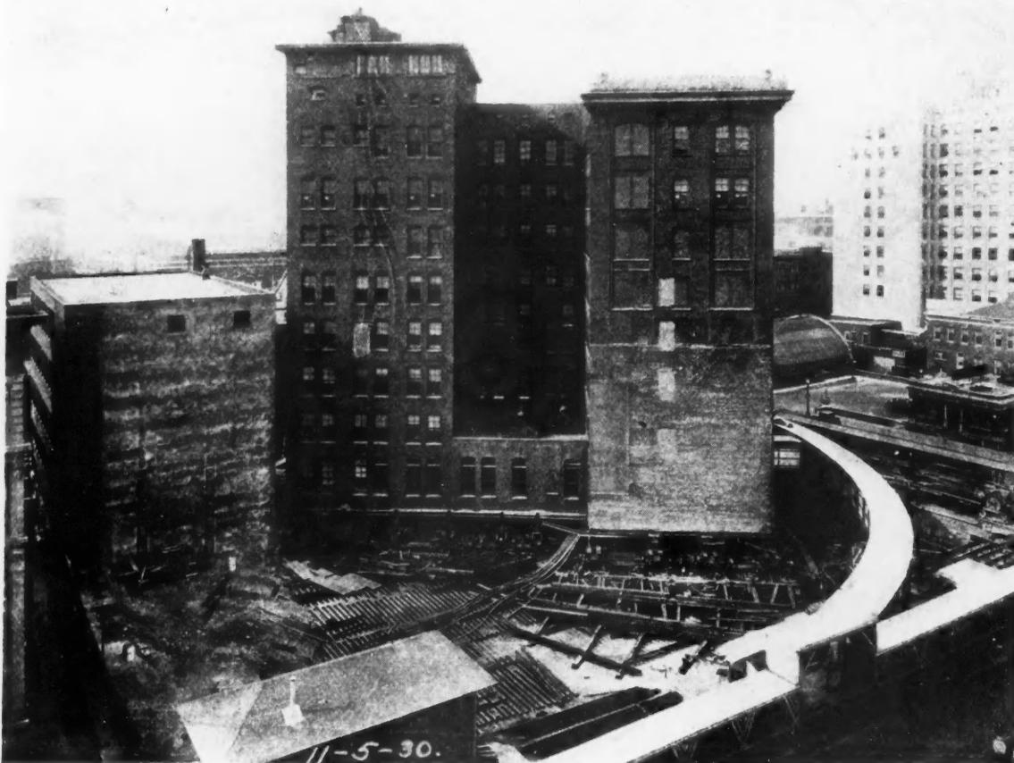
The Concrete, Steel and Timber Roadway for Moving.
