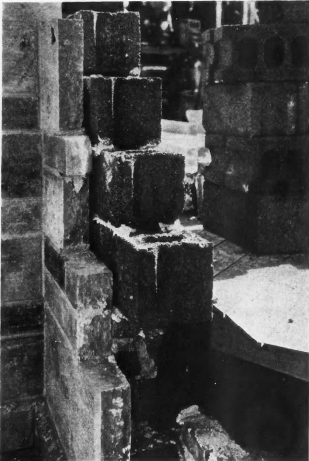
It Is Recommended That an Air Space at Least One Inch Be Provided Between Facing and Backing.
