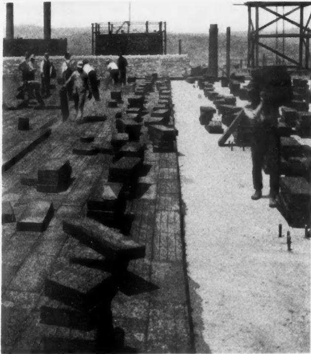
Blocks of Corkboard Used as Roof Insulation Are Easily Handled and Are Highly Effective.
