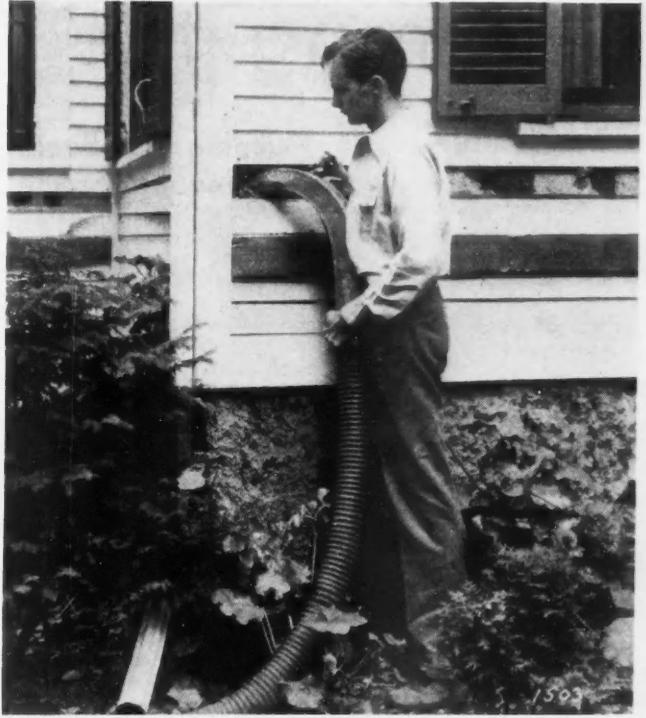
Rock Wool Can Be Blown Into the Walls of Even an Old House by Removing a Few Strips of Siding. An air compressor furnishes power.
