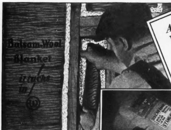
Easy to fit snug! Made extra wide for easy flanging between studding, joists or rafters. Scored on both sides for easy application. Flexible—calks every sized opening with amazing ease
