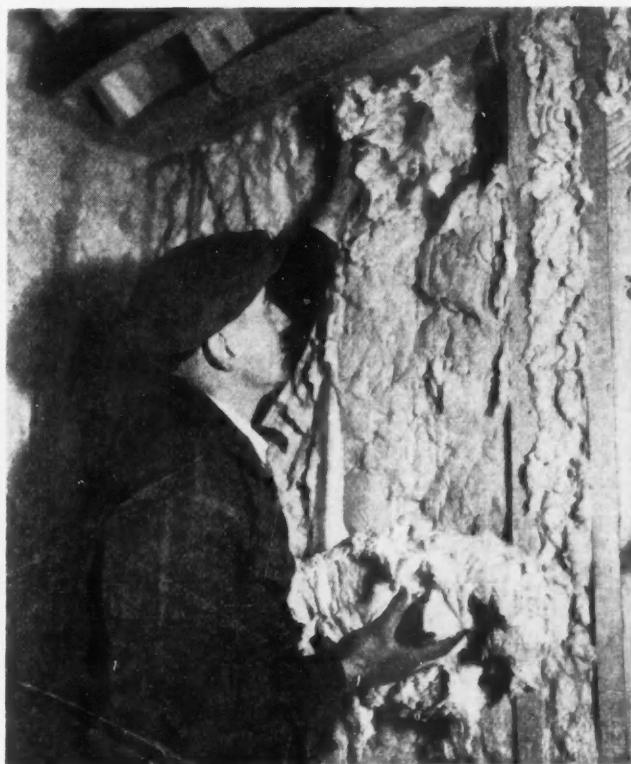
Mineral and Rock Wools Can Be Handled in This Way and Stuffed into Every Crack and Corner.
