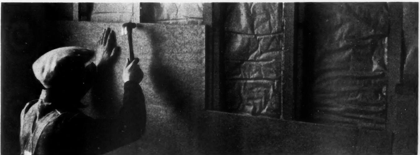
Here Is an Almost Ideal Insulation Job. The Air Space Between the Studs Is Divided by Means of a Flexible Blanket Material and a Fiber Board Is Applied to the Studs as a Plaster Base.
