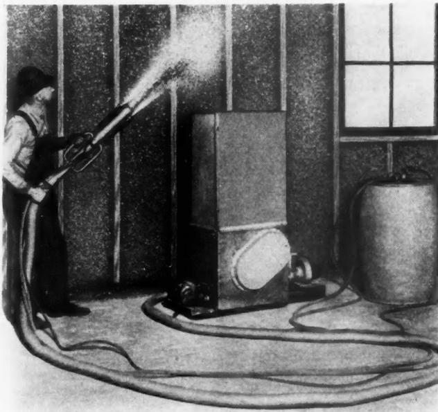
Insulation and Binding Material Blown Together Against a Wall to Which It Adheres Permanently.
