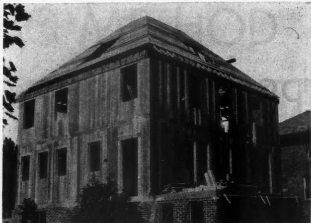
After the Gypsum Supported Concrete Slab Floor Is in Place, Vertical Units Form the Exterior Walls; Openings Are Left for Doors and Windows and Walls Are Complete Ready for the Exterior Veneering.
