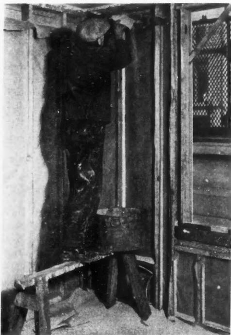
INSULATION WAS PLACED in the walls by the contractor's workman. A treated sawdust was used to provide both insulation and fire protection.
