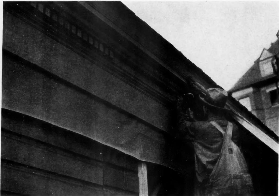
THE NEW DENTIL CORNICE SHOWN UNDER CONSTRUCTION ABOVE contributed greatly to the charm of the re-novized house in Portland. Compare the detail above with the old style treatment before rebuilding. (See illustration on page 28.) Willard Griffith was the contractor.
