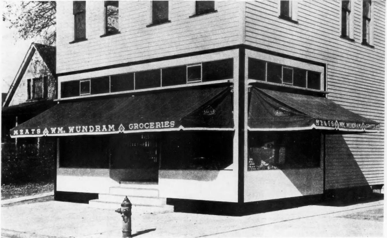
CONTRACTOR EMIL SCHRECK of Davenport, Ia., remodeled the old store below into the attractive, modern, revenue-producing store above. The building was cleaned up and painted, new concrete steps built, modern front of aluminum and Carrara glass installed. The cost was \$860.
