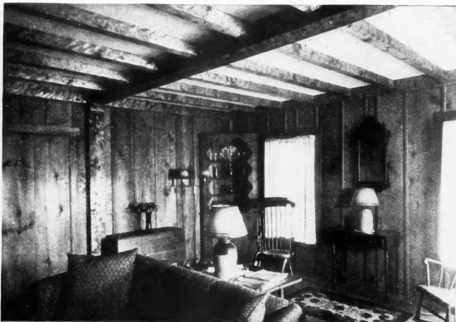
WALLS ARE COVERED with cedar shingles spaced 5" to the weather; asbestos shingles are used on roofs. Hand hewn pine timbers are used in the living room secured with hand made dowels. Side walls were sheathed with varying widths of  $\frac{7}{8}$ " pine and joints covered with  $\frac{1}{2}$ " strip moulding with a small bead on each edge for decoration.
