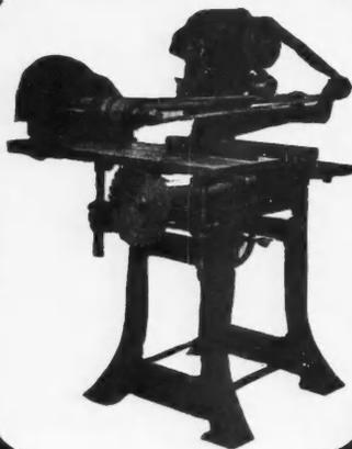
This remarkable machine cuts costs as quickly and as surely as it cuts wood! Does the work of five ordinary machines—eighteen different everyday jobs—faster and at less cost! Cross-cut saw, rip saw, jointer, shaper and router—five machines in one . . . at the cost of one. Ball-bearing throughout. Write for full particulars.
