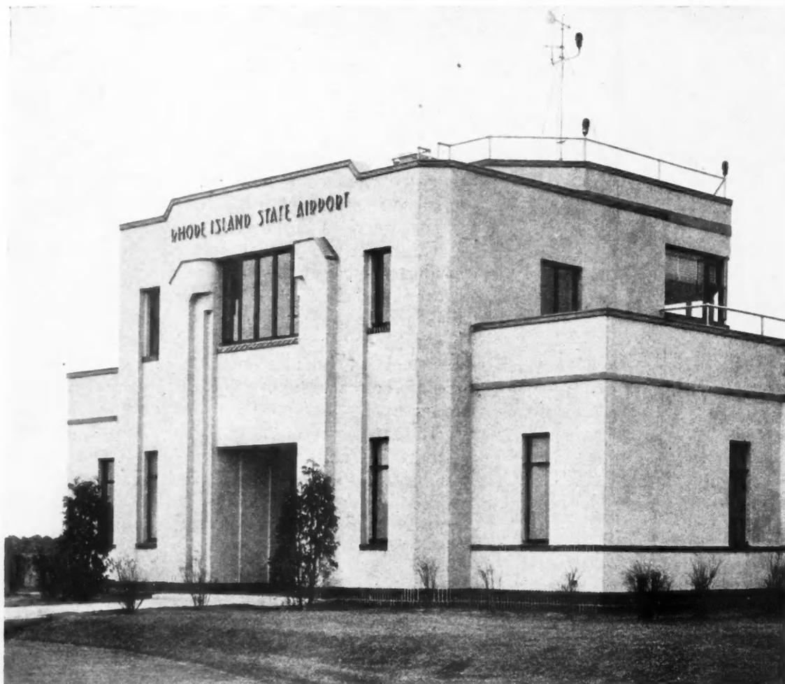
STANDING unprotected from the full sweep of storm, this airport building must face the worst kind of weather. Its stucco exterior must give protection from driving rain and sleet and snow, from bitter winds and constant freezing and thawing.
