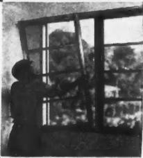
... drawing weights and baffle out of the way, inserts ordinary wood screws in prepared holes to complete the installation.
