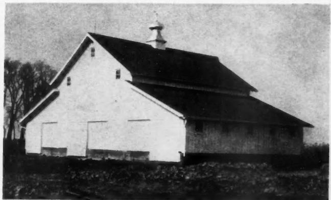
FIFTY YEAR OLD HAY BARN which was remodeled at cost of less than \$1300. The framing was in fairly good condition. New roof, side walls, concrete foundation and floor had to be placed.
