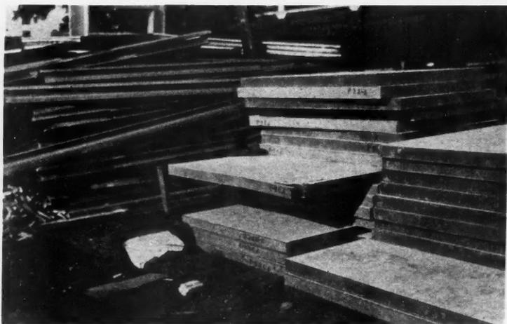
A PILE of Motohome wall panels delivered on job at Boston. Panels are made of four 1/2-inch thick sheets of cane fibre insulating board cemented together with 1/8-inch layers of cement asbestos on outside and inside of panel.
