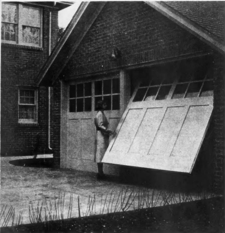
ABOVE: "A woman's touch" operates these Over-the-top doors supplied by the Frantz Mfg. Co. through the Eclipse Lumber Co. of Clinton, Iowa, for this modern garage built by the Hanson Construction Co. Each door is composed of 2 four-foot doors, angle-ironed together.
