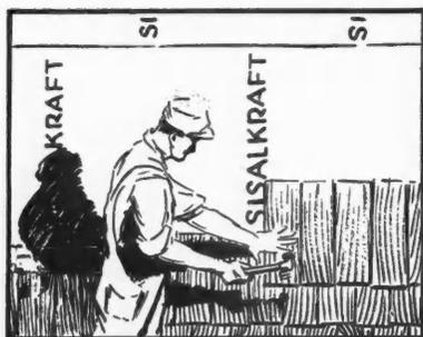
It has no equal when real protection is desired in frame wall construction. It guards against spotted or wet plaster. It wraps a house in a moisture and air proof blanket and makes it drier and more comfortable under all conditions.
