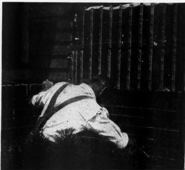
BELOW, mortar is being applied to brick slabs that have been locked in place on vertical furring strips.
