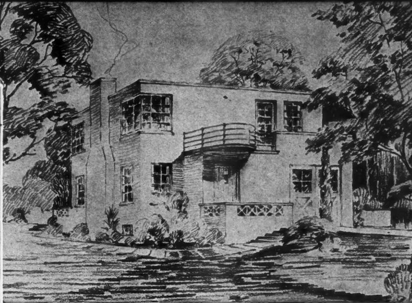
HOUSE No. 3 at Purdue is of poured concrete construction, sponsored by the Portland Cement Association; Burnham Brothers & Hammond, Inc., architects, Chicago. Basement excavation blasted through 2 1/2 feet of frost and work progressing under a canvas tent.
