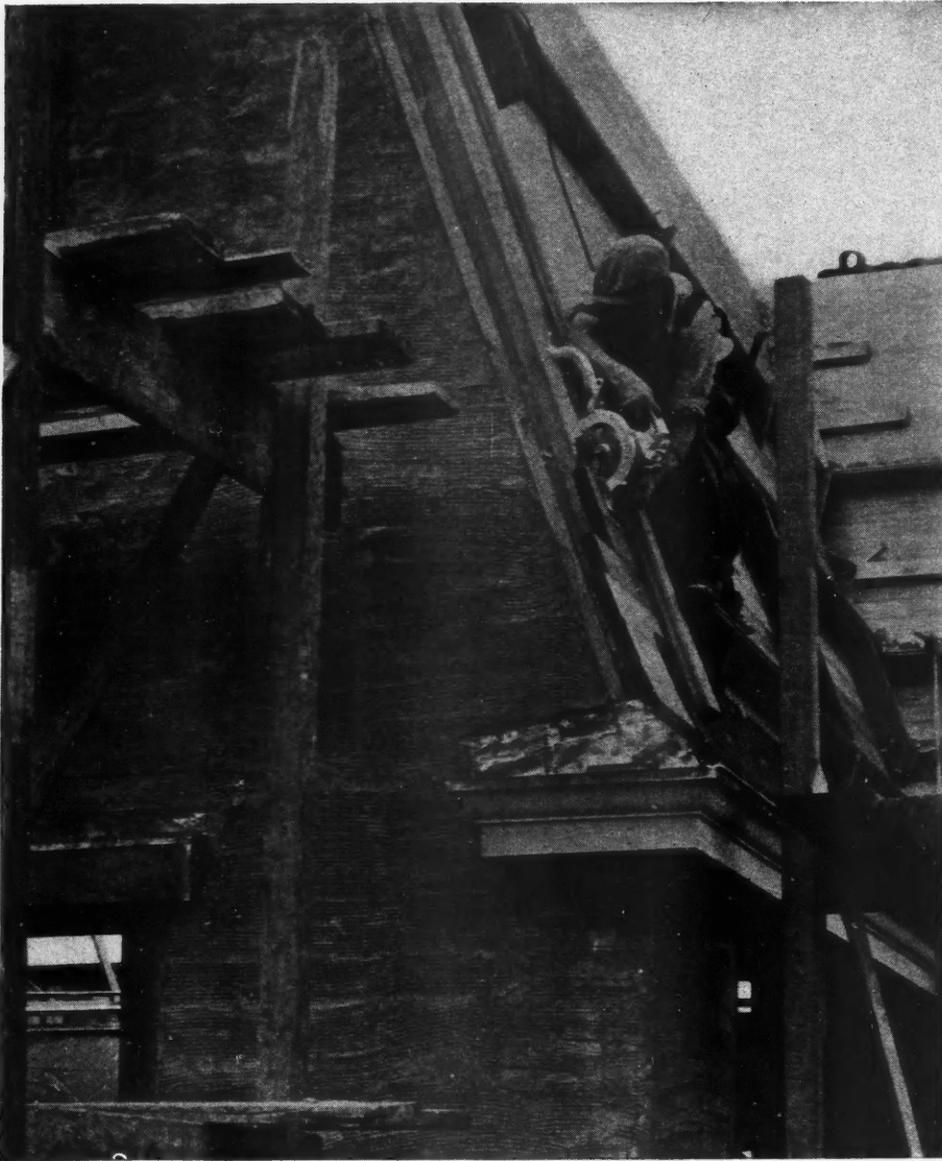
AN awkward cut that is being speedily handled at considerable saving with the electric saw.
