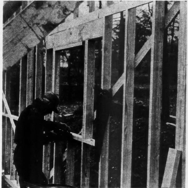
WORK under way on House No. 1 on the Purdue University Campus, the Housing Research Project. This house, by J. Andre Fouilhoux, architect, is of insulated wood construction with flat roof.
