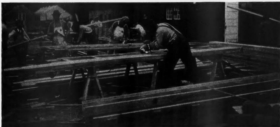
CONCRETE form building involving extensive heavy cutting is done much more cheaply with electric power.
