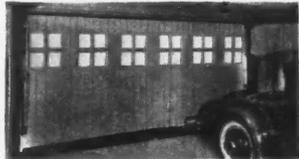
There's a size for every opening and only 3/4" head-room is required above standard openings. No excess trackage, no weights, pulleys, cables or chains.
