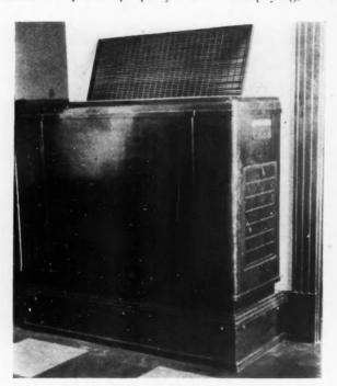
FIG. I. A wall unit of trim appearance and large capacity. Filter at top. Grille removed.
