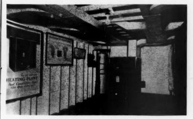
VIEW of the Reis model home basement, showing oil burning heating and conditioning system with duct installations and oil tank at right.
