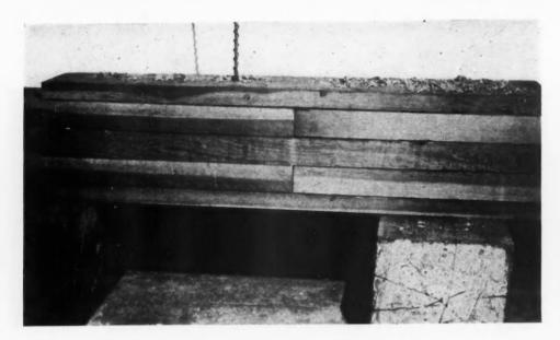
3-B. HOLES are then bored with a portable motorized drill, the full thickness of the splice assembly. Care should be taken to plumb the drill so that the hole will be perpendicular to the timber surfaces.
