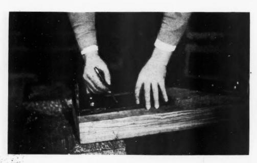
2-C. MARKING the holes for a column footing connection. The steel shapes with which the connection is made may be used as templates in spotting holes. Use of a drilling punch which fits the hole in the steel or template is preferable to marking with a pencil.
