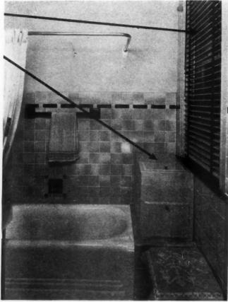
THE OLD two-tube high radiator behind door was replaced with seventube low radiator, and covered with radiator cover in the top of which was placed one-inch board of insulation. Now used in place of stool.
