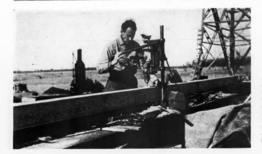
8-B. BORING timbers from shop details for a wood radio tower. Timbers for important structures are often laid out from shop details in the same way as structural steel, cut to length, drilled, and grooved ready for assembly in the finished structure. This may be done in the shop or at the site. Any millwork plant has the necessary equipment for such work.
