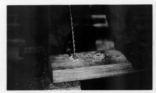
3-C. BORING 9/16" bolt holes at the points marked from the steel plate as a template. Holes should be bored from each face to meet at approximately the center of the timber.
