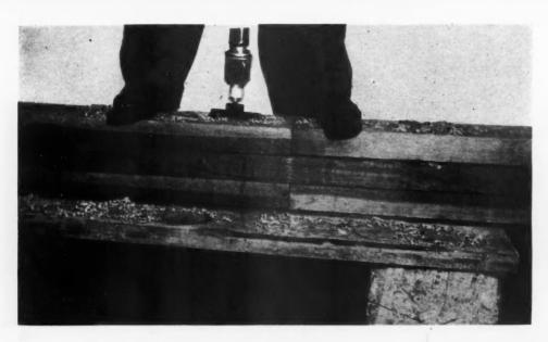
4-B. THE pieces forming the splice are then laid apart and grooved with a 4" grooving tool obtainable from the Timber Engineering Company. This also can readily be driven with a portable motorized drill. The pilot of the grooving tool fits in the bolt hole, centering the groove about the hole.
