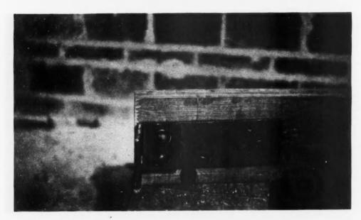
7-C. BOLTING on the steel fittings. Note wide washers used to give the half-inch bolt head adequate bearing over the 15/16" hole in the steel. Note also the end of the boss or hub of the shear plate showing in the 15/16" hole at left.
