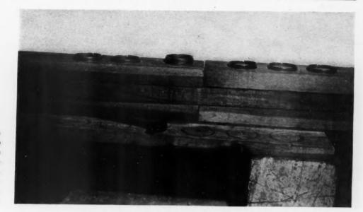
5-B. SPLIT rings being placed in the outer chord members. Outside splice plate shows below grooved to fit on the rings as shown above. Note the split or break in the ring perimeter. The grooving tool is purposely made to cut a groove slightly larger than the diameter of the ring when closed.
