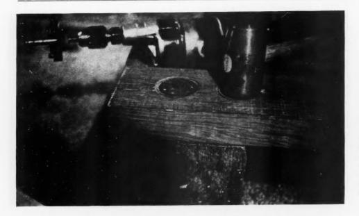
6-C. THIS shows one shear plate already imbedded and one in process of driving. Note the tip of the striking sledge on top of the recessed sledge. Grooving tool and motorized drill appear in the background. Pilot of the grooving tool showing at extreme left is inserted in the bolt hole to center the dap accurately.
