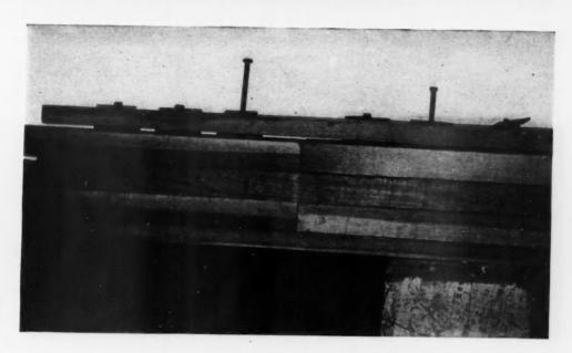
6-B. SPLICE pieces reassembled and bolts are being inserted to hold the members together in the structure.
