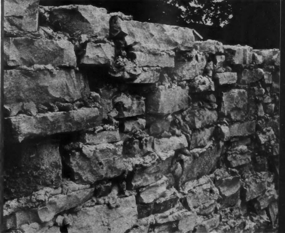
**INSIDE LINING WALL**—This photo of "Ageless Art" Double Wall Construction tells a big story. Against the inside of the outer wall is a blanket of waterproof sprayed-on insulation averaging  $\frac{1}{2}$ " to  $\frac{3}{4}$ " in thickness. The inner wall, which consists of a 3" light weight cinder or gypsum block, covers the irregularities of the stone wall and provides a plaster base.
