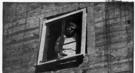
Building paper applied. Fenestra Casement lifted through the opening and installed from inside.
