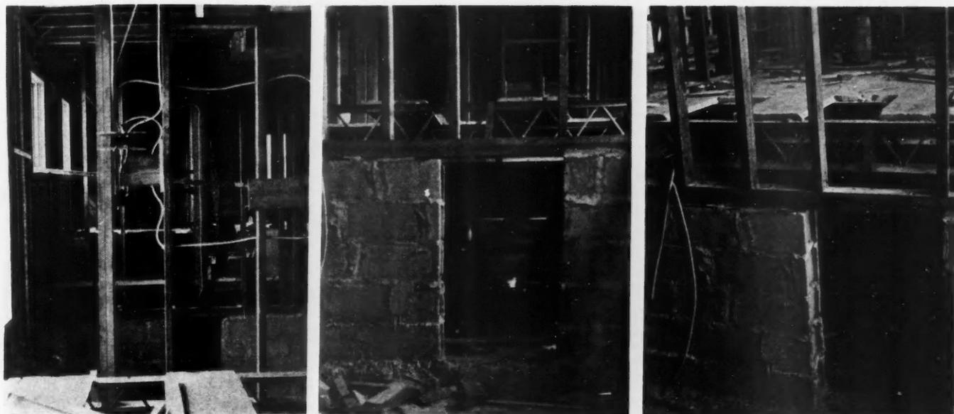
**THREE VIEWS** of heater room and floor construction. At left: looking across from first floor level. Middle: view from floor of heater room looking under house. Right: detail of floor construction.
