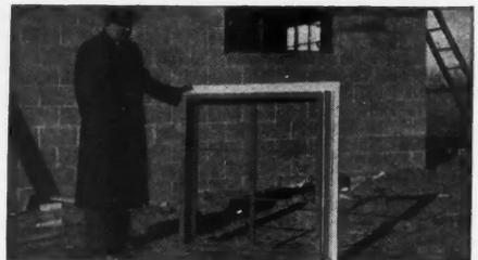
Fenestra Casement and Casing with outside wood trim in place ready for installation.
