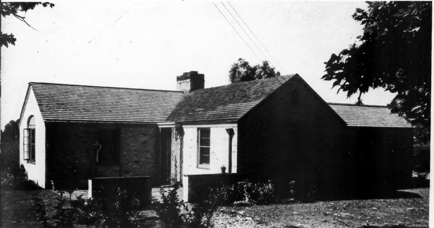
THE SIMPLE details of this entrance give life to an otherwise bare corner. Walls are of second-hand brick, painted with oil paint. Roof is of red cedar shingles. Outside trim is painted cream color.
