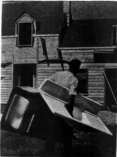
LIGHTER weight, a means to lower cost—plumber on Fred J. Walsh project at Markham, Ill., carries in a full-size bathtub and kitchen sink of new formed metal.
