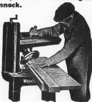
Cutting jack-rafters with No. 1 Radial Saw. Machine also rips, cross-cuts, dados, copes, routs, etc. A versatile and accurate tool.
