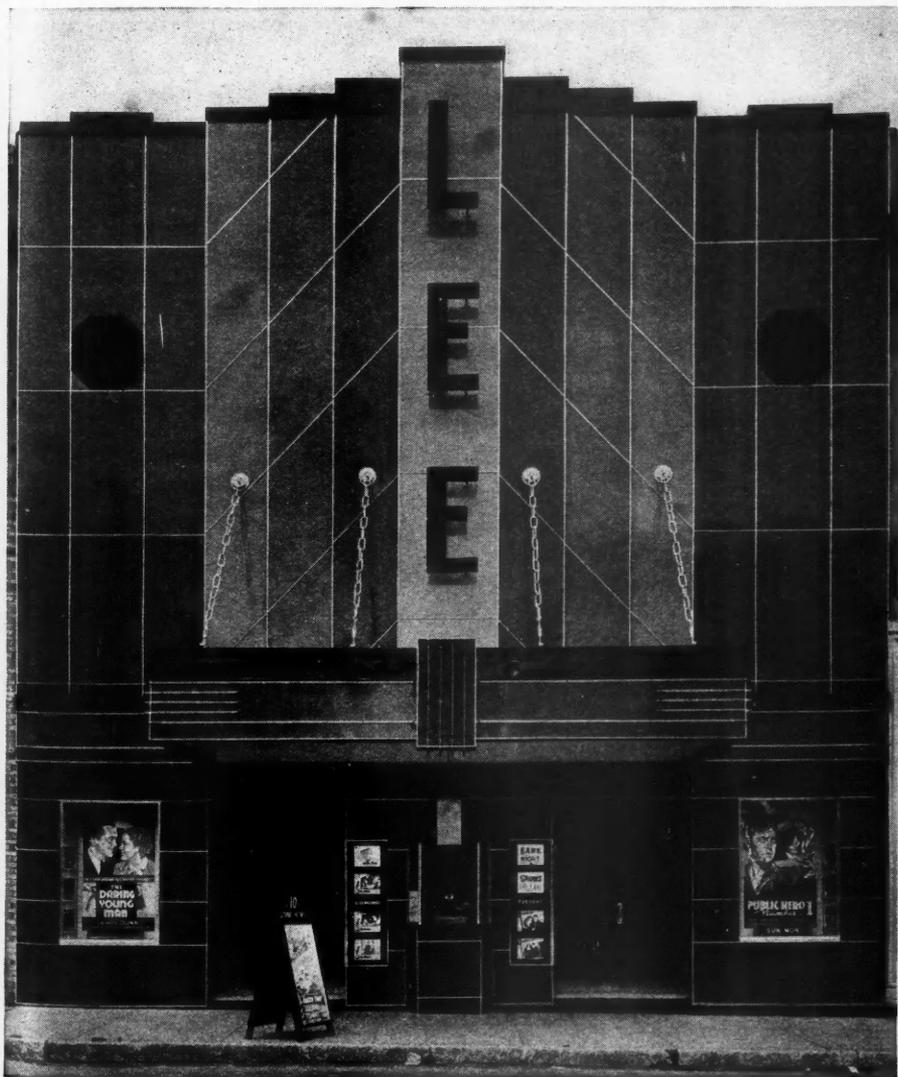
AFTER a treatment of broad, colorful surfaces, brightly lighted at night, the structure has been given new business character at reasonable cost. The drawings above illustrate details of applying the pressed-wood panels as used on this and similar types of commercial buildings.
