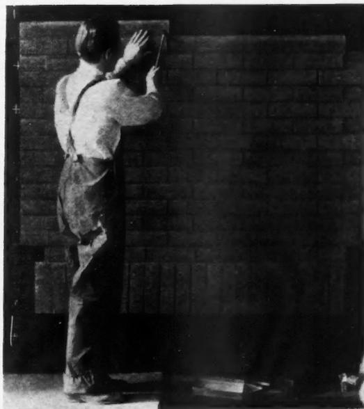
APPLYING 3-in-one brick type siding made of Portland cement reinforced with asbestos fibres.
