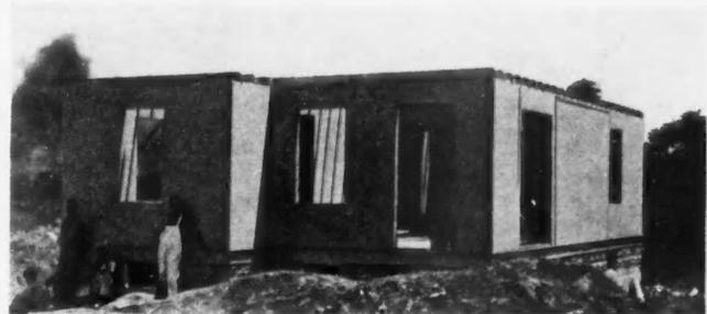
SHOWING ERECTION of a small home by precision-built methods, using Homasote board in sheets up to 8 x 14 feet.
