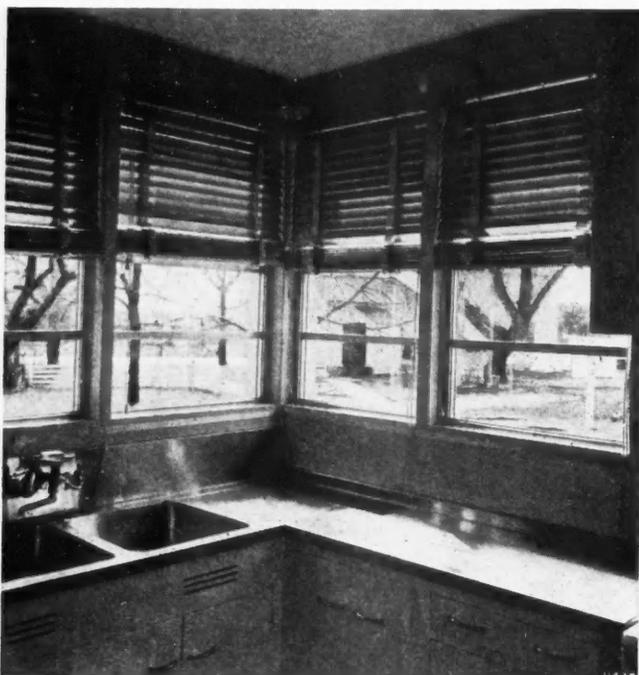
found on the famous Zepher, and other streamlined trains, and the new "silent" surface cars operated by the Chicago Street Railway Company. It was reasoned that a window sturdy enough to withstand the constant vibration of railway rolling stock should deliver new and higher standards of satisfactory operation in houses, and so the recently perfected unit was introduced to the building industry.
