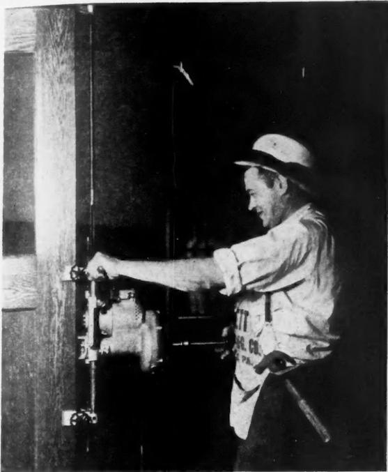
**SLOW AND EXPENSIVE** hand mortising of doors is being replaced by the electric mortising machines. With the mortiser above, 45 perfect mortises can be cut per hour—a tremendous reduction in the time and cost of this operation.
