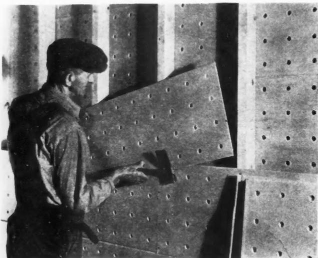
**PERFORATED Rocklath partitions, plastered in the approved manner with gypsum plaster have a one-hour fire rating.**
