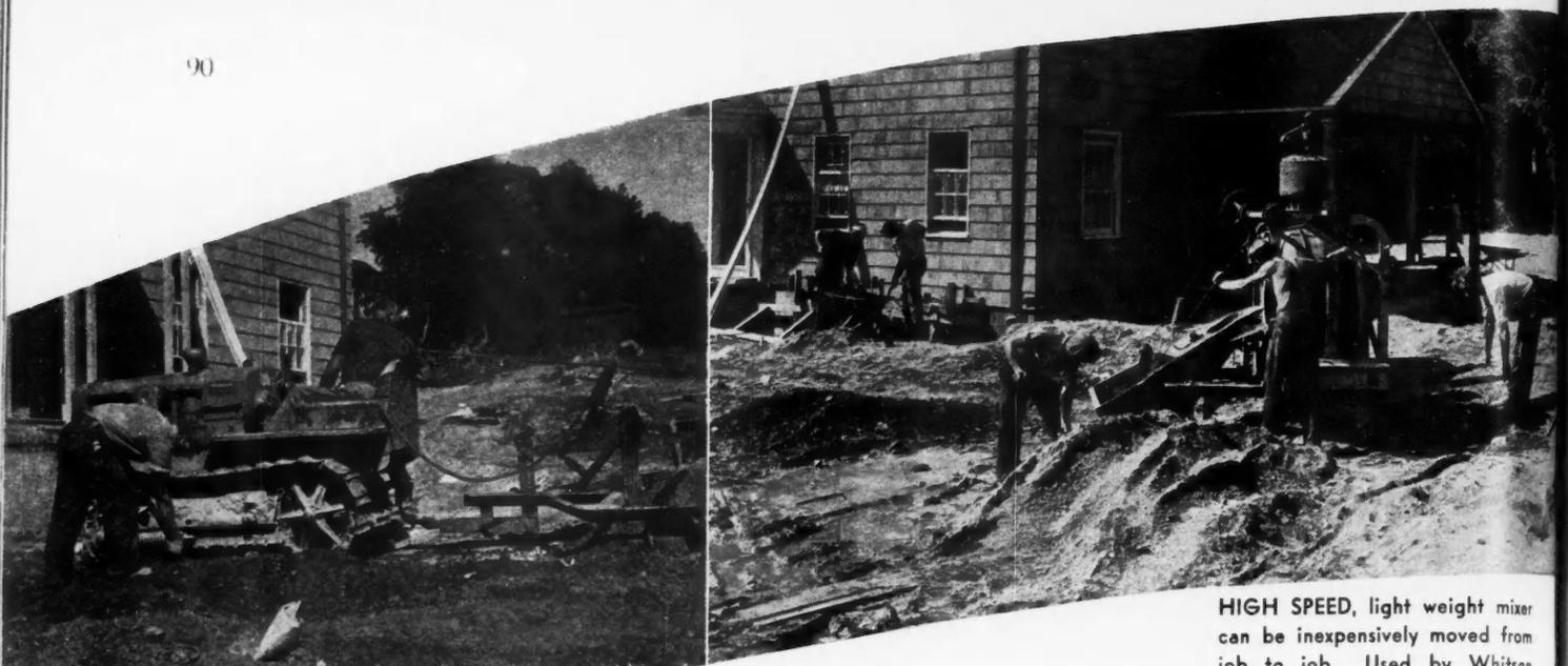
CATERPILLAR tractor with rotary scoop reduces excavation, grading and back-filling costs.
