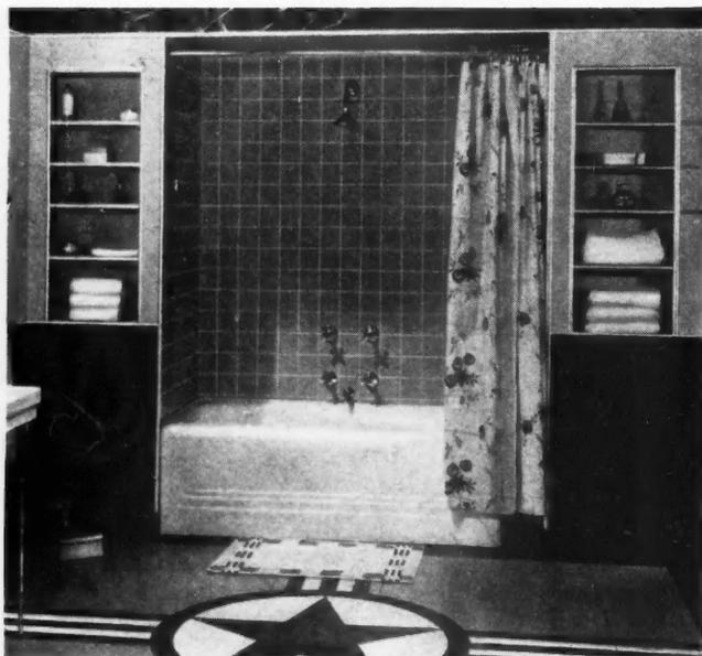
**LACK OF LARGE-UNIT TILING** a decade ago ran up the cost of vitreous walls. Decorative wall boards were developed in an effort to reduce the cost of covering kitchen and bathroom walls. In 1929, Johns-Manville manufactured and sold a decorative board consisting of a sheet of flat transite covered with a lacquered finish. It was fireproof, easy to clean, and attractive in appearance. The finish, however, was not as durable as the 1937 product.
