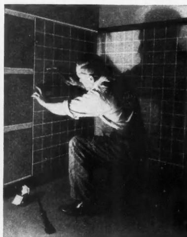
Cupped head finishing nails are furnished which can be readily driven through the panel. No drilling of nail holes is necessary.
