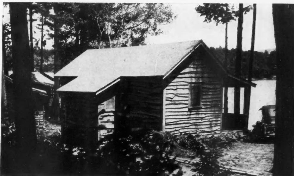
THESE are the Lamb Bros. single-unit cabins, the main part of which is 12' square. There is a 6' porch and a 4' x 4' toilet addition at rear. This addition is sometimes placed on the side but is a little more difficult and expensive to build. The rough-sawn pine board exteriors can be left in their natural color or given a coat of light brown or green stain.
