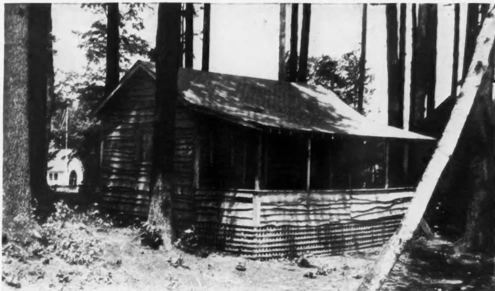
REAR VIEW of the double-unit Lamb cabin overlooking Lake George, N. Y., showing the double toilet room projection at rear. Dimensions of the cabin are 12' x 24', to which is added a 6' front porch, full length, and a small toilet room projection at rear which is 4' x 8'. Putting the 2 units together in this fashion reduces the plumbing costs.
