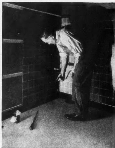
Curves and large holes can be cut with a coping or jig saw and holes up to one inch can be drilled with a brace and bit.
