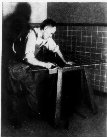
Where desired, the edge of the sheet can be beveled with a draw knife or block plane as illustrated in the photograph above.
