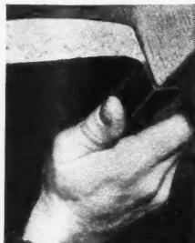
● The new Balsam-Wool Spacer Flange that increases Balsam-Wool efficiency and reduces costs. The flange is fastened to the face of stud, rafter or joist with staple hammers—no lath required.
